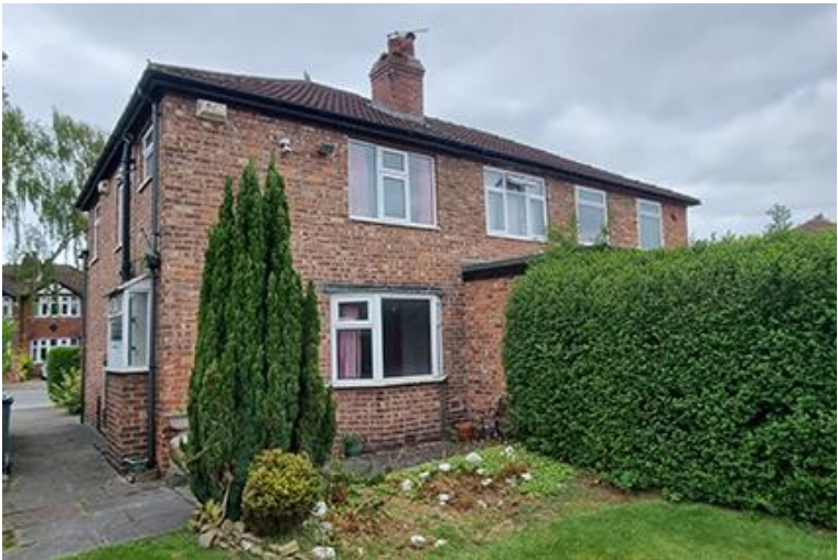
Photo of existing rear elevation
