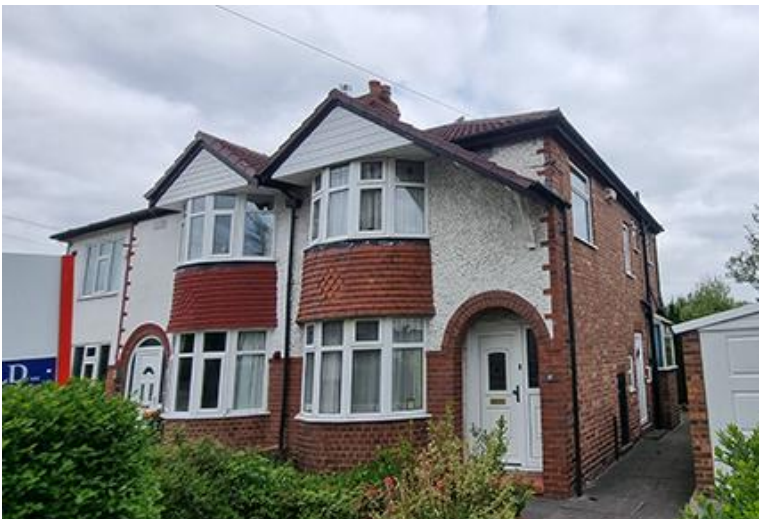
Photo of existing front elevation
