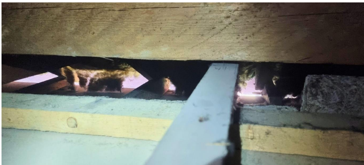
Plate 15: An internal view of the soffits in Graham.
