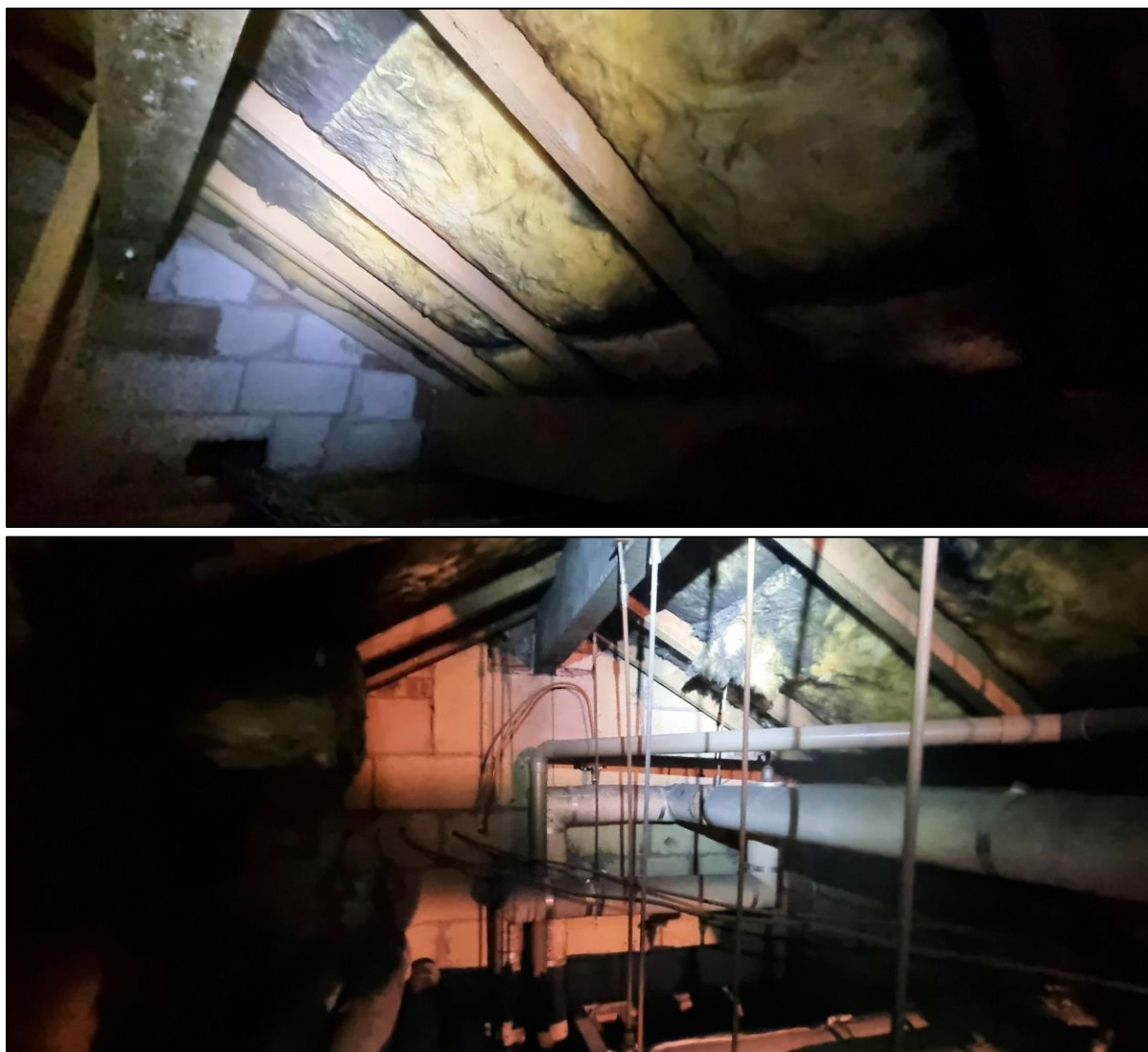
Plate 13: The roof voids were subdivided into separate spaces that were open to the roofing timbers and insulation.
