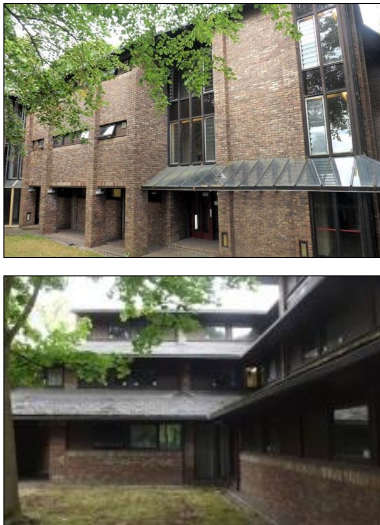
Plate 1: General views of Ewing and Graham Hall
