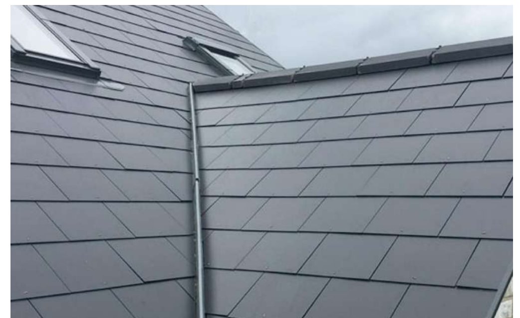
Fibre Cement Roof Tiles to houses
