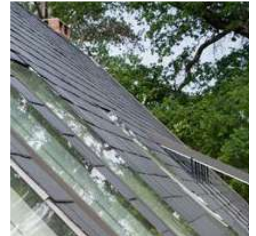
Roof Lights- Flush roof lights
