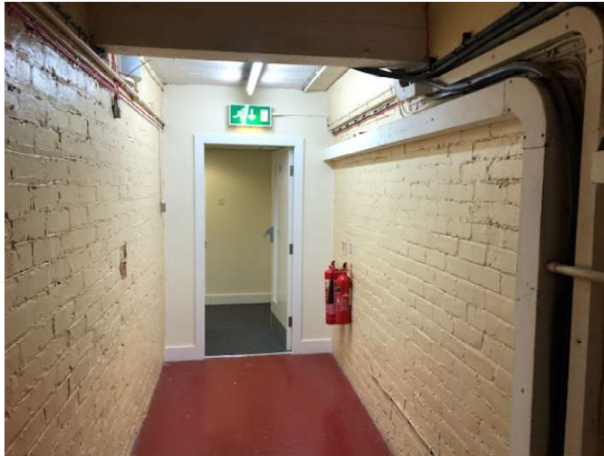
1. View of fire door / wall to be removed. Trunking to be boxed in.
