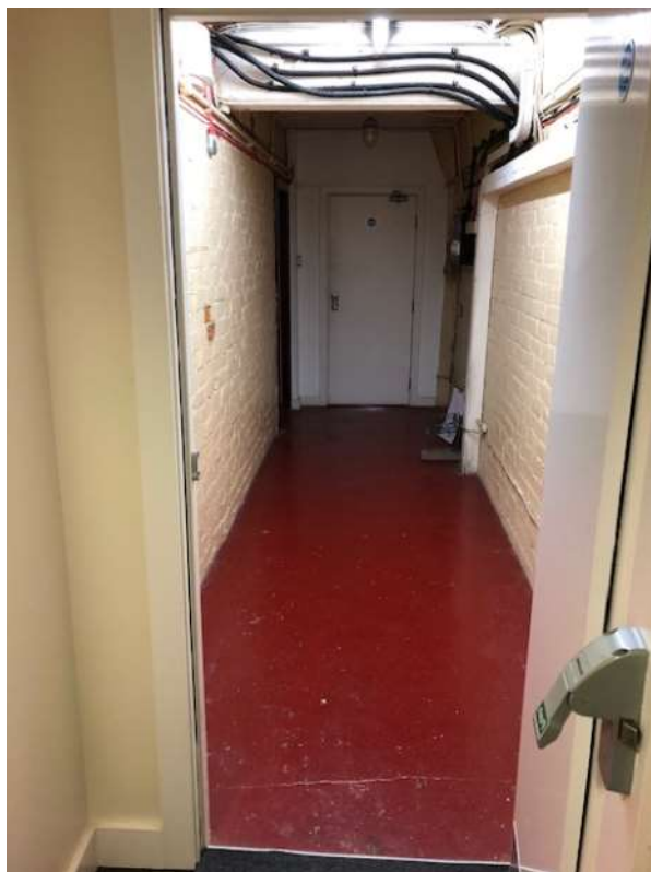
2. Opposite view of fire door to be removed.
