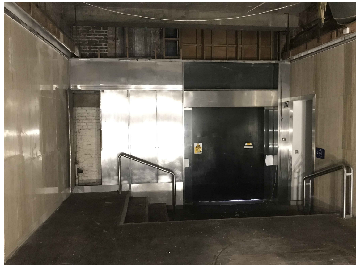
07 EXISTING ENTRANCE LOBBY 500 NTS INTERNAL PHOTO
