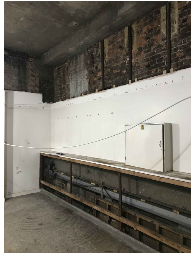
05 FIRST FLOOR DOOR HOUSING 500 NTS INTERNAL PHOTO
