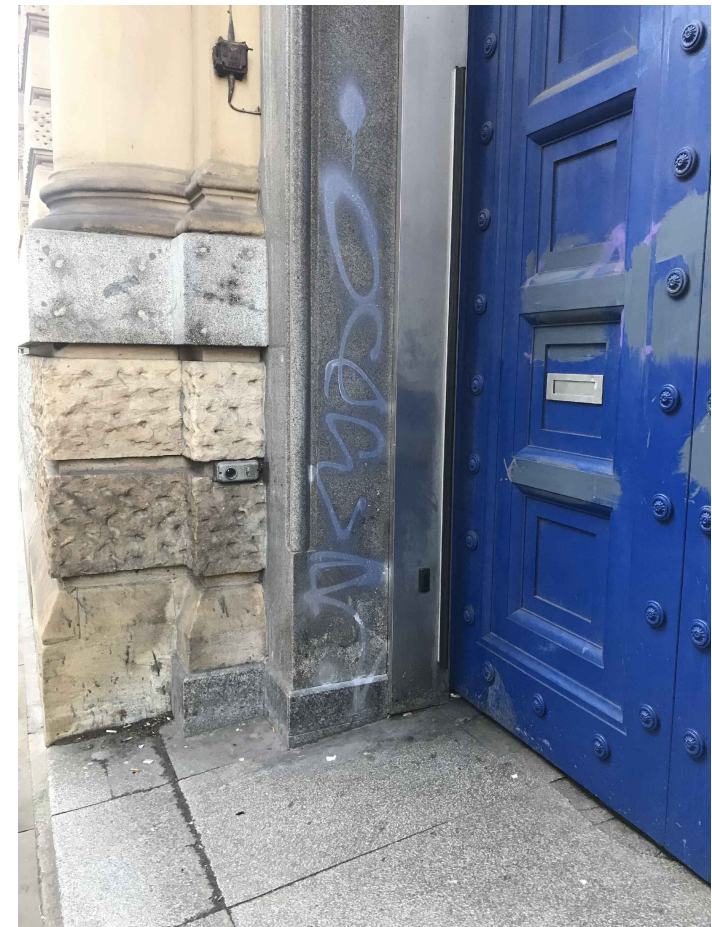
08 EXISTING MAIN DOOR 500 NTS EXTERNAL PHOTO
