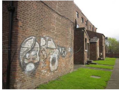
4 Exposed rear of the properties
