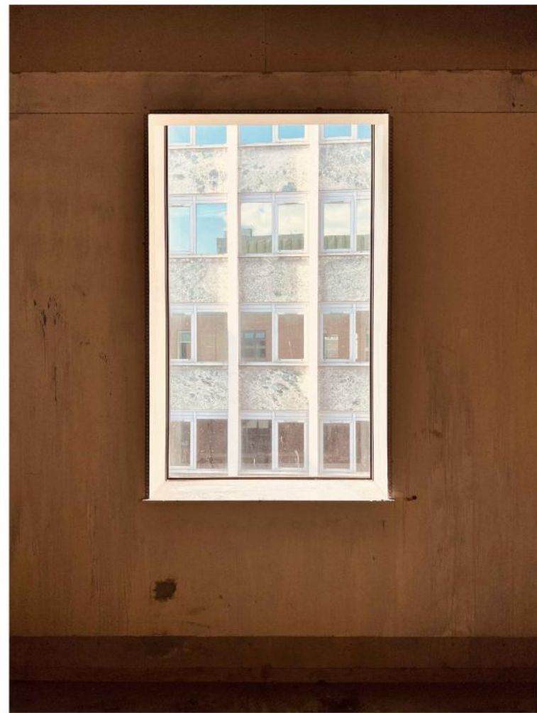
03 SECOND FLOOR EXISTING WINDOW PHOTO SCALE - N/A PHOTOGRAPH
