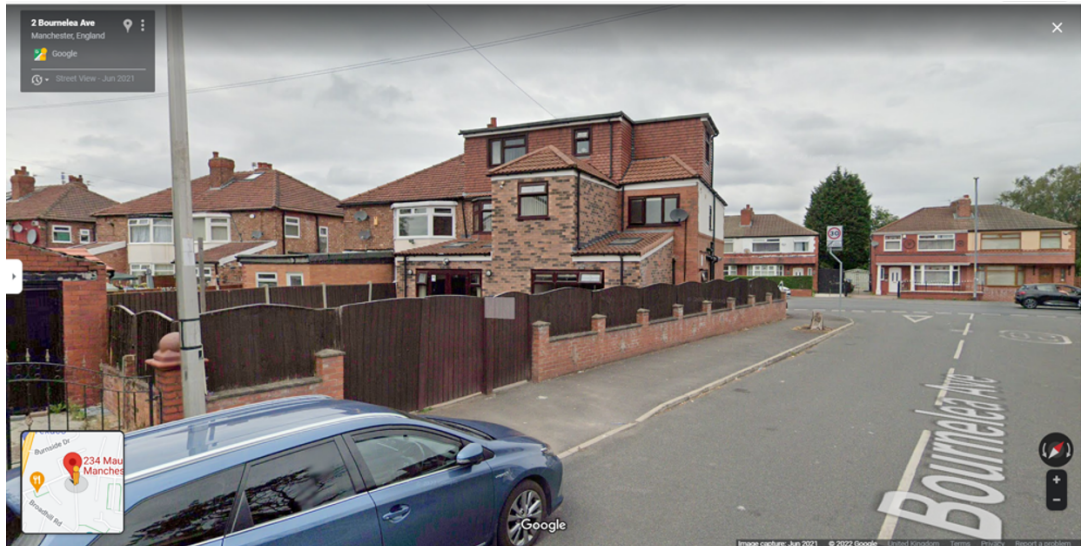
Figure 2: Showing dormer allowed on appeal at 234 Mauldeth Road.
