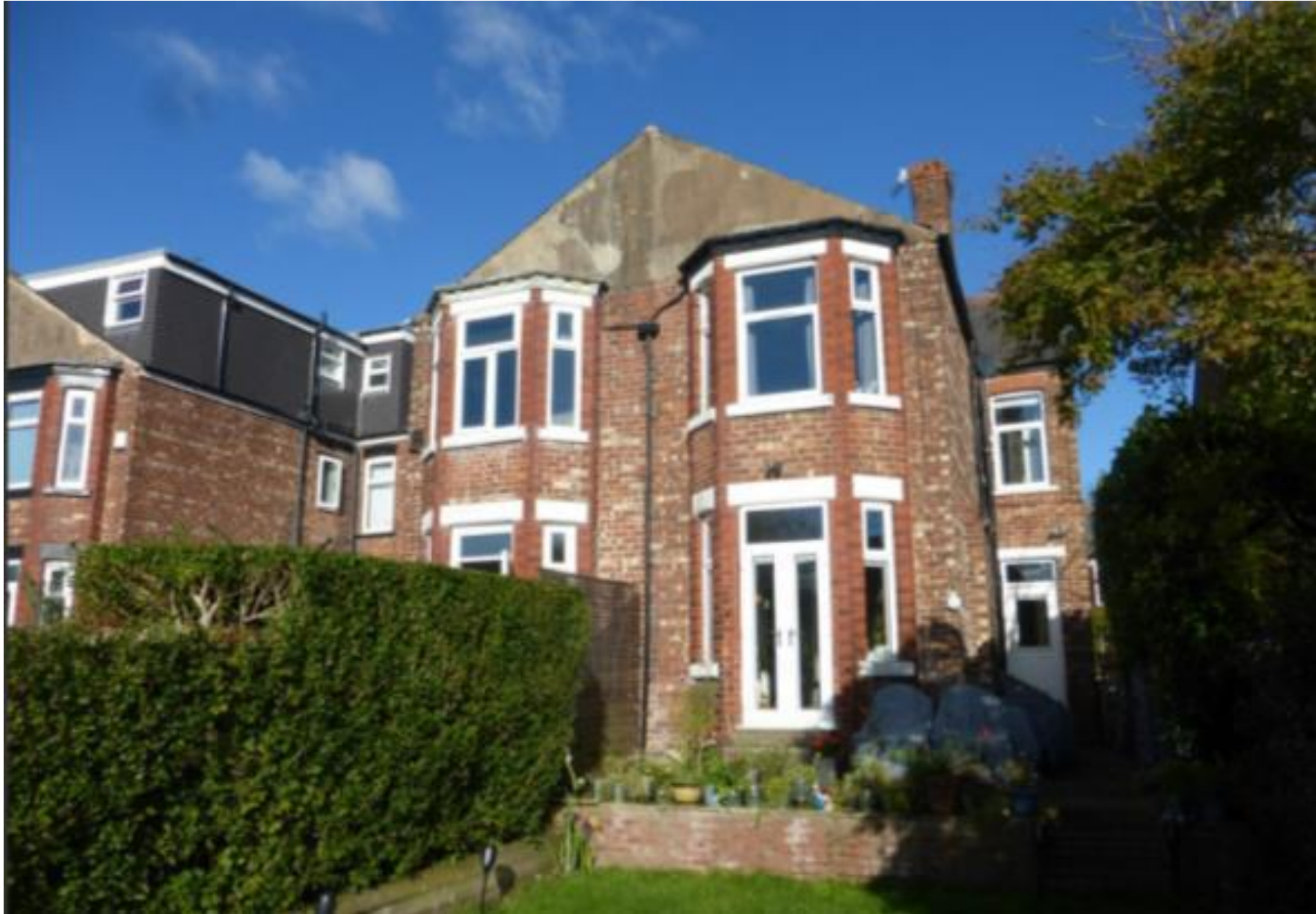
Photo showing rear of 16 and the existing rear dormer of 12 Clarendon Road (on the left).
