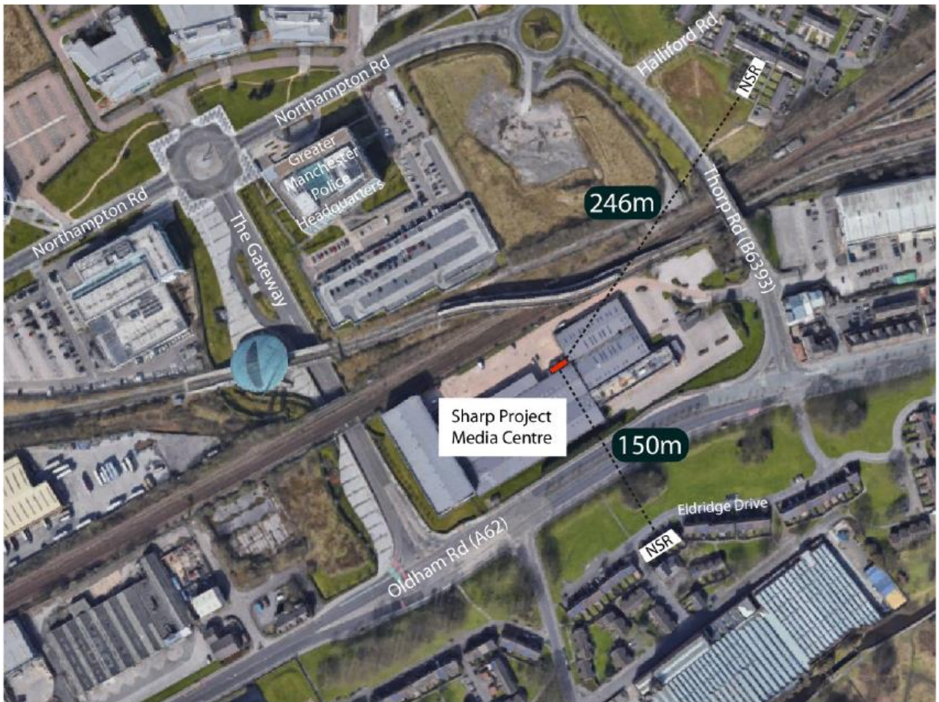
Figure 1: Location of installed plant equipment highlighted in red and closest NSR properties highlighted in white
