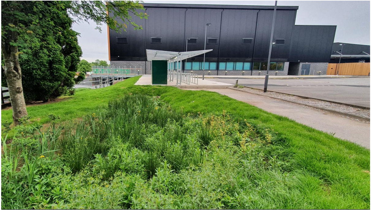
Rain garden swale general image
