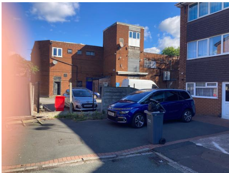
View of rear
