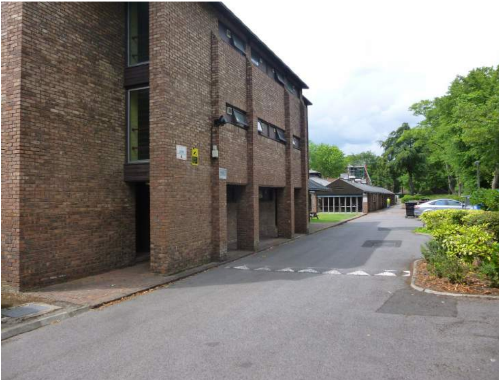
Looking north towards Dining Hall,
