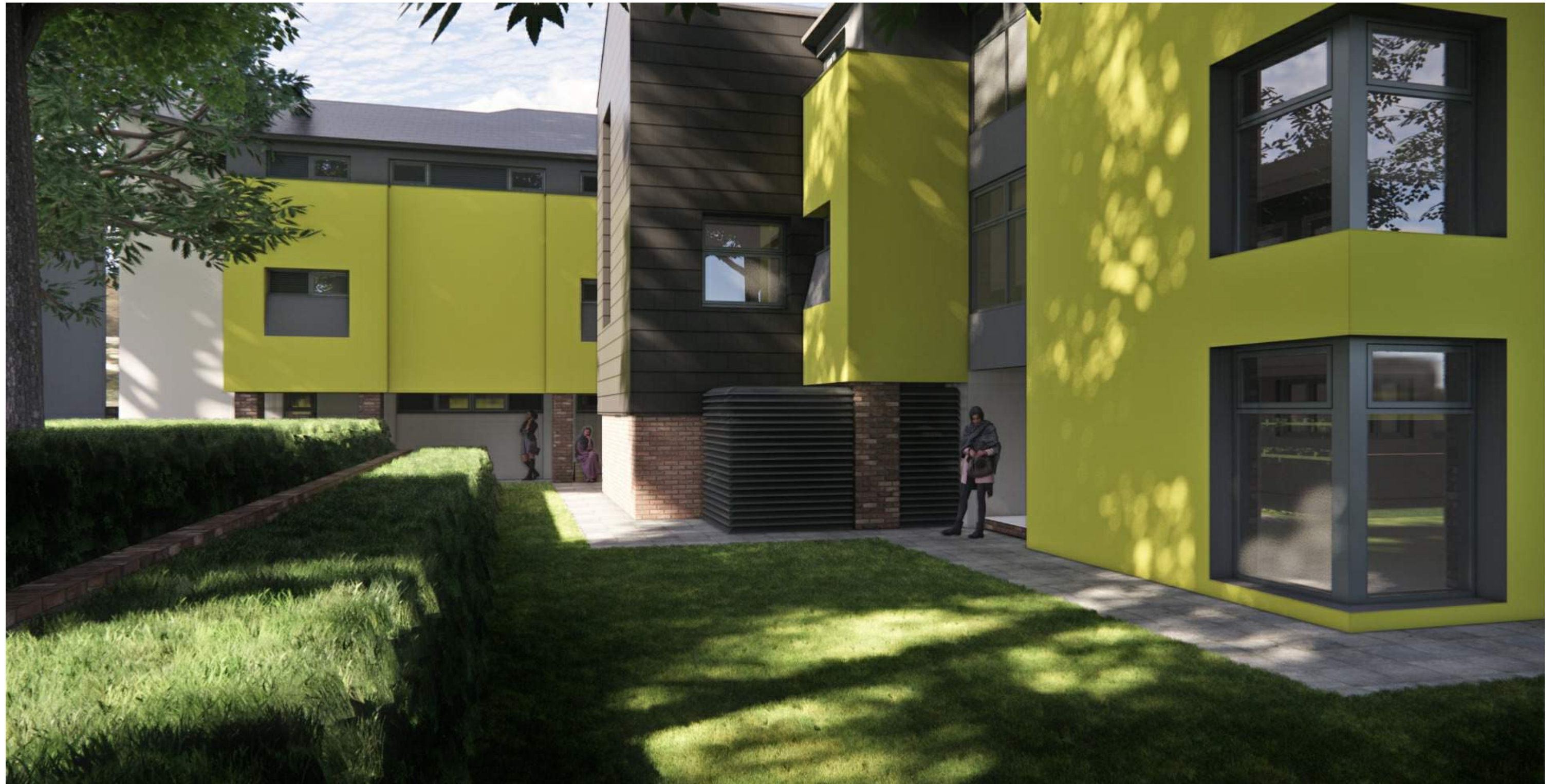
Graham Building - looking west from Anson Road frontage
