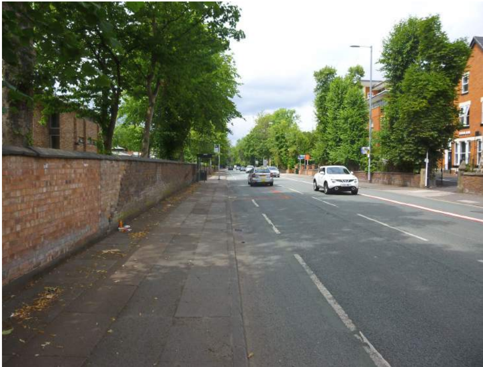
Looking north along Anson Road, with Ewings Building on left
