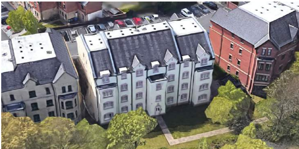
Hadfield Close /Conyngham Road (unlisted)
