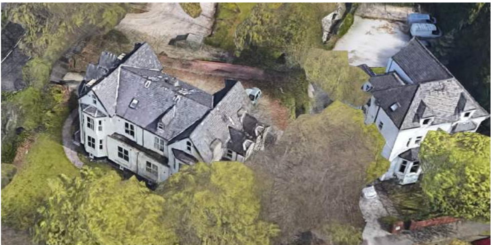
23 Denison Road /9 Conyngham Road (unlisted)
