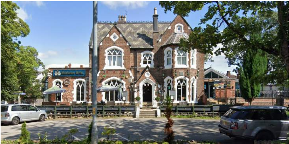
Milverton Hotel (formerly Rampant Lion Hotel), Anson Road
