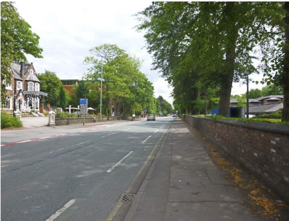
Looking south along Anson Road, with Dining Hall on right + Ewings Building beyond
