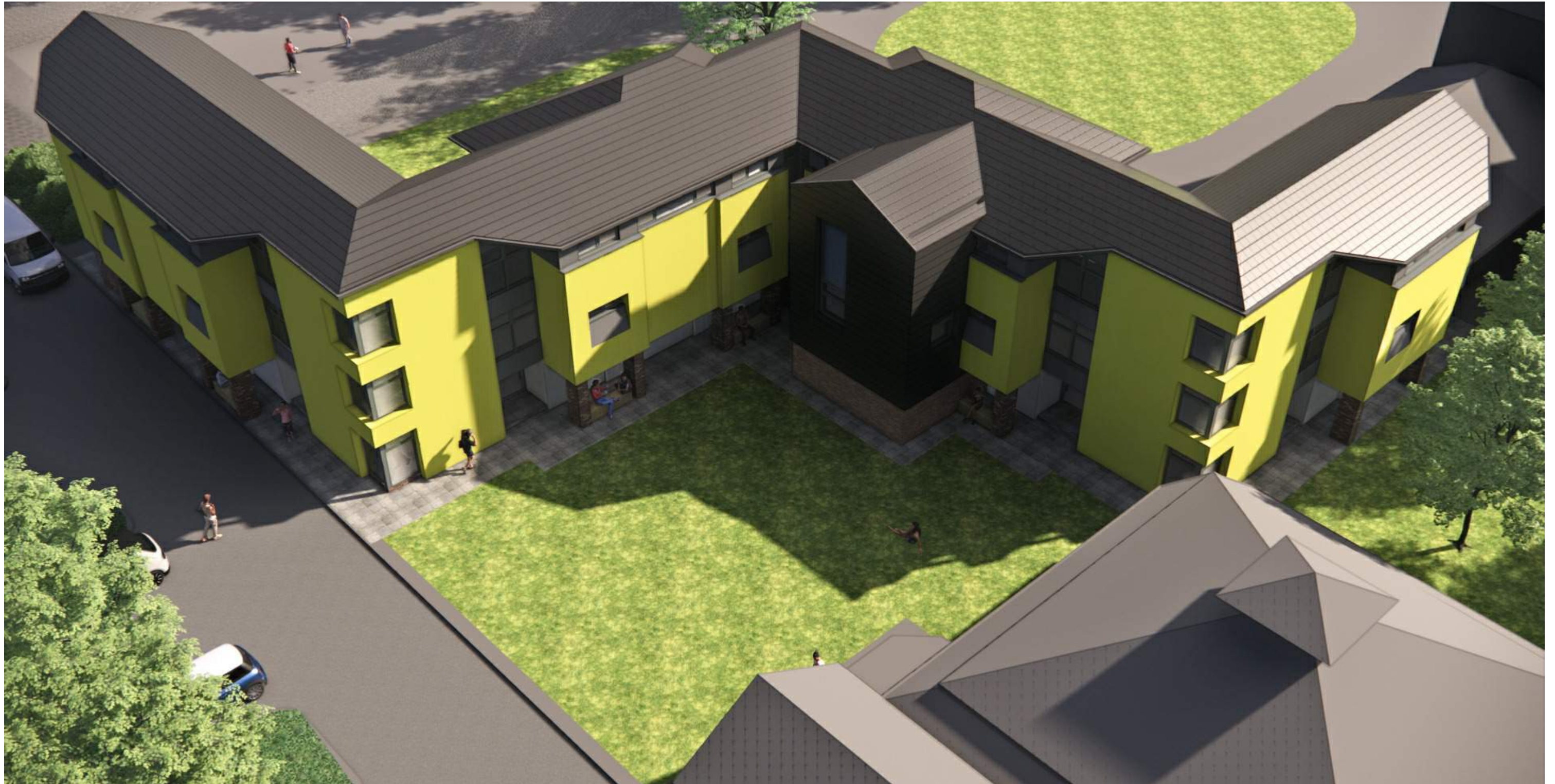
Ewings Building – aerial view looking south
