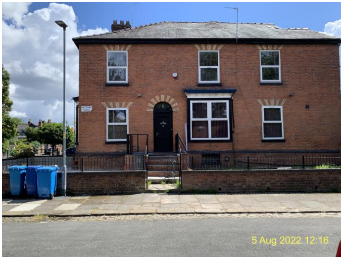
Photograph 1: Mitford Road Frontage
