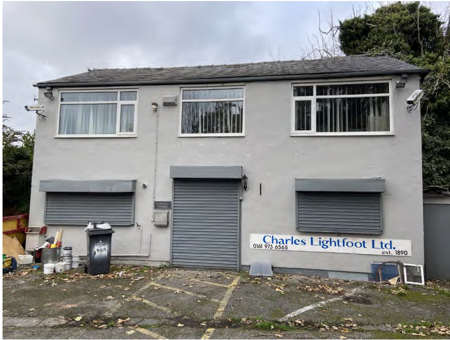
Existing building to be demolished
