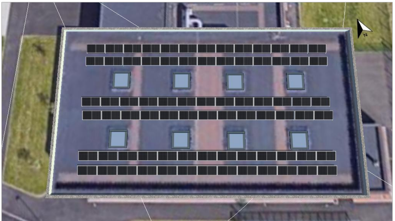
Figure: 1. Module Area - Building 01-Roof Area Southwest
