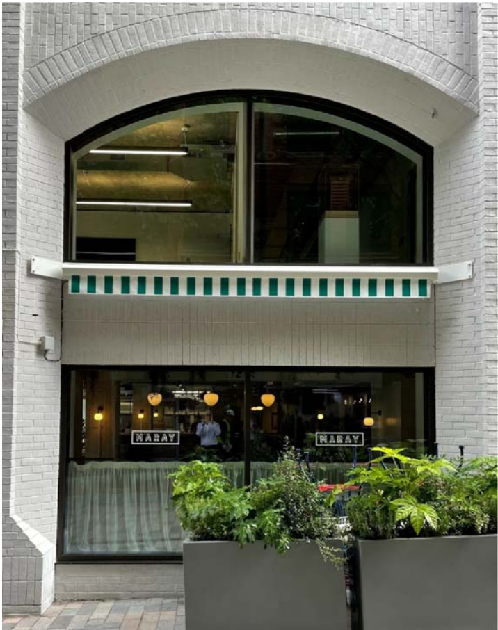
Image of Installed Canopy NTS @ A3
