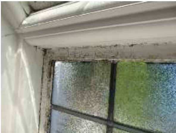
Single glazed window and timber window frame
