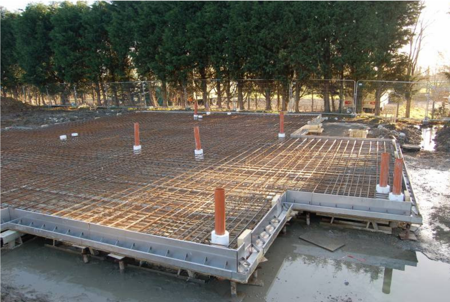
The slab prior to the concrete pour. The reinforcement steel, service ducts rising up through the slabs and the stainless steel edge detail can all be seen. The edge is levelled to a high tolerance by means of perimeter jacks.
