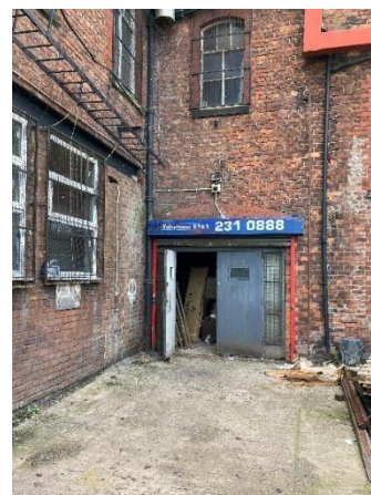
Figure 2.7 View of existing entrance to the building
