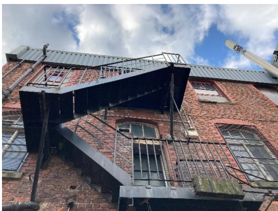
Figure 2.6 View of external stairwell on side east elevation
