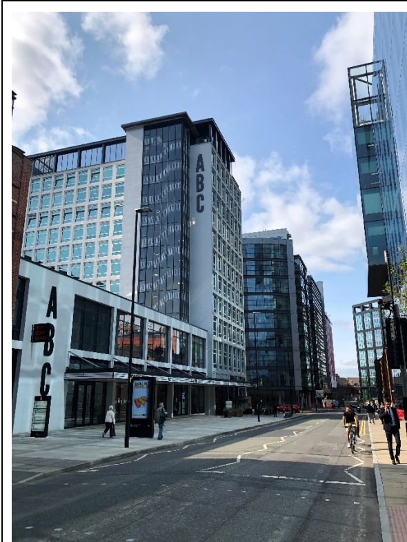
Figure 14: Looking west along Quay Street from its junction with Byrom Street and the Site, illustrating the entirely modern streetscape from this location, including a number of medium-rise office buildings from the 1960s, 2000s and 2020s.
