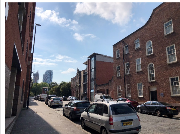
Figure 15: Looking south into Byrom Street from outside the side return of No. 17, illustrating the smaller scale and height of buildings leading into St John Street Conservation Area.
