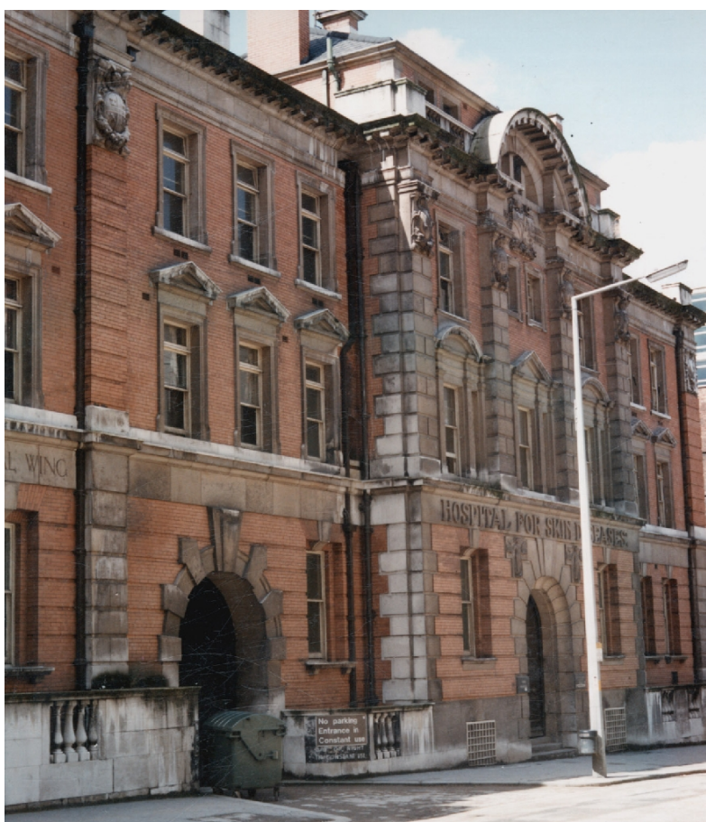
Figure 8: A view of the Quay Street elevation of the hospital as seen in 1988. (Source: Manchester Archives)
