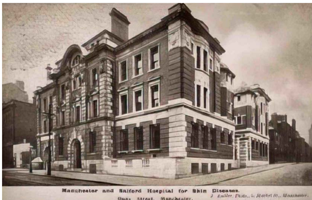
Figure 5 – A view of the newly completed Hospital for Skin Diseases as seen in the early 1900s. Note the vacant plot to the left of the building on Quay Street. (Source: historic postcard)
