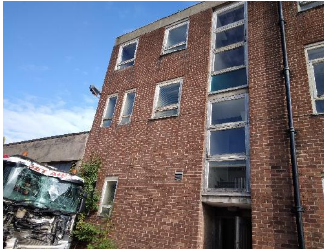
Southwest elevation of office block
