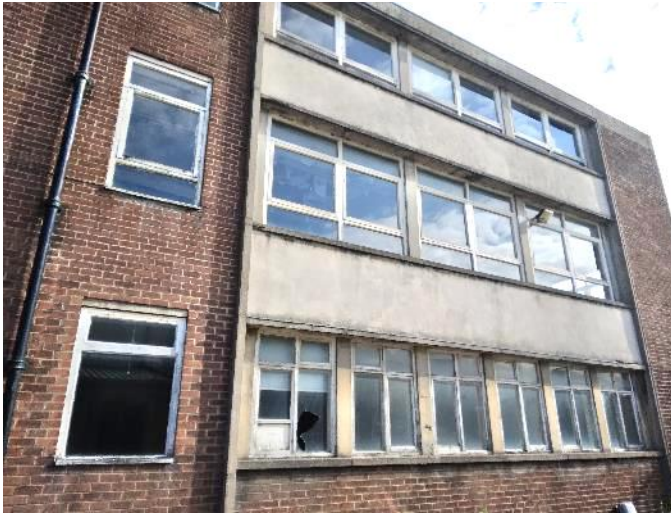
Southeast elevation of office block
