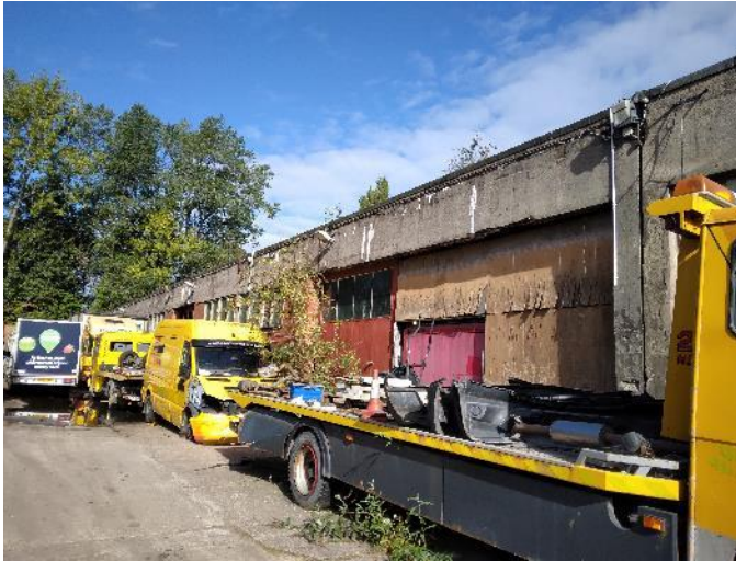
Southwest elevation of garages
