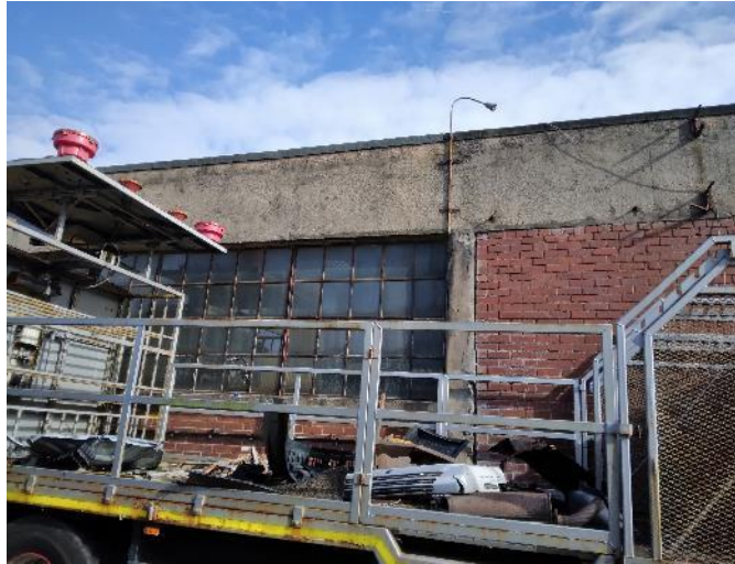
Southwest elevation of garages
