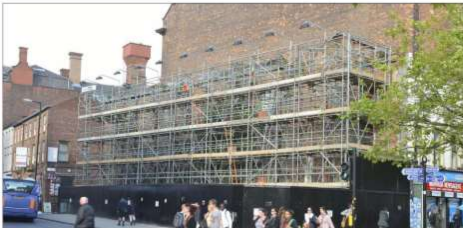
VIEW OF SCAFFOLD WITHOUT SHROUD
