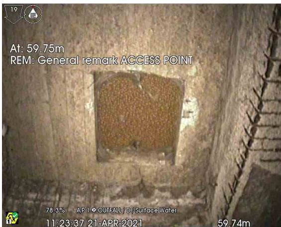
1_59-74m_112337.jpg, 00:07:13, 59.74 m General remark, ACCESS POINT
