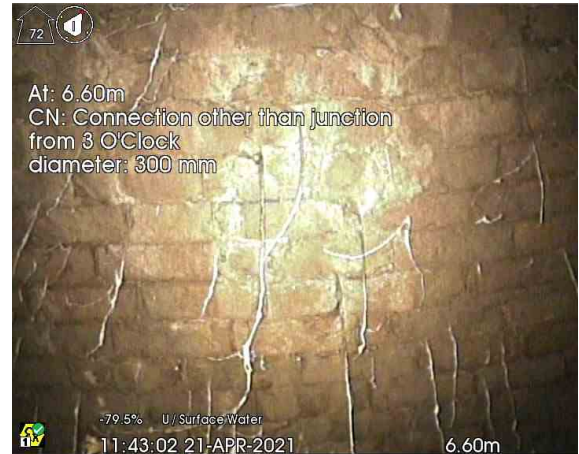
2_6-60m_114302.jpg, 00:04:21, 6.60 m Connection other than junction at 3 o'clock, diameter: 300mm
