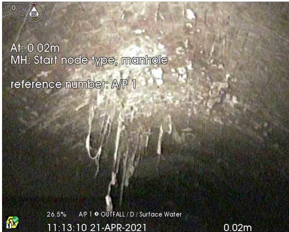
1_0-02m_111310.jpg, 00:00:03, 0.00 m Start node type, manhole, reference number: A/P 1
