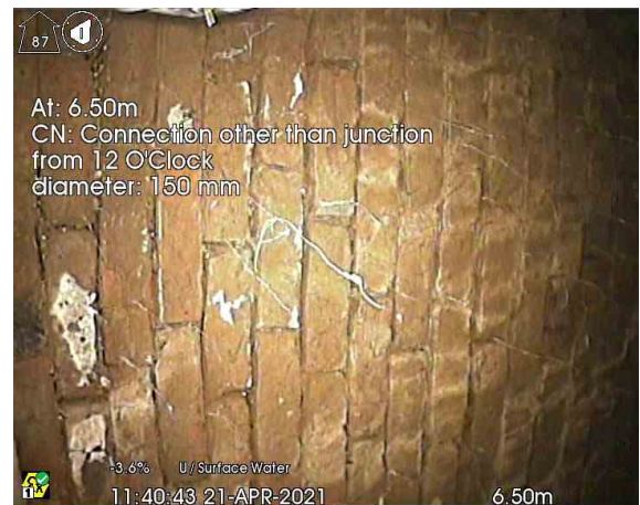
2_6-50m_114043.jpg, 00:02:18, 6.50 m Connection other than junction at 12 o'clock, diameter: 150mm
