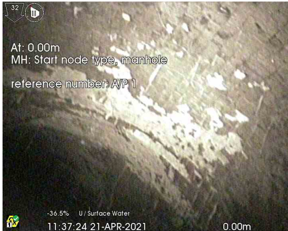
2_0-00m_113724.jpg, 00:00:01, 0.00 m Start node type, manhole, reference number: A/P 1
