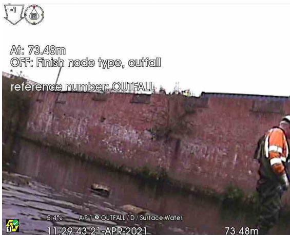
1_73-48m_112943.jpg, 00:10:12, 73.48 m Finish node type, outfall, reference number: OUTFALL
