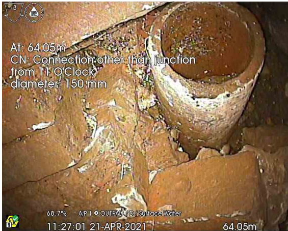
1_64-05m_112701.jpg, 00:08:51, 64.05 m Connection other than junction at 11 o'clock, diameter: 150mm
