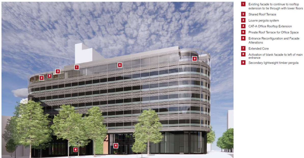
Figure 1-1: Proposed building refurbishment
