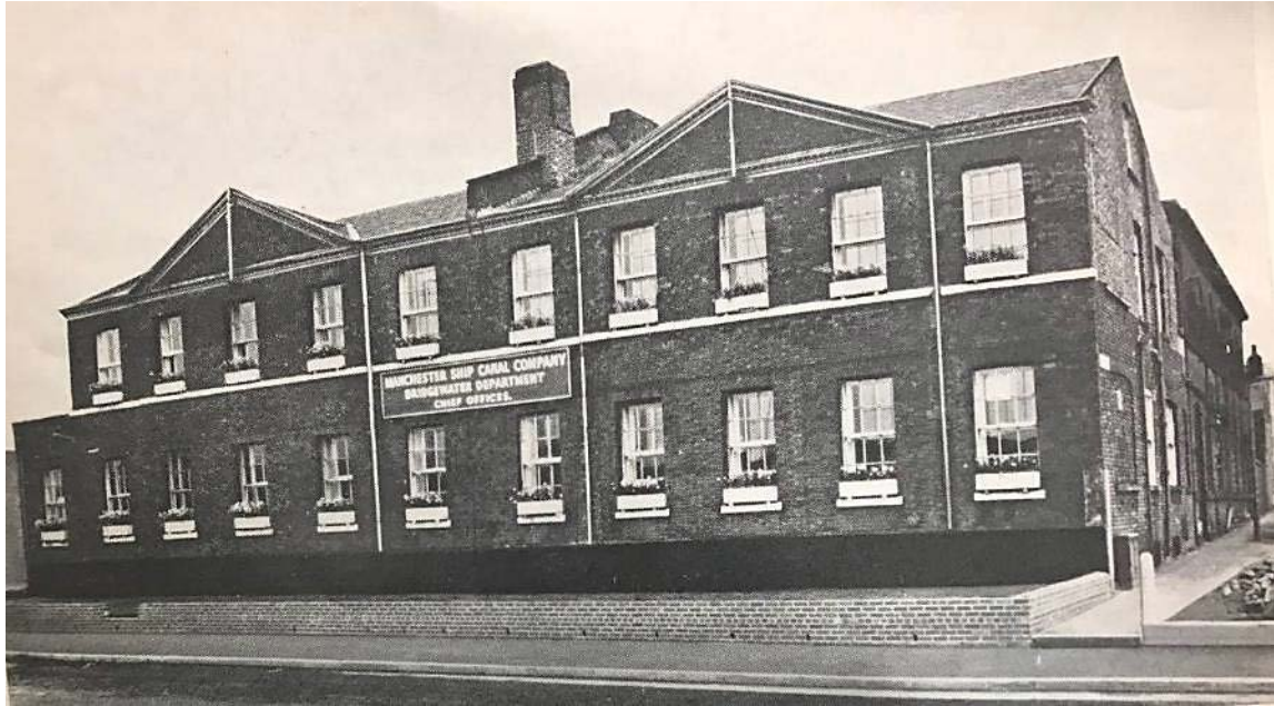
Figure 24: c1961/2 – This image shows the front of the site following the widening of Chester Road and the removal of much of the original front gardens and boundary walls/railings. This image was taken shortly after the construction of the current low-level garden wall in its new location, but before railings were erected. Note the basement windows have now been infilled, and a painted cement plinth added. Note the three original chimney stacks have now been removed. (Source: Manchester Archives)
