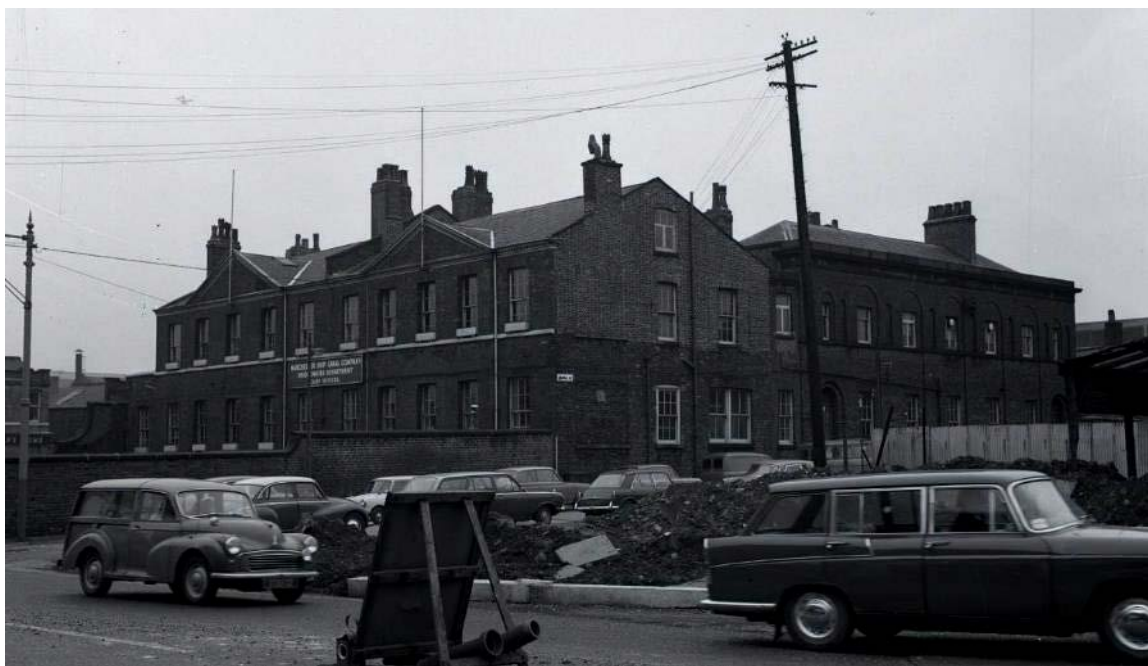
Figure 21: A view of the front and Crown Street elevation of Bridgewater House as seen in the early 1960s. (Source: Manchester Archives)
