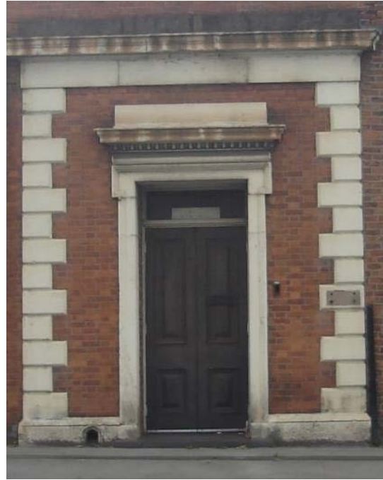
Figure 16: Photo showing the original red sandstone door surround and quoins, which were painted white in the late-20 th century.
