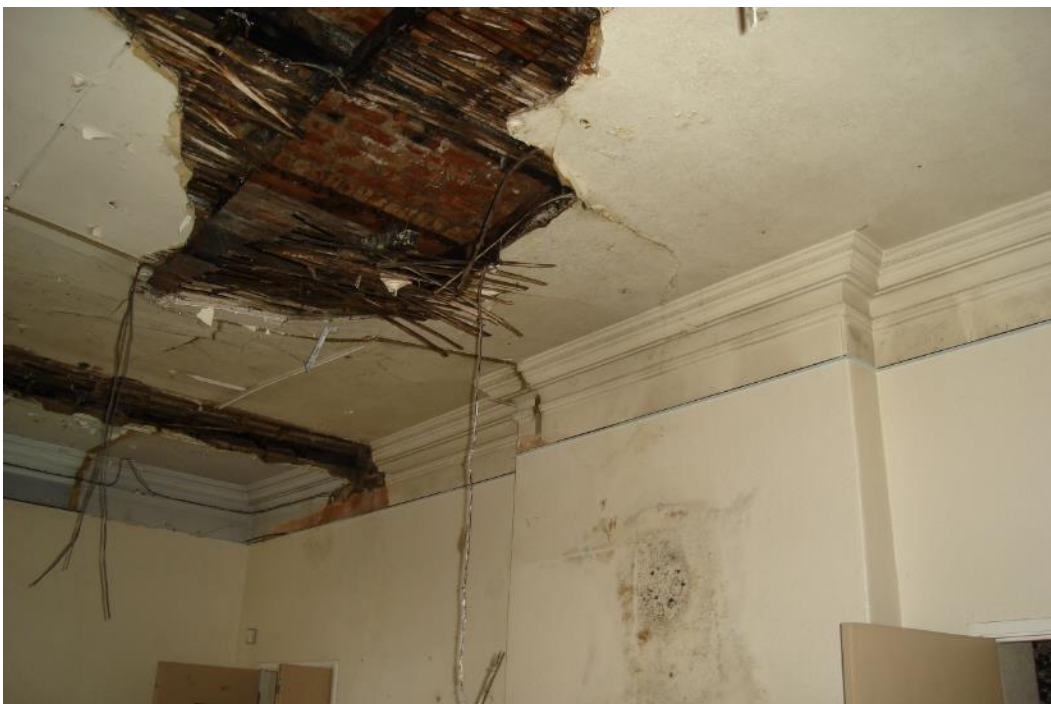
Figure 14: Room G16 as seen in 2007 showing the fireproof brick jack-arches concealed beneath the polite lath and plaster ceiling and cornice. (Note – the condition of office wing has since severely deteriorated with the loss of most original lath and plaster and cornice. (Source: SLHA)
