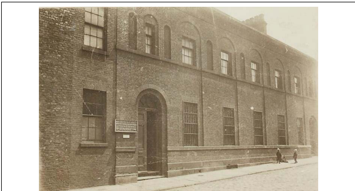
Figure 11: The c1842-3 Bridgewater Canal Company office on Crown Street, as seen here in c1920 when used by the Manchester Ship Canal as their offices, note the now removed original ground floor iron security railings to the windows, necessary due to the important records held within and the undesirable nature of the area (Source: Canal & Rivers Trust)
