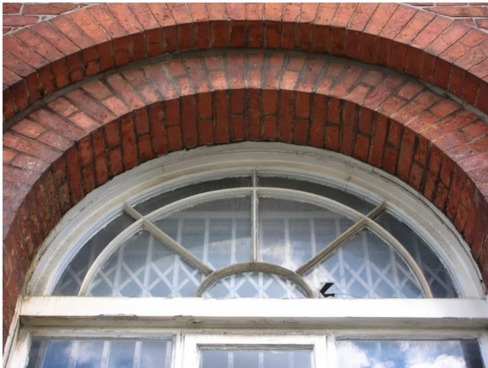
Figure 13a: The surviving original fanlight to the office extension as seen in 2007. (Source: SLHA 2017)
