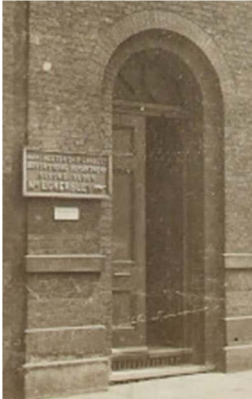
Figure 12: A closer view of the northern entrance door of the Crown Street office in c1920, showing the original panelled double doors. Note the original steps were on the inner side of the door originally (Source: Canal & River Trust)
