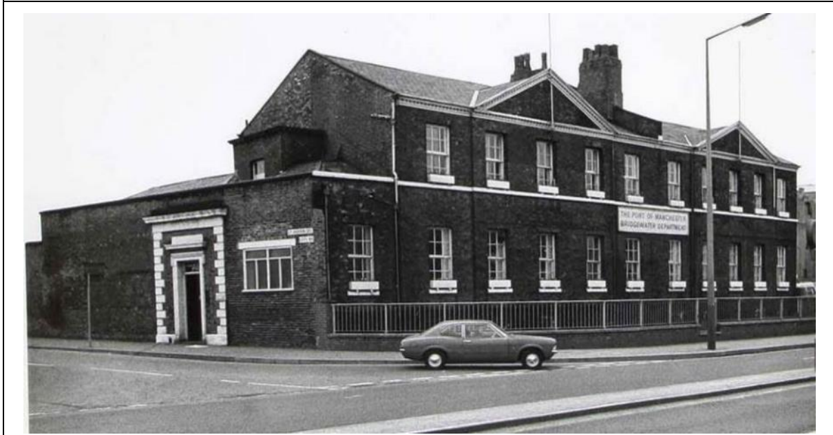
Figure 23: The same view as seen in 1975 following the widening of Chester Road and the subsequent shortening of the original gardens to the dwellings and demolition of the original perimeter walls and fences. Note the attic window has now been bricked-up. (Source: Manchester Archives)
