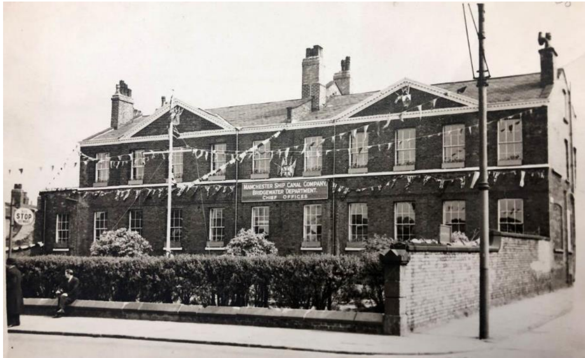
Figure 20: A view of the front of Bridgewater House in c1953, showing the original long boundary wall and railings. (Source: Manchester Archives)
