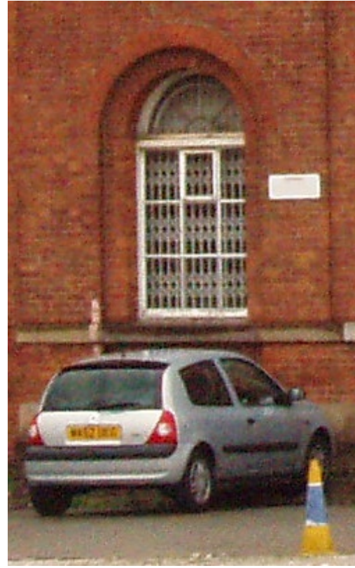
Figure 13: The same doorway as seen in 2007 showing the alterations undertaken by Securicor Limited in 1976 to convert the doorway into a window. Note the original surviving fanlight. (Source: SLHA 2007)
