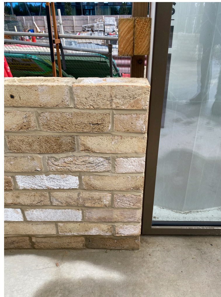
Left and above. Sample panel. TBS Mystique brickwork. Tarmac Y111 "Maize" mortar Tiger 68/60307 C33 Medium Bronze Anodised effect framing.
