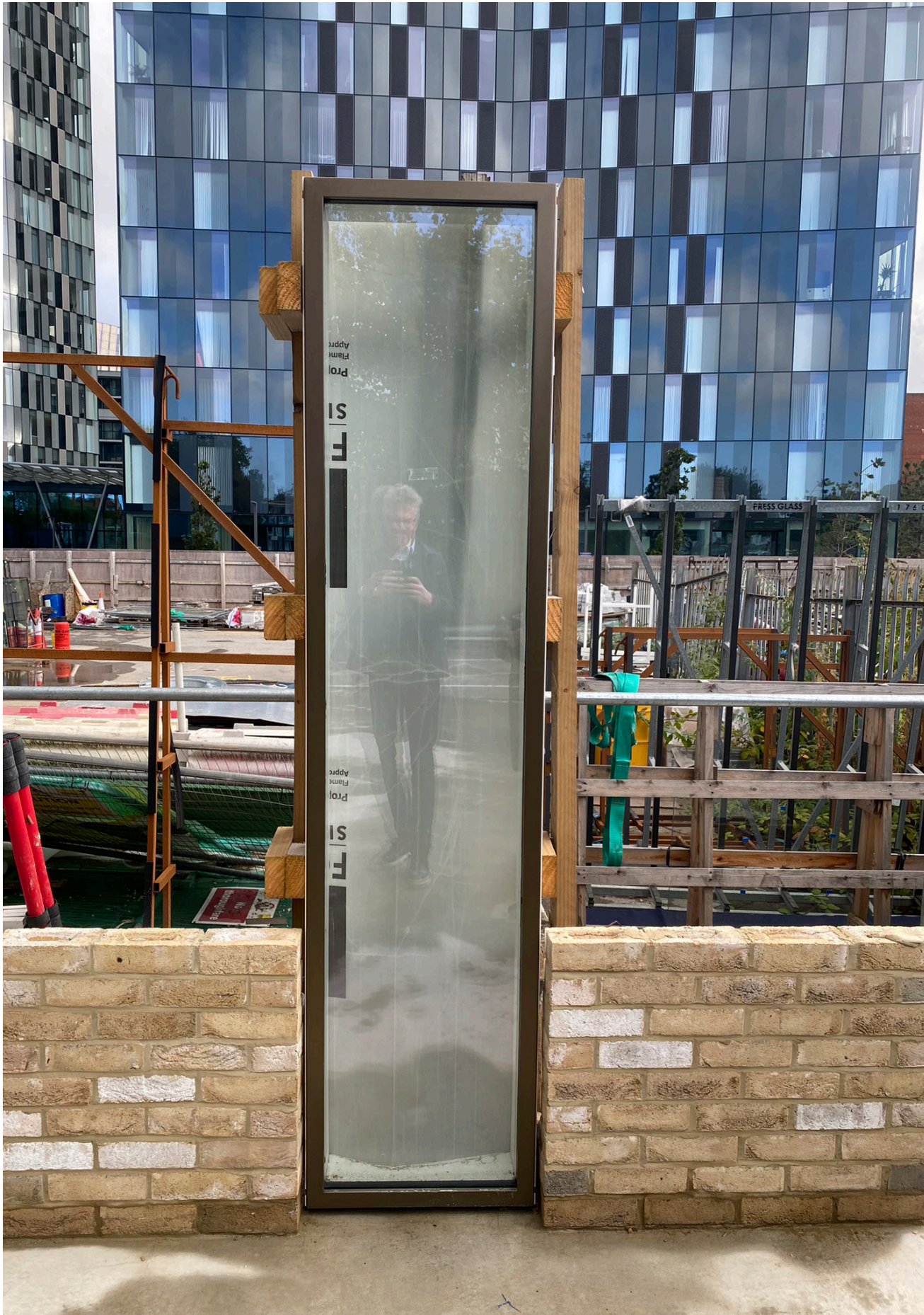
Left and above. Sample panel. TBS Mystique brickwork. Tarmac Y111 "Maize" mortar Tiger 68/60307 C33 Medium Bronze Anodised effect framing.
