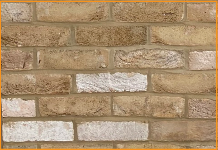
Brickwork, mortar and pointing
