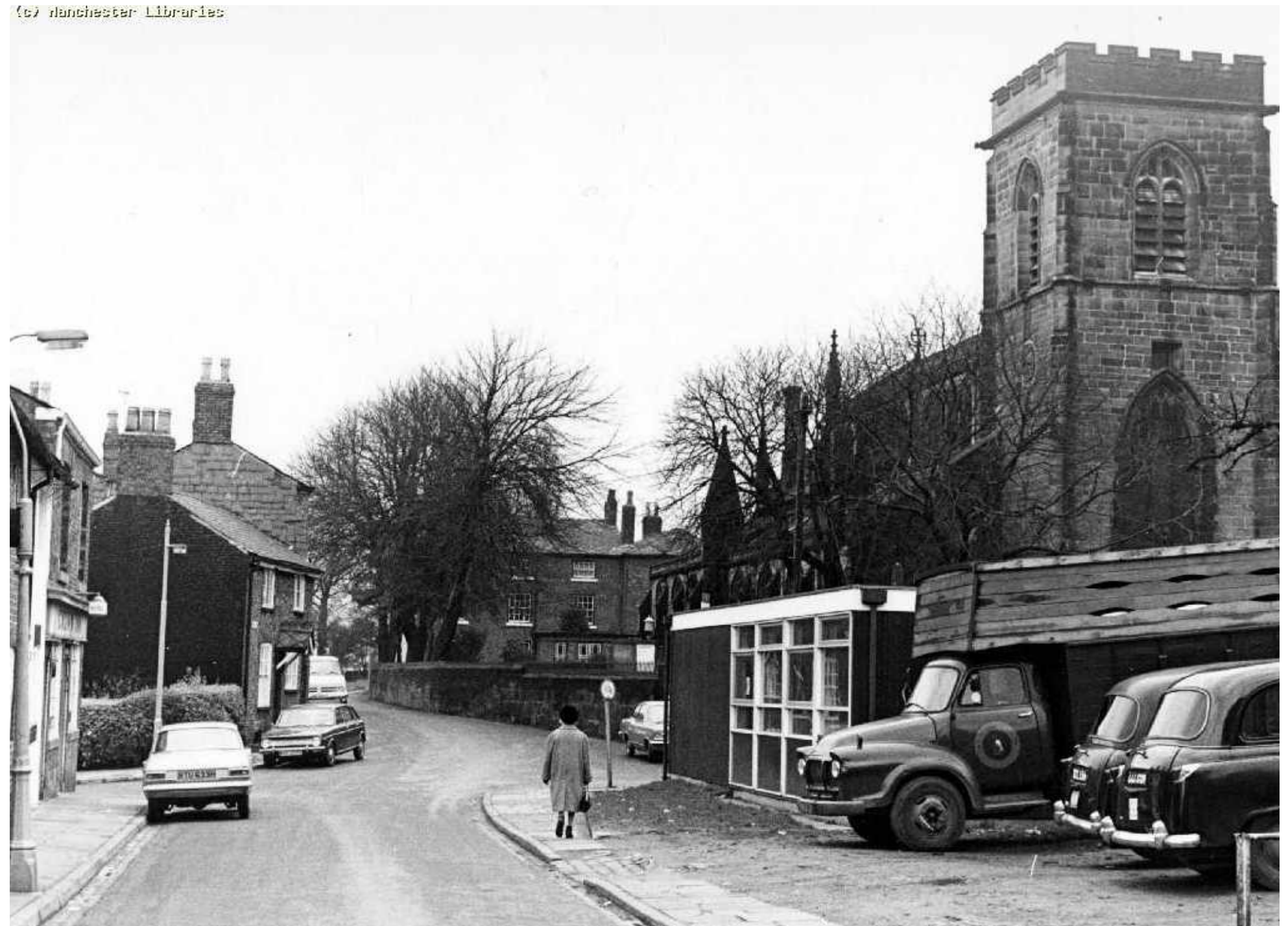
Figure 13 Photograph dating from 1971 looking east along Ford Lane with Northen House to the left and St Wilfred's Church to the right (Source: http://images.manchester.gov.uk , accessed 10th May 2022).
