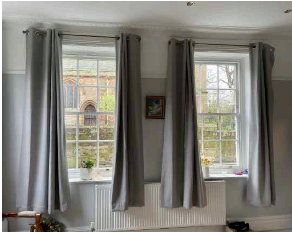
2 View looking towards the existing Master Bedroom windows overlooking the Church
