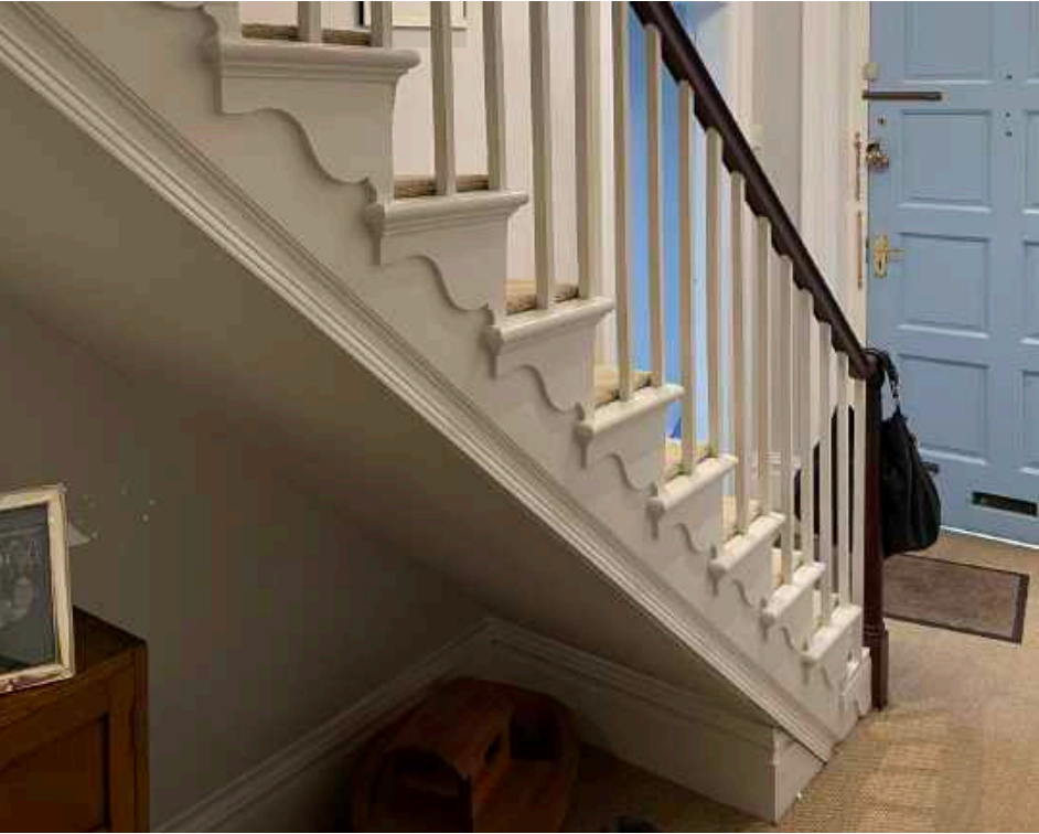
1 View looking towards the existing stair and front door to the Georgian south wing
