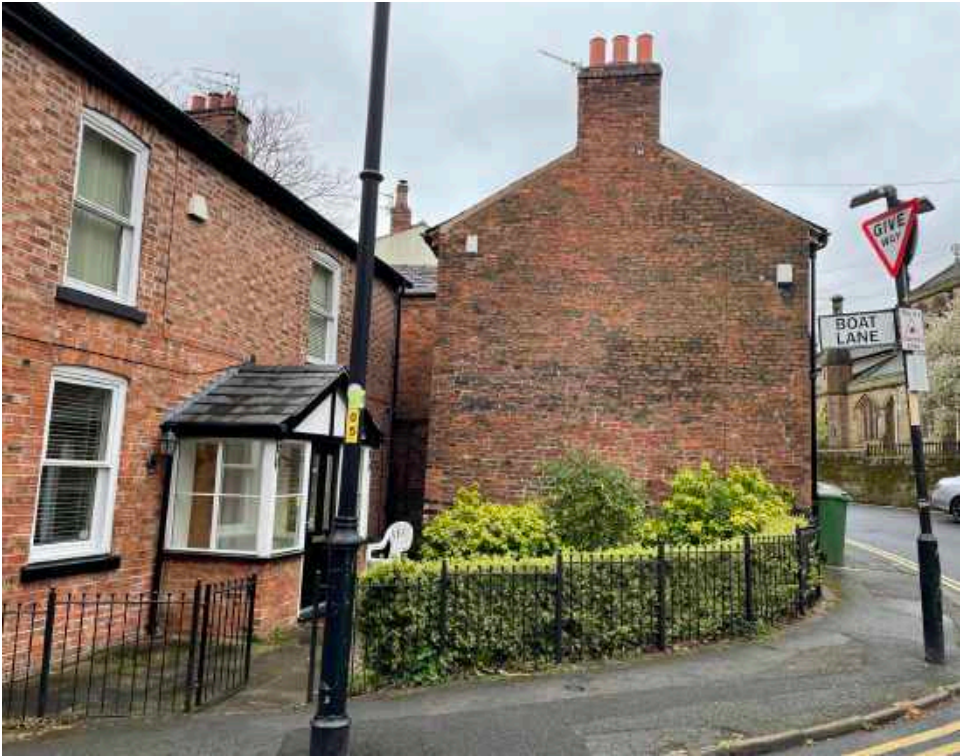
3 View looking east from Boat Lane looking towards Northern House
