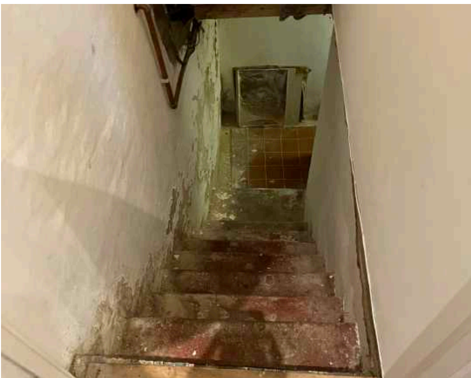
5 View looking down into the Cellar
