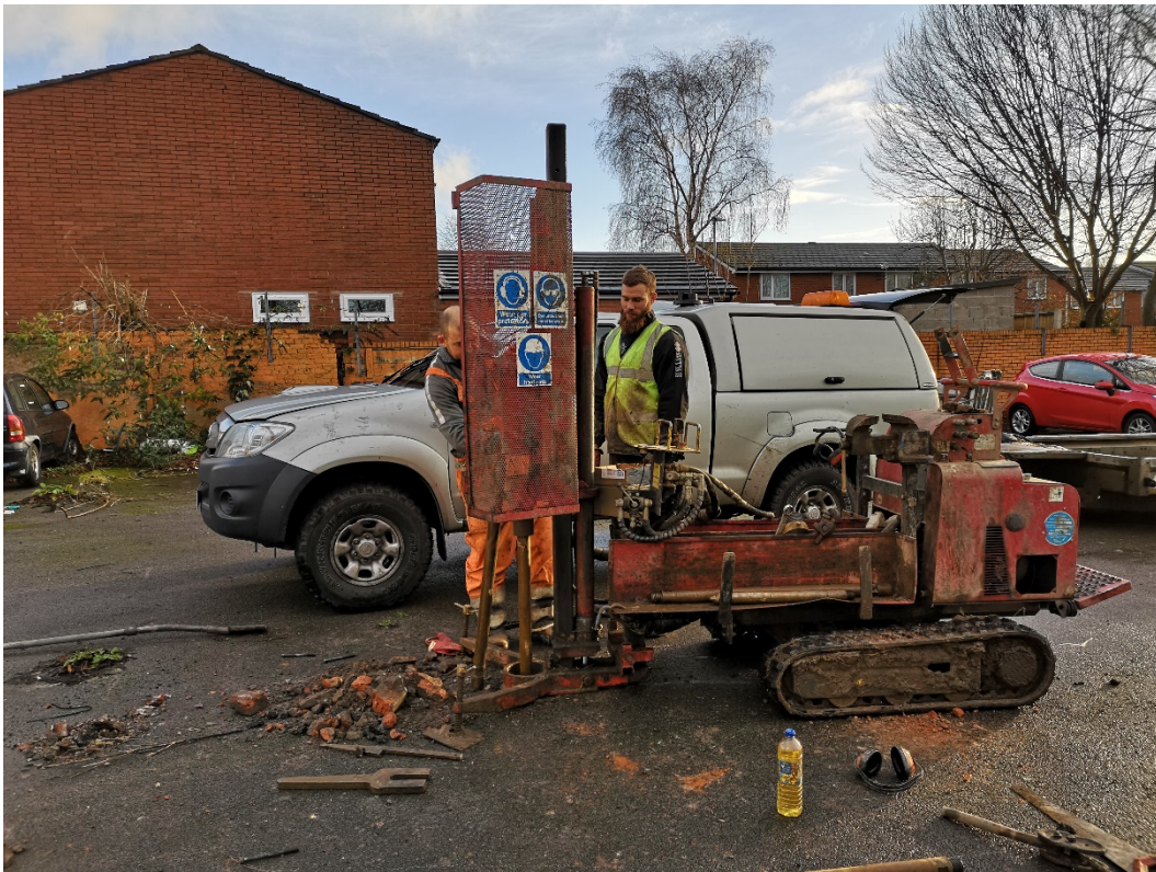
Figure 4 Drilling rig in position WS1
