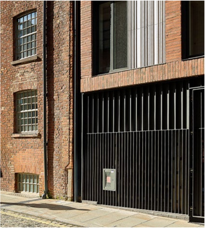
Precedent imagery showing PPC steelwork slatwork at the base of Murray Mills, within the Ancoats Conservation Area.
