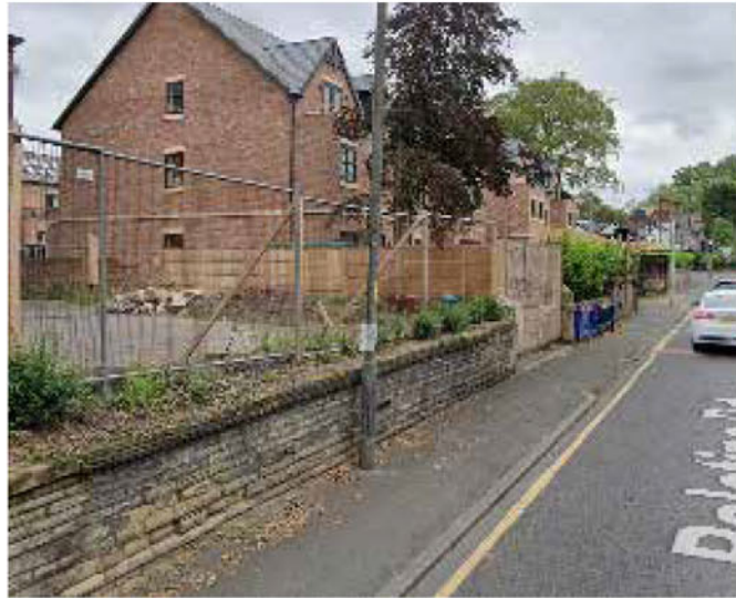
Stone Frontage Wall reinstated
