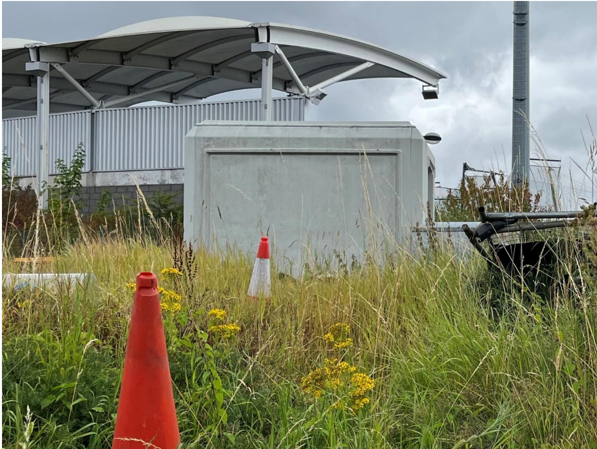
Figure 6: Building B1, located in the east of the site, looking east
