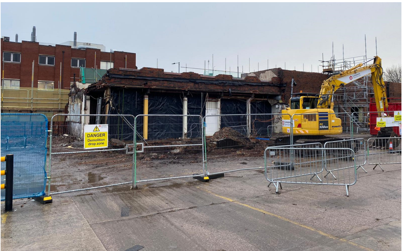
Photograph 4 – Demolition of buildings
