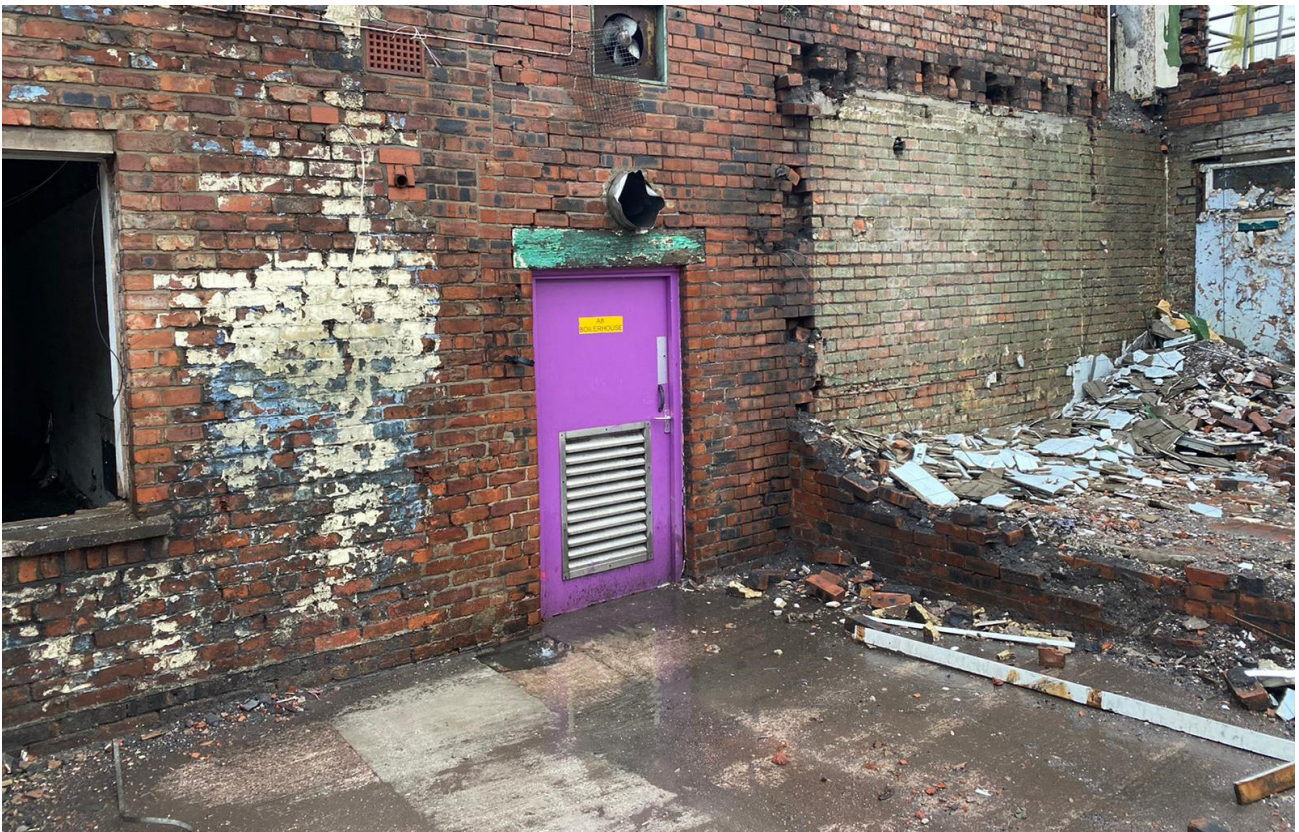
Photograph 3 – Boiler house room in north west area
