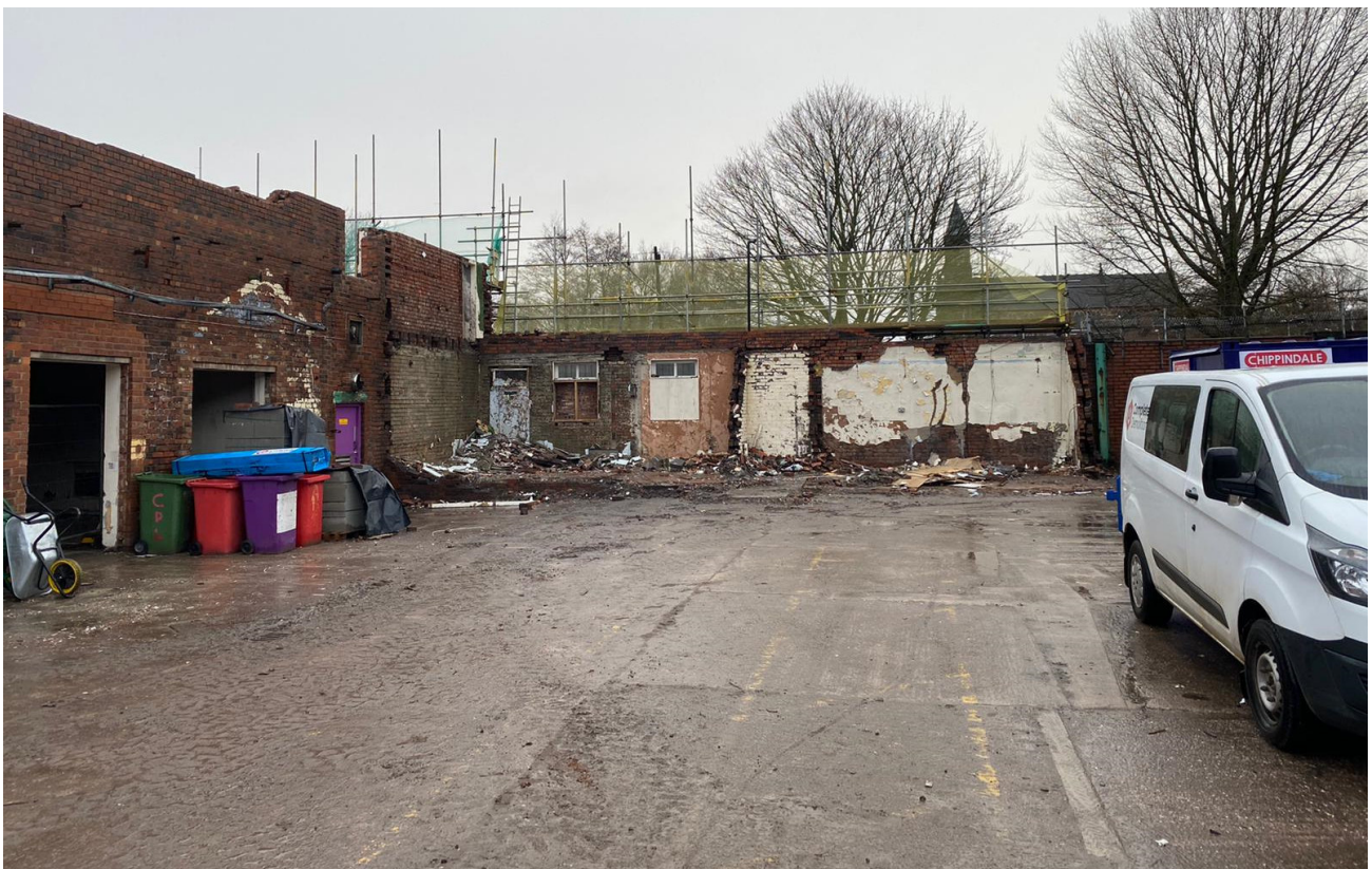
Photograph 2 – Buildings being demolished
