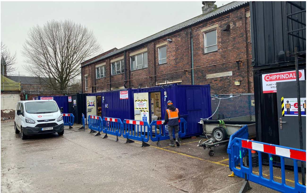
Photograph 1 – Existing chemical works buildings
