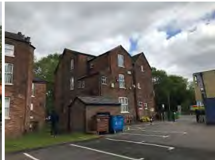
Southern view of eastern building
