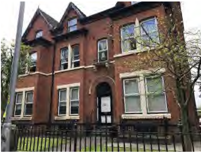
View from Moss Lane of eastern building
