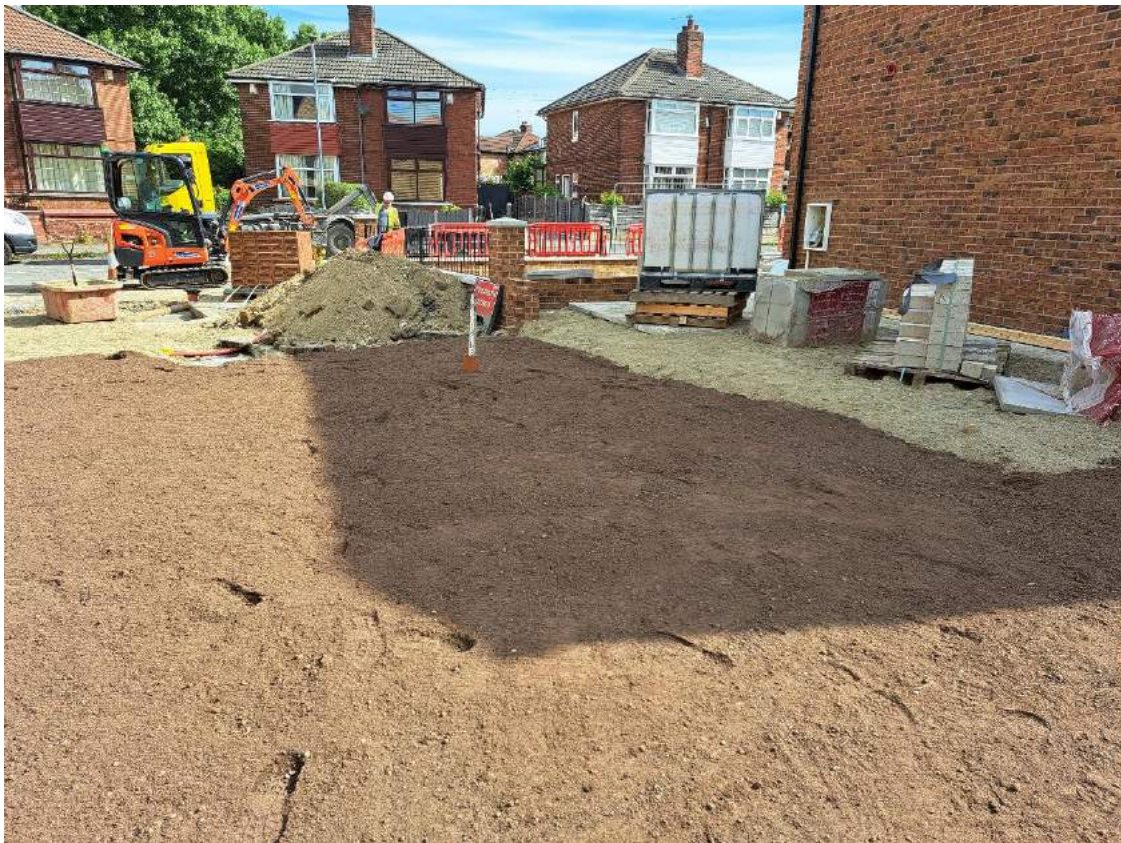
Photograph 2 Landscaped area showing VP01 location prior to completion of topsoil capping.
