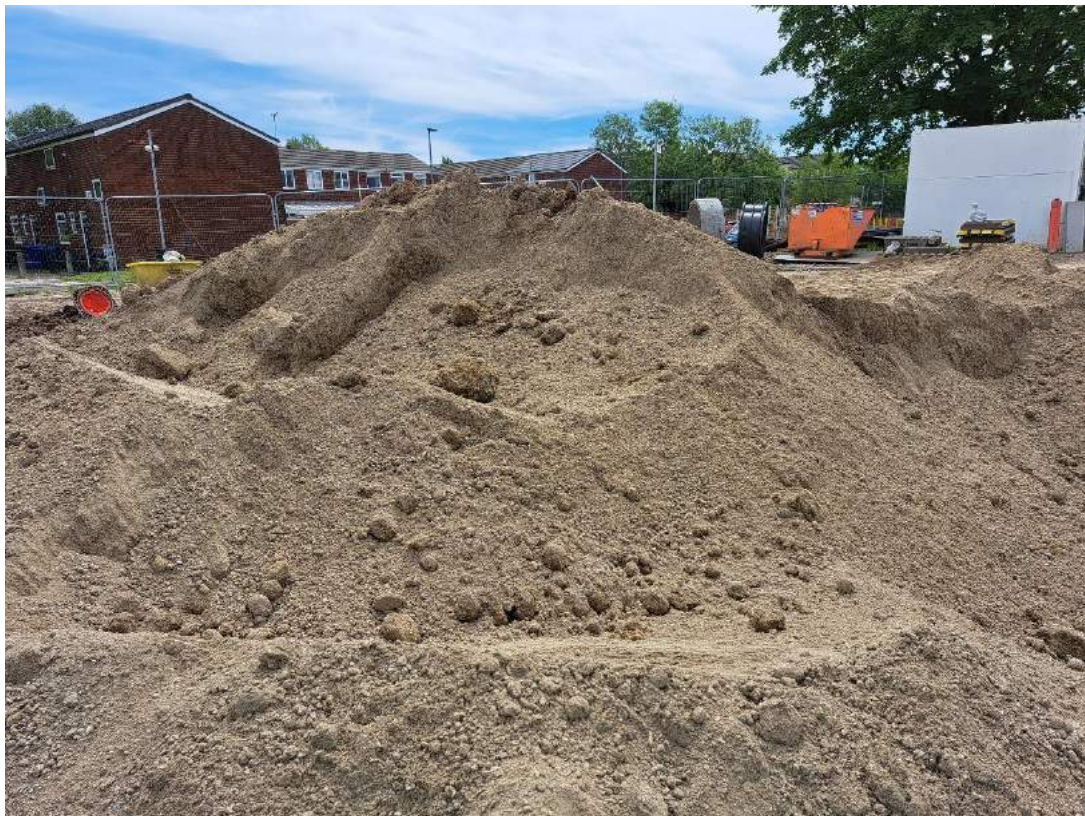
Photograph 40 Stockpiled imported subsoil prior to emplacement.
