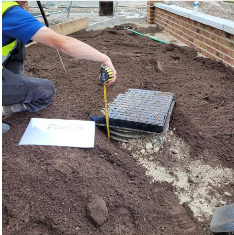
Photograph 45 Confirmation of 200mm topsoil emplaced into Plot 6 front garden.
