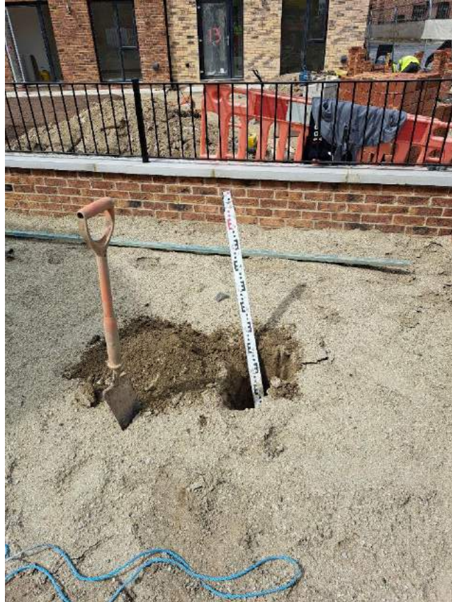
Photograph 31 Landscaped area showing imported subsoil at VP12 prior to topsoil import.
