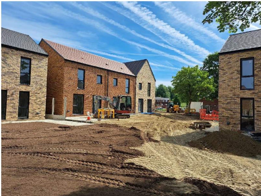
Photograph 42 Overview of rear garden areas showing progressive placement of topsoil over imported subsoil on 16 th June 2022.
