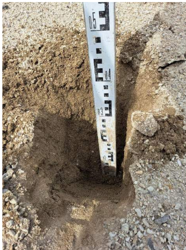
Photograph 30 450mm of subsoil emplaced in VP12 prior to the placement of 150mm topsoil.
