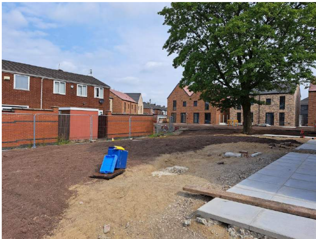
Photograph 47 Capping soils emplaced to rear of Plots 18 to 21, including around retained tree.
