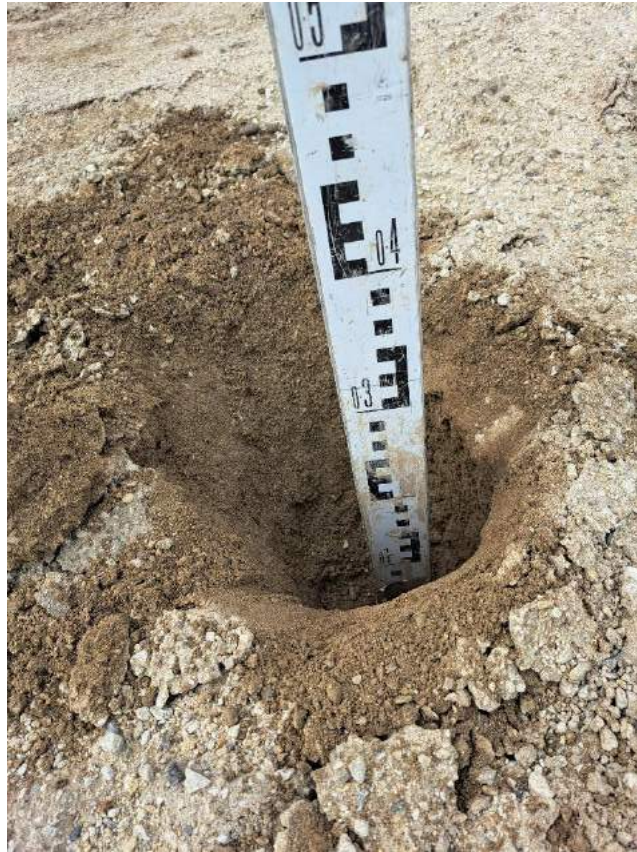
Photograph 25 300mm of subsoil emplaced in VP10 prior to the import of topsoil.
