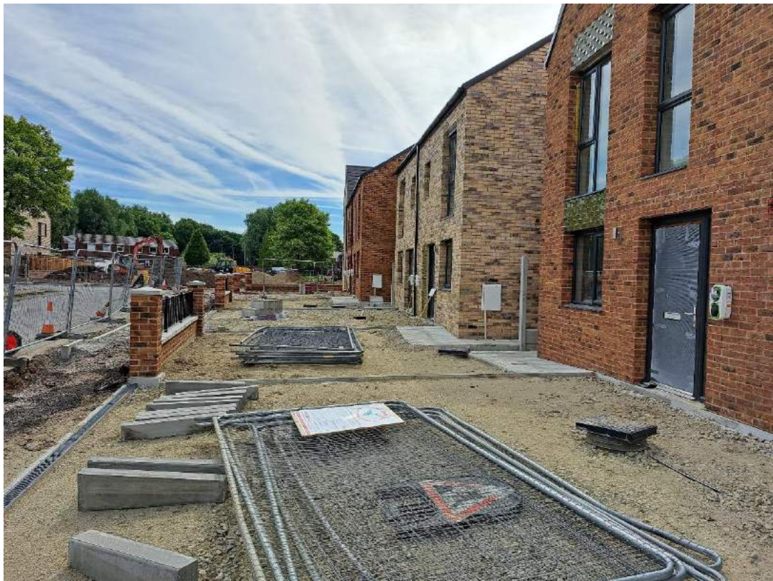
Photograph 44 Overview of front garden areas of Plots 6 to 12, showing partial cover system in place on 16 th June 2022.
