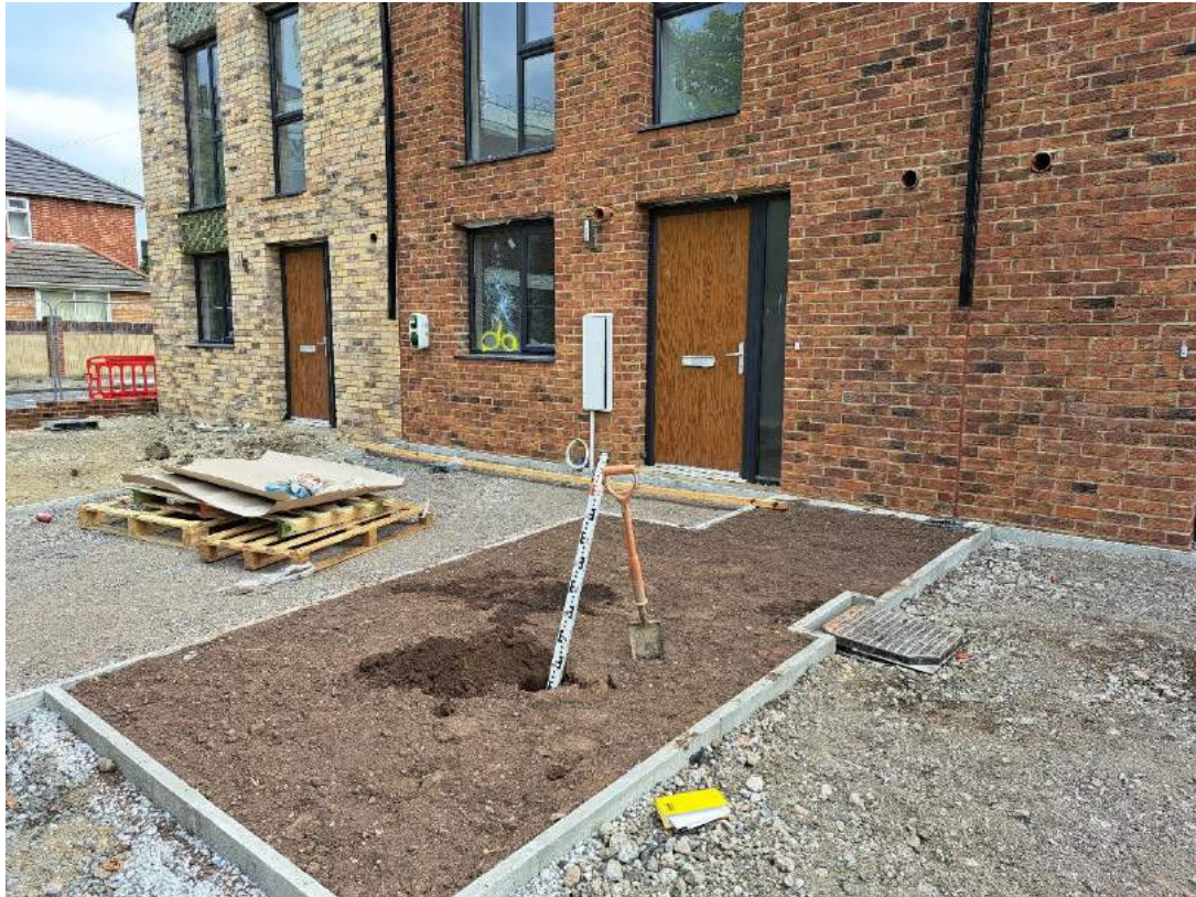
Photograph 37 Overview of landscaped area at VP15 following soil emplacement.
