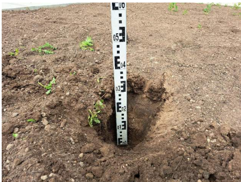
Photograph 14 Confirmation of 350mm of topsoil emplaced in VP06 following additional soil import.
