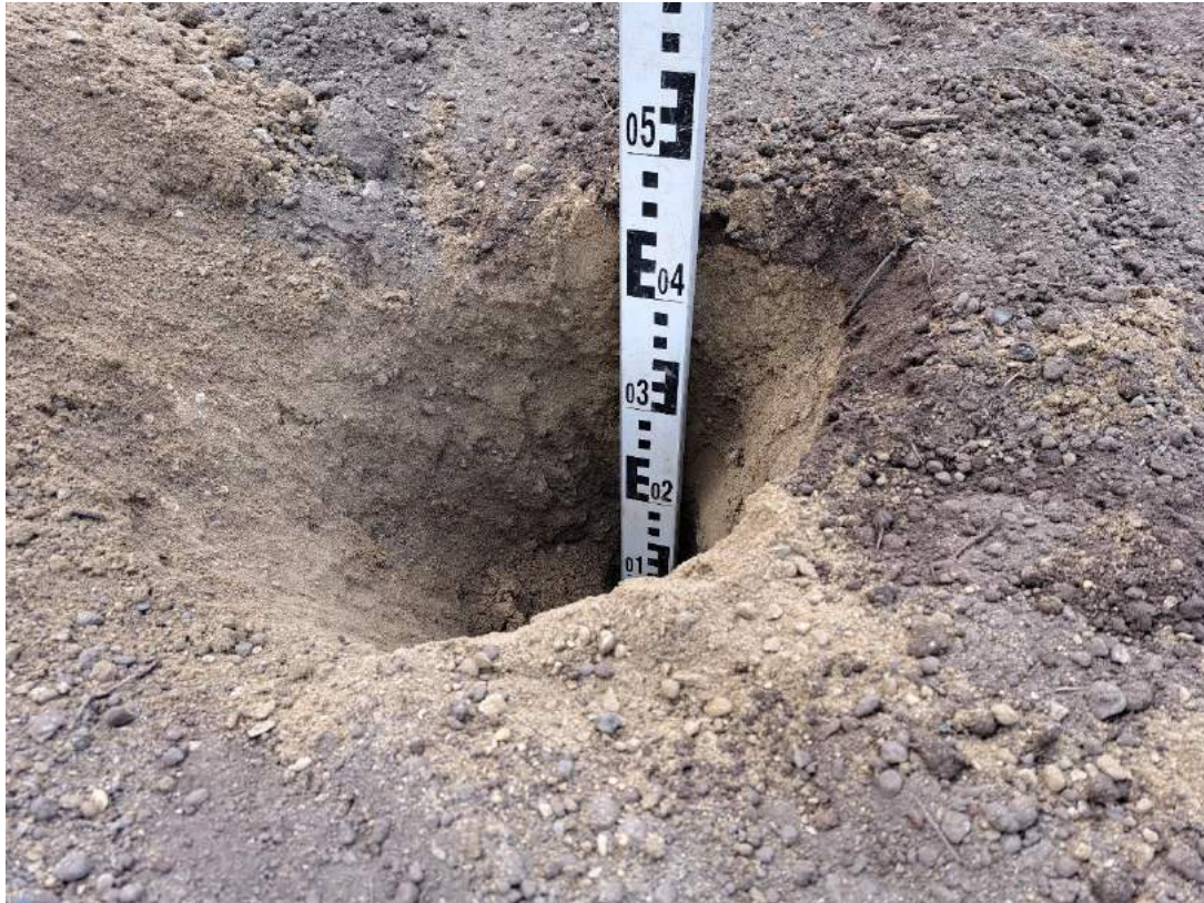
Photograph 35 450mm of imported subsoil emplaced at VP14 prior to 150mm topsoil placement.
