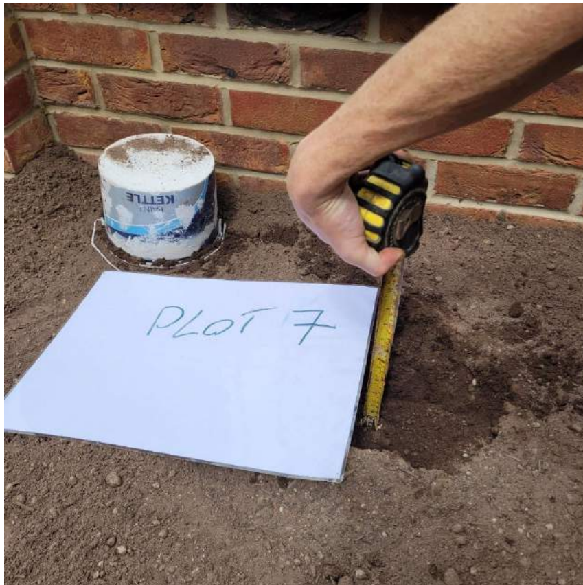
Photograph 26 Landscaped area showing 250mm imported topsoil at VP10.
