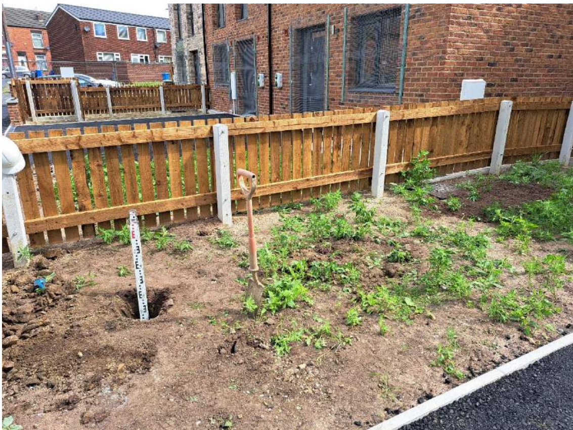
Photograph 20 Landscaped area showing emplaced soil at VP08. The site manager confirmed the area would be rotavated prior to finalisation.
