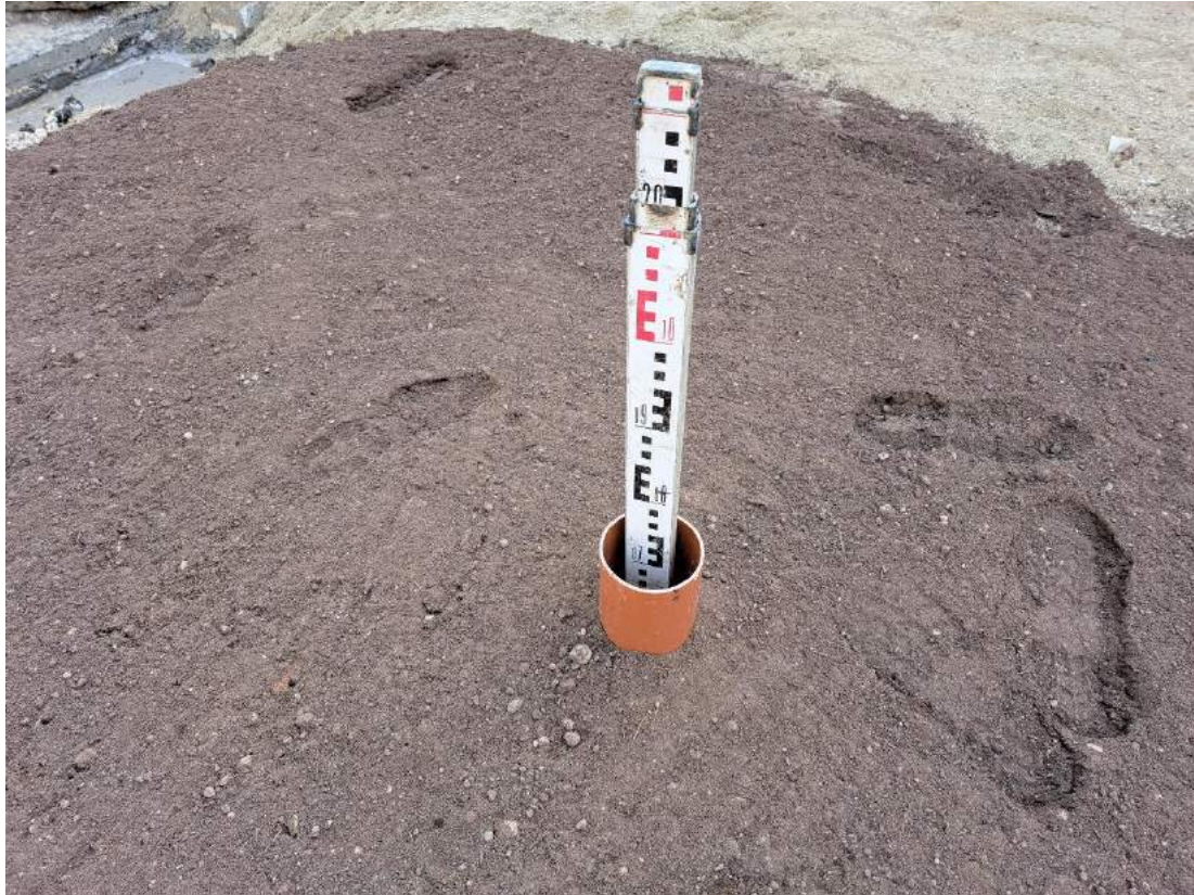
Photograph 1 150mm of topsoil and 450mm of subsoil emplaced in VP01.
