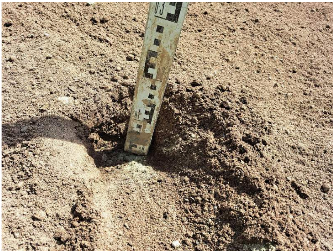
Photograph 33 150mm of topsoil emplaced at VP13 following original pit excavation.
