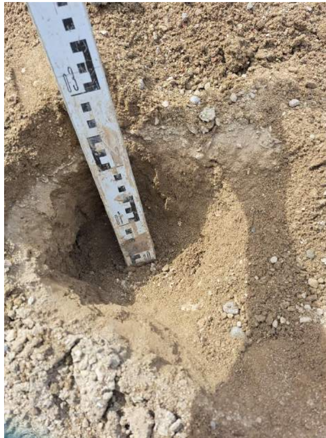
Photograph 28 300mm of subsoil emplaced in VP11 prior to the placement of topsoil.
