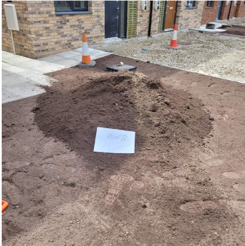
Photograph 29 Landscaped area at VP11 following 150mm topsoil import.
