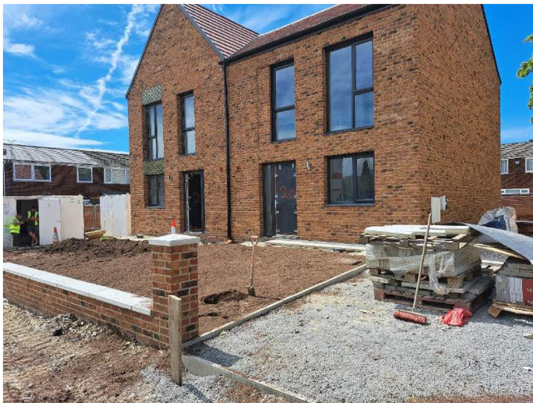
Photograph 34 Landscaped area showing imported topsoil at VP13.
