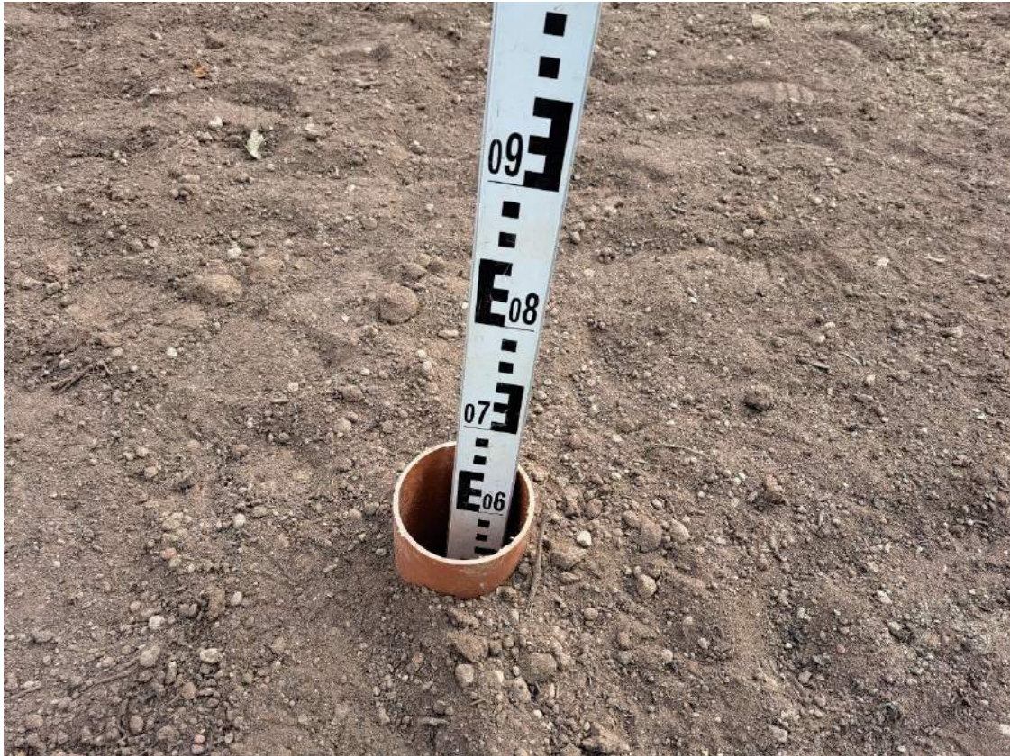
Photograph 11 150mm of topsoil emplaced over subsoil at VP05.
