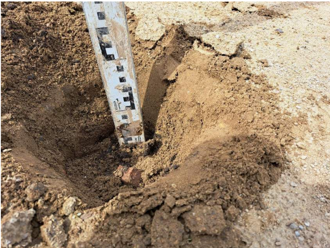
Photograph 22 200mm of subsoil emplaced in VP09 prior to the import of topsoil.
