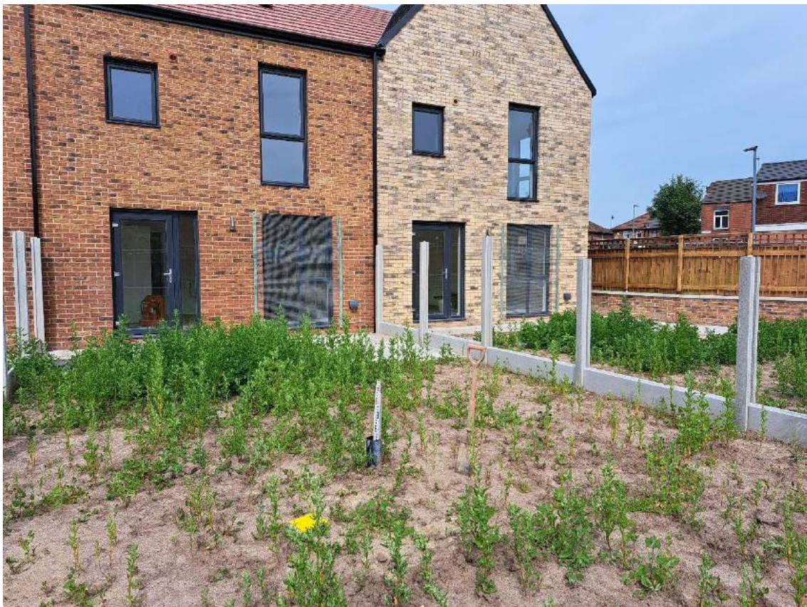
Photograph 18 Landscaped area showing emplaced soil at VP07. The site manager confirmed the area would be rotavated prior to additional topsoil placement.
