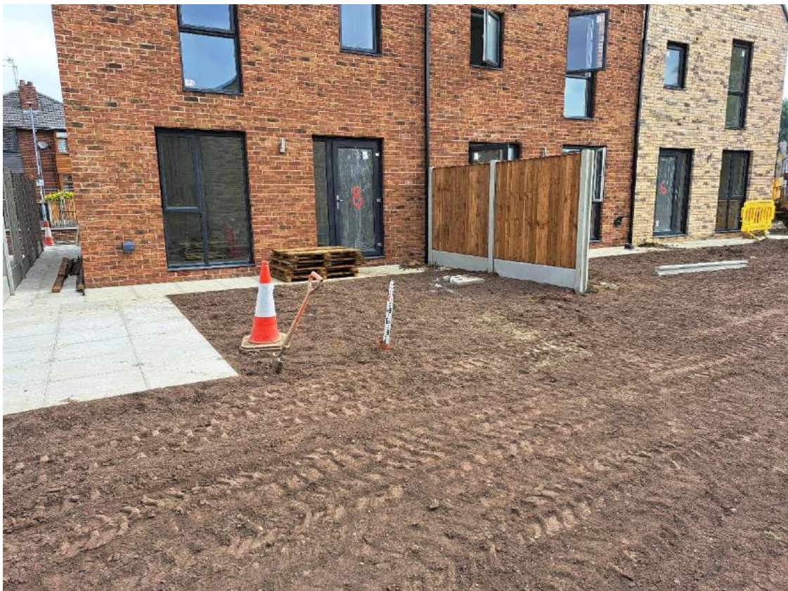
Photograph 12 Landscaped area at VP05 following placement of topsoil.
