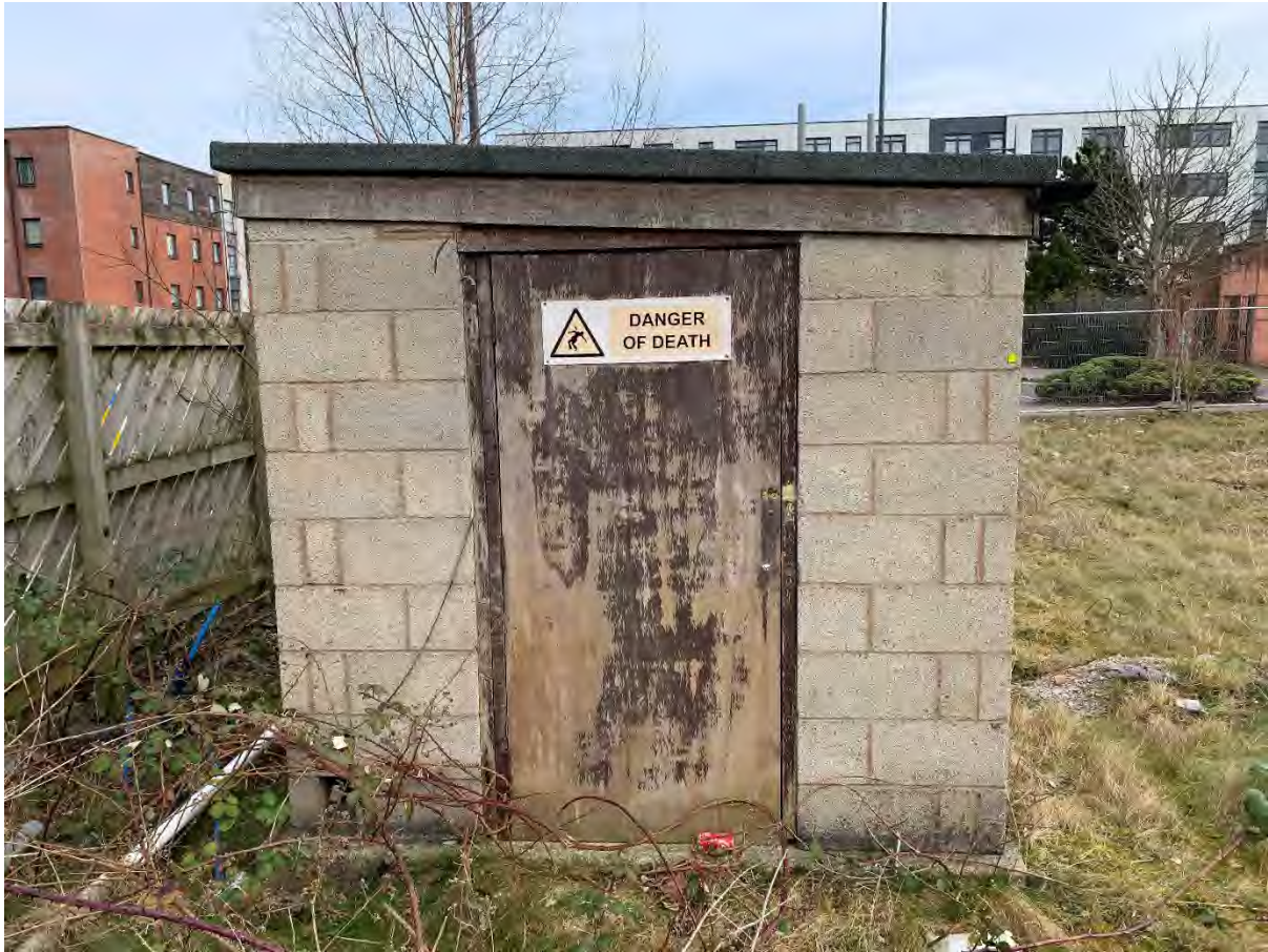
Photograph 6: View of disused breeze block services buildings
