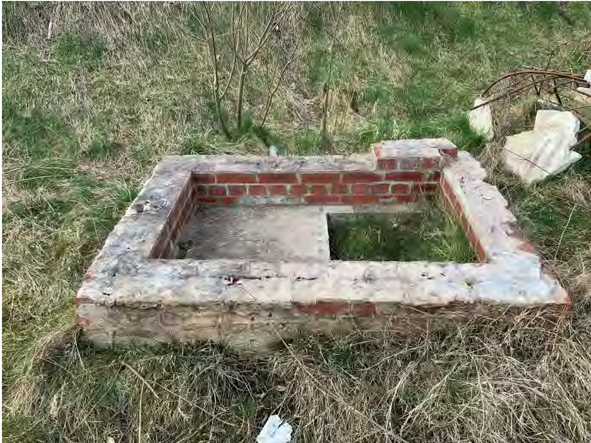
Photograph 7: Brick footing related to services building
