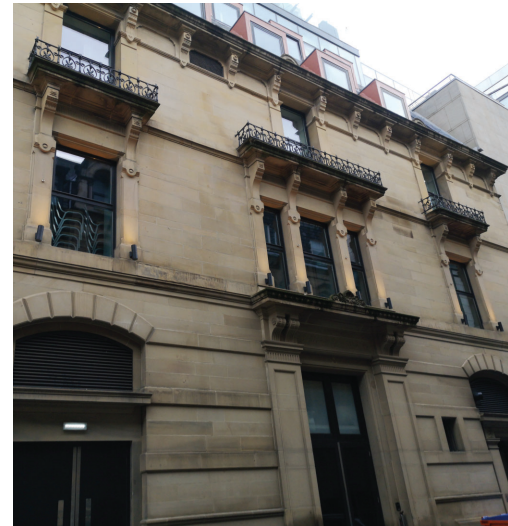
Existing Facade Lighting - Kennedy Street Facade
