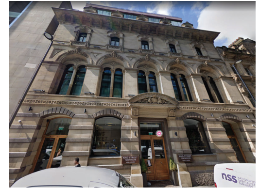
Street View - Booth Street Facade
