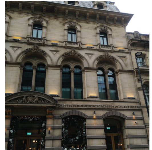
Existing Facade Lighting - Booth Street Facade
