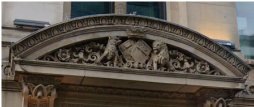
Entrance canopy ornamental pediment detail
