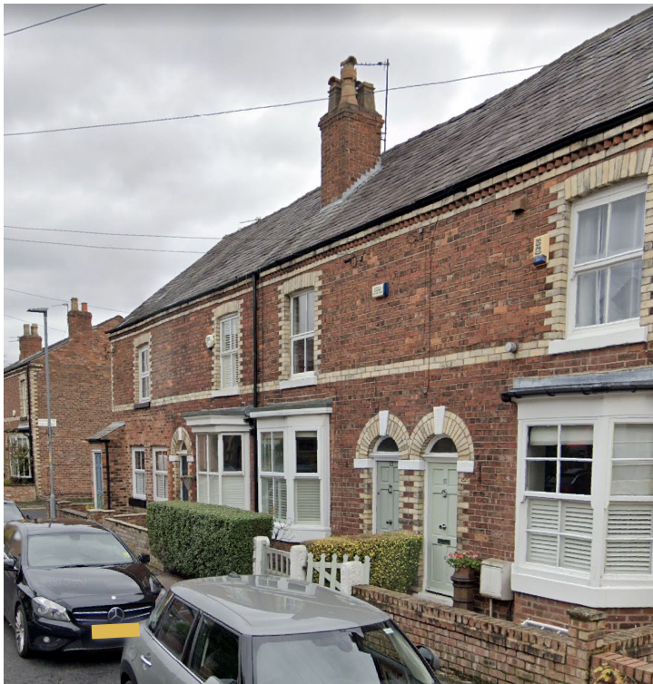
View along Gillbrook Road Existing white brick window reveals and arched lintels
