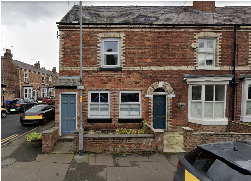
Gillbrook Road Street Elevation Historic alterations to the frontage have made no. 9 Gillbrook Road distinct from the neighbouring properties. Pitched roof porch is a later addition.
