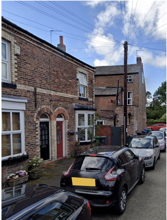
Rear View from Rushton Street
