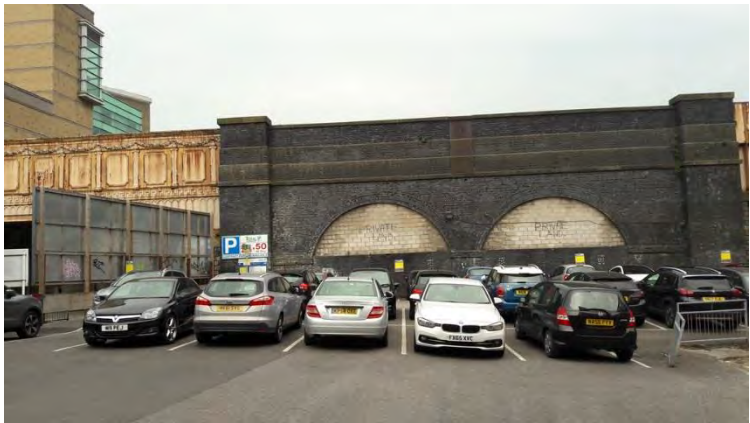
Photograph 1 (P1) View to the south with car park and disused railway viaduct visible.
