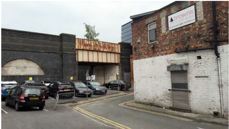
Photograph 3 (P3) The existing commercial building and Breslyn Street.
