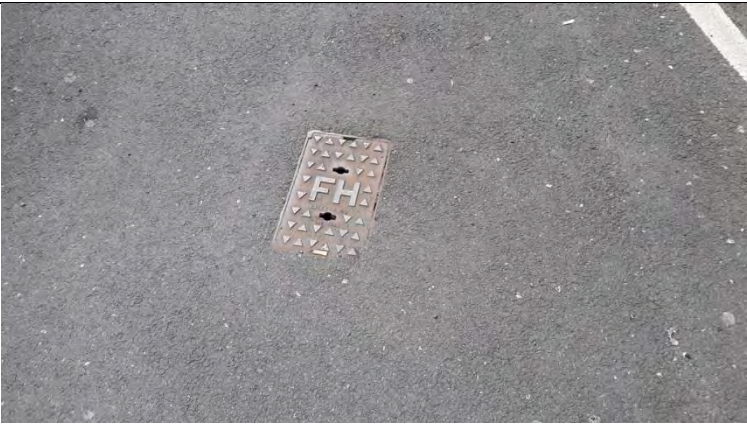
Photograph 6 (P6) Fire hydrant cover located in the south east of the car park.
