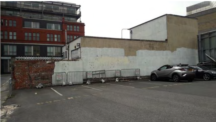
Photograph 2 (P2) View to the north from car park with adjacent retail premises visible.
