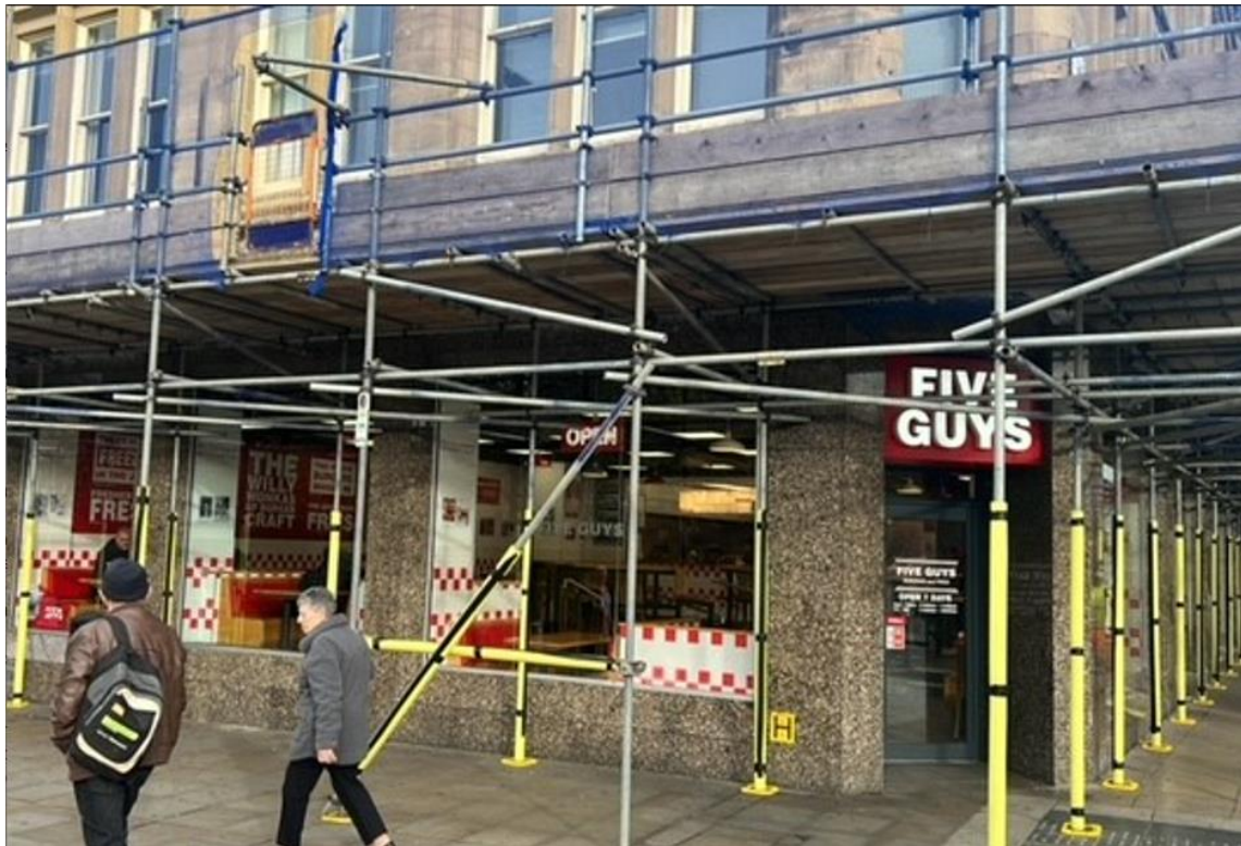
Figure 1: Current scaffolding surrounding existing Five Guys restaurant unit
