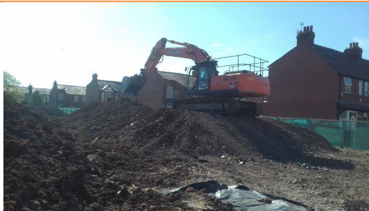
PLATE 9 – CONTAMINATED MATERIAL BEING TURNED
