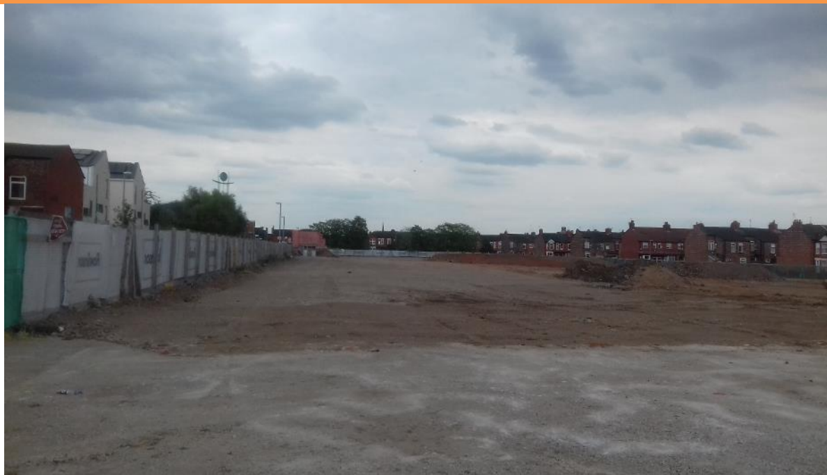
PLATE 11 – INFILLED SOURCE AREA 1
