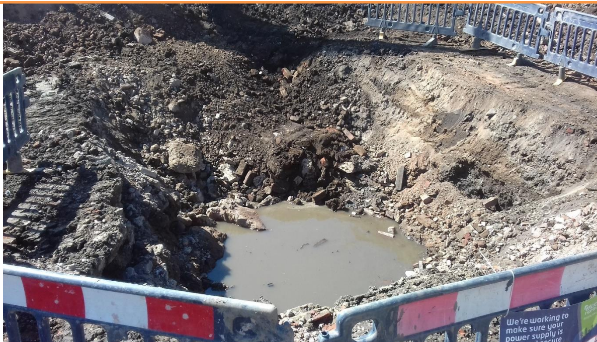
PLATE 28 – POST DEMOLITION EXCAVATION BENEATH SUBSTATION
