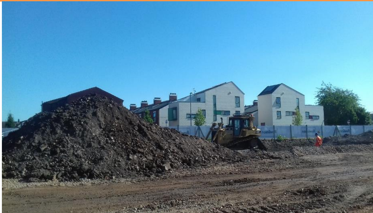
PLATE 8 – TOP 1.0m OF RETAINED MATERIAL FROM SOURCE AREA 1
