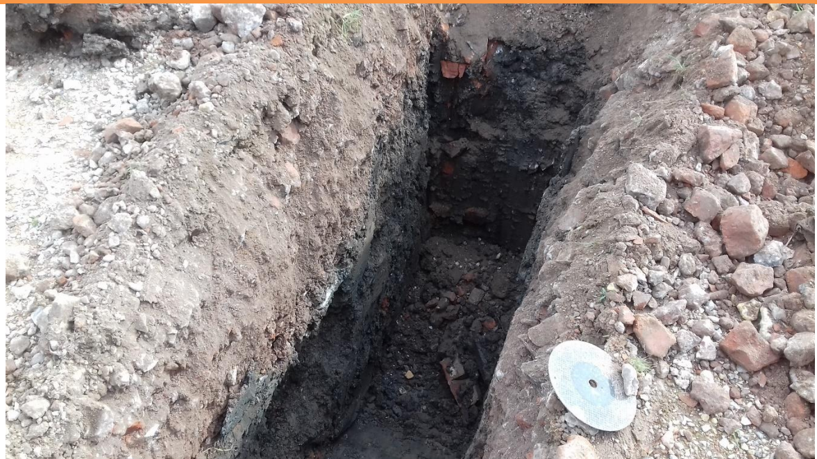
PLATE 25 – PRELIMINARY TRIAL PITS IN VINICITY OF SUBSTATION
