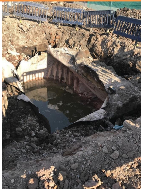
PLATE 32 – IN SITU UNDERGROUND TANK BENEATH FORMER SUBSTATION
