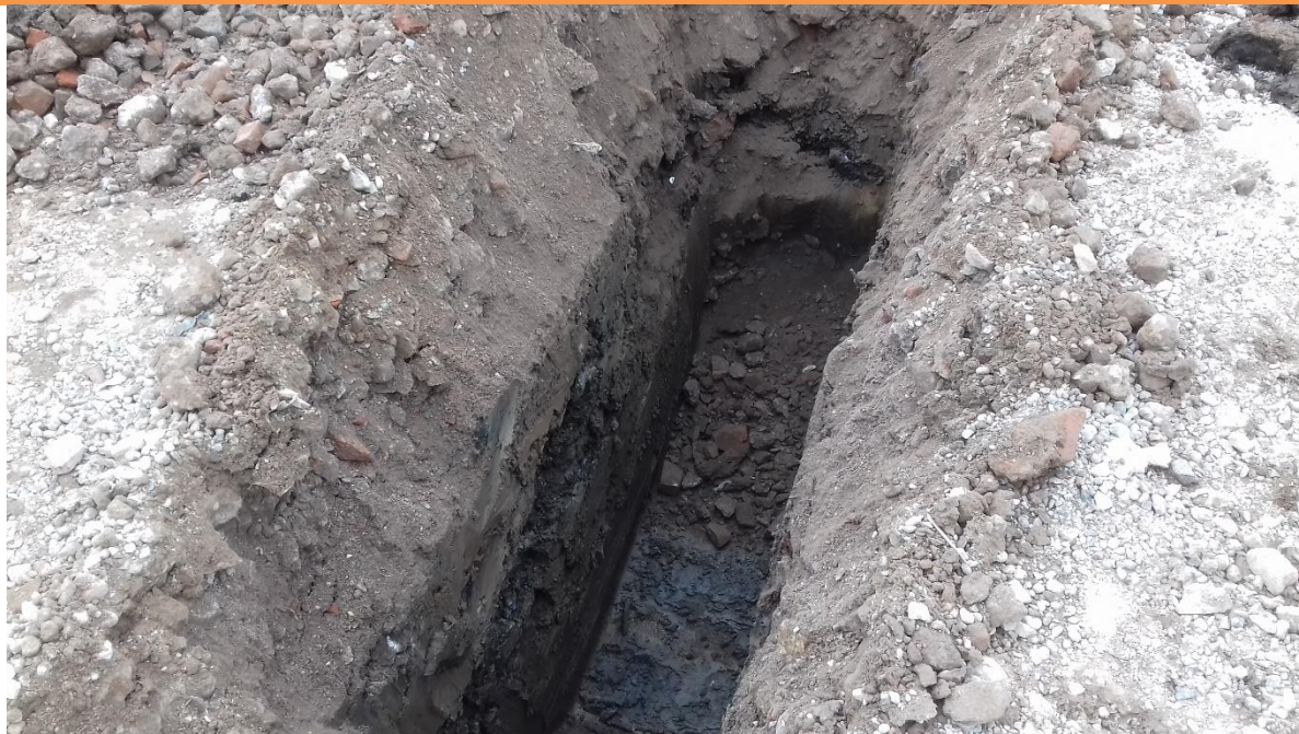
PLATE 24 – PRELIMINARY TRIAL PITS IN VINICITY OF SUBSTATION
