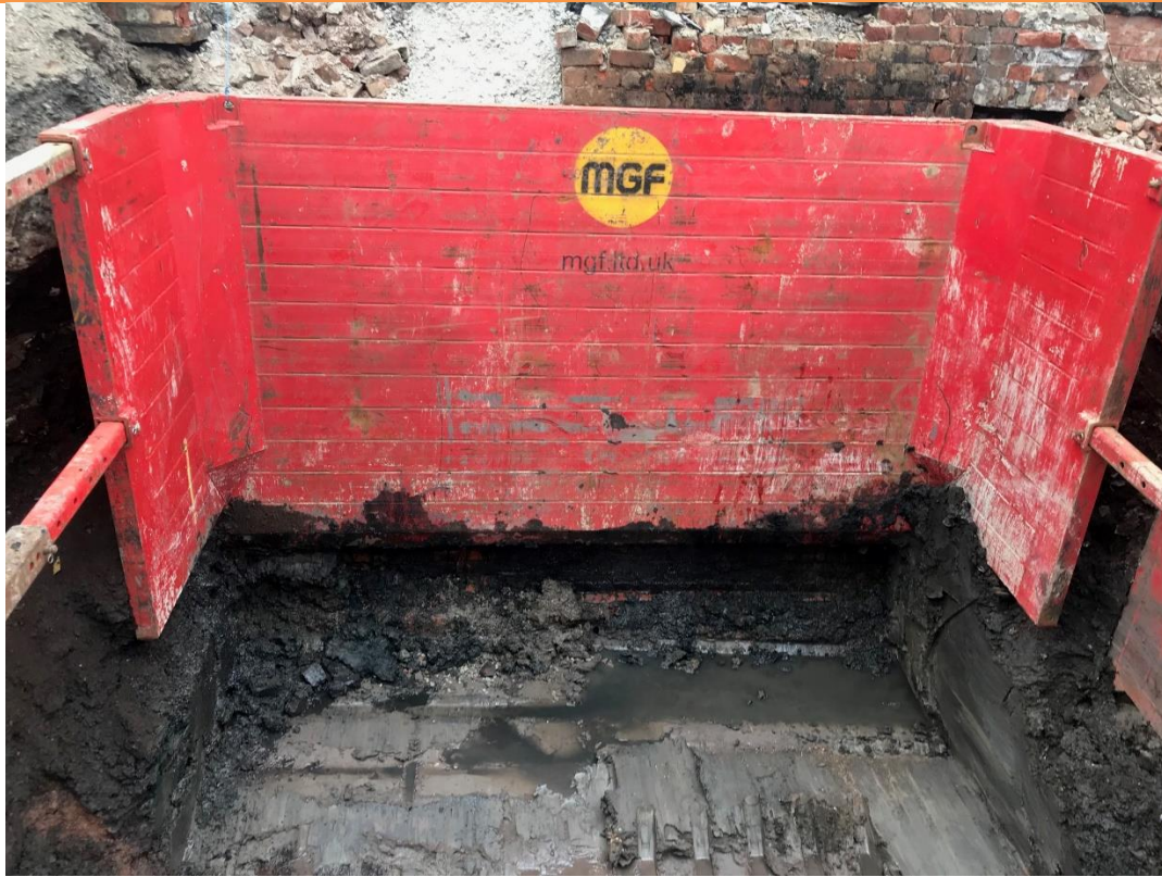
PLATE 31 – CLEAN BASE AND BATTERED SIDES OF EXCAVATION DURING VALIDATION
