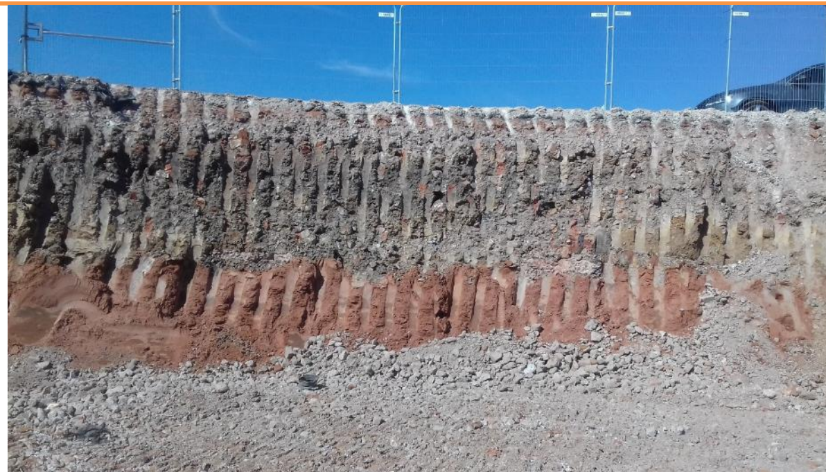
PLATE 10 – WEST SIDE OF SOURCE AREA 1 EXCAVATION
