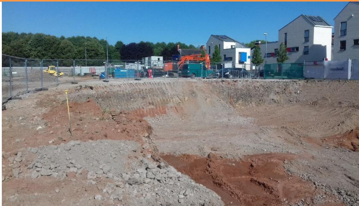
PLATE 7 – WIDE VIEW OF COMPLETED SOURCE AREA 1 EXCAVATION
