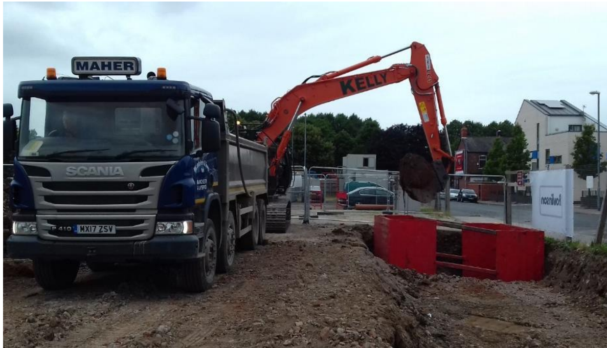
PLATE 1 – EXCAVATION OF SOURCE AREA 1
