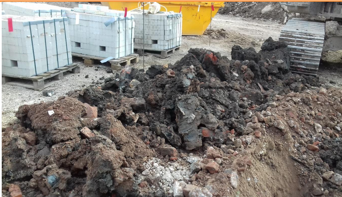
PLATE 26 – ARISINGS OF PRELIMINARY TRIAL PITS
