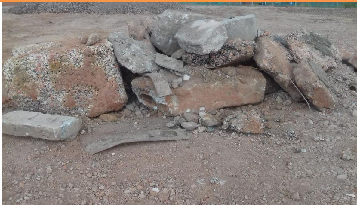
PLATE 23 – UNDERGROUND OBSTRUCTIONS FROM SOURCE AREA 1
