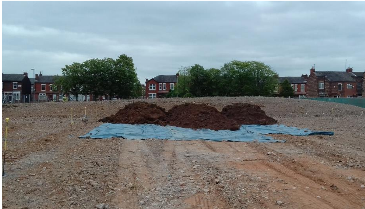
PLATE 3 – STOCKPILING OF EXCAVATED MATERIAL FROM SOURCE AREA 1
