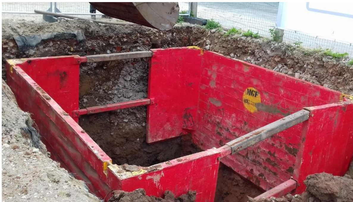
PLATE 2 – BATTERING OF SOURCE AREA 1 EXCAVATION AGAINST ADJACENT HIGHWAY
