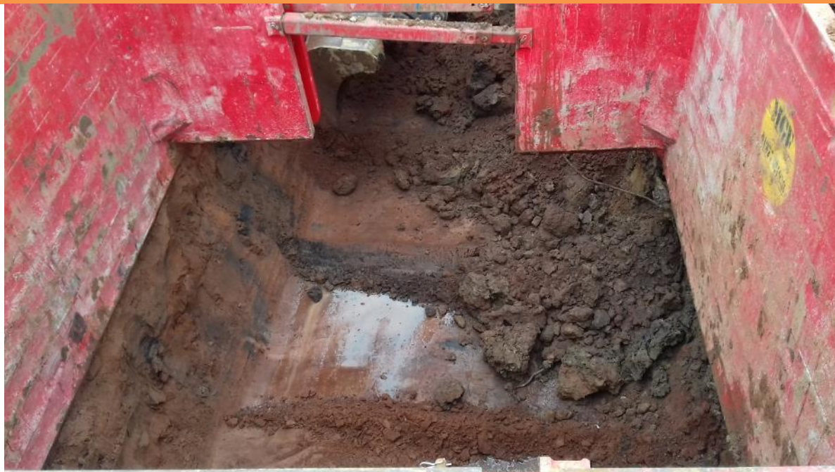
PLATE 5 – BASE OF SOURCE AREA 1 AFTER EXCAVATION
