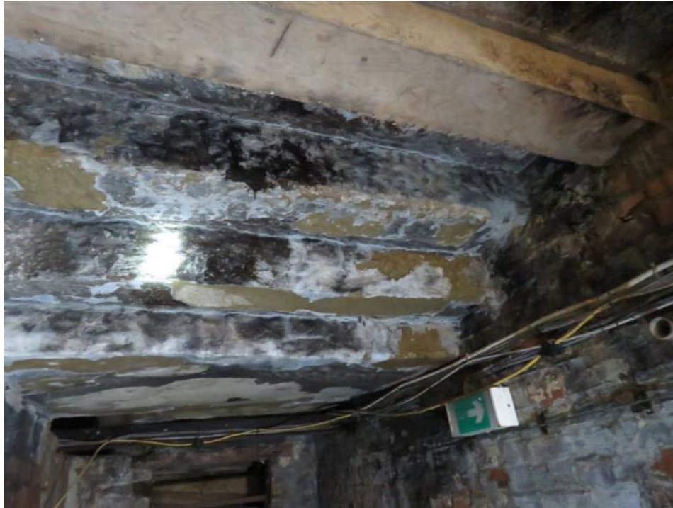
Figure 118: Room B15/B36 (looking west) – The underside of stone steps leading from the rear of the house to the west, onto Crown Street, and now blocked and floored over. (Source: SLHA 2017)
