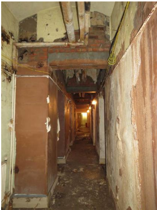
Figure 107: Room G25 (looking south) – This view looks south along the central ground floor corridor, showing the substantial alterations to the lintels and walls undertaken in 1977. (Source: SLHA 2017).
