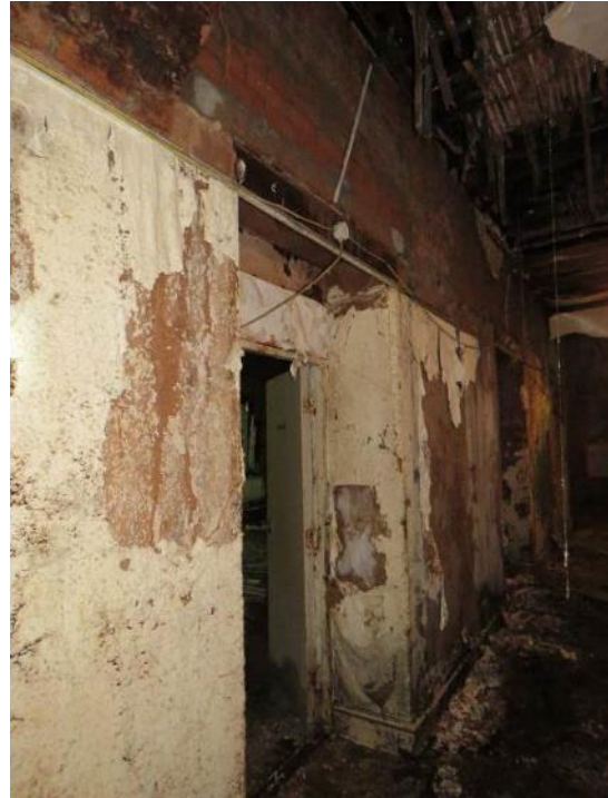
Figure 114: Looking north along the central corridor (Room F13) showing the 1977 alterations and water damage. (Source: SLHA 2017)
