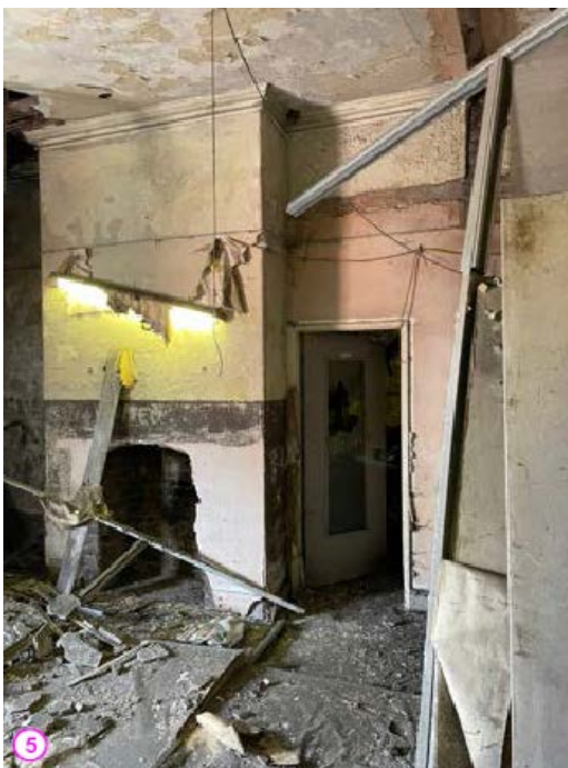
Figure 114a: Looking south-west to the corner of Room F04 in 2022, showing the partial survival of original lath and plaster ceiling and deep cornice. (Source: Snook Architects 2022).
