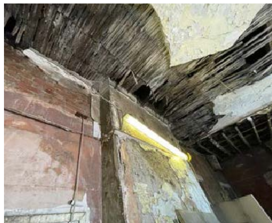
Figure 114: Looking north along the central corridor (Room F13) showing the 1977 alterations and water damage. (Source: SLHA 2017)
