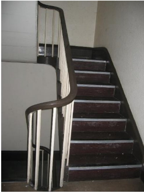
Figure 109: The original stone staircase to the south of the building (G21) (Source: SLHA 2007).
