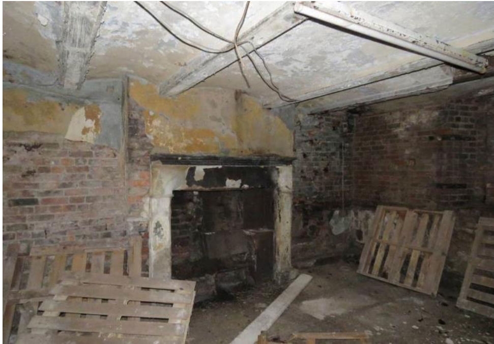
Figure 115: Room B24 (looking north) – The original kitchen of the office building, which retains its original kitchen range and stone surround. Note the exposed and plastered jack-arched ceiling. (Source: SLHA 2017)
