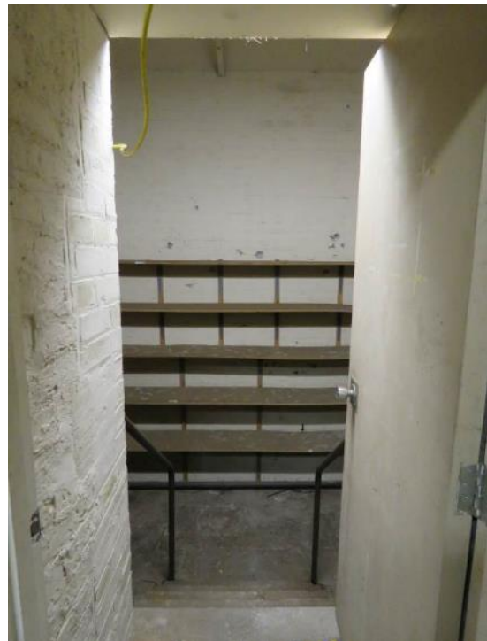
Figure 108: Room G28 - Looking into the 1847 Bridgewater Company strong room (Source: SLHA 2017).
