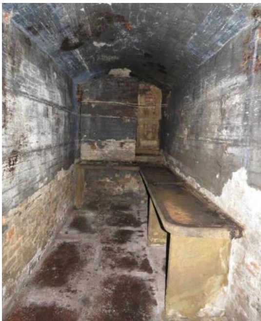
Figure 116: Room B22 (looking east) – The 1842-3 cold store for the adjoining kitchen in Room B24. Note the cold shelf and small stone window surround which looked out into a lightwell on the east elevation. (Source: SLHA 2017)
