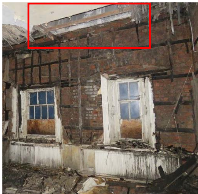
Figure 111 & 112: Room F10 (looking west) - showing the original window shutters in 2007, and the same view in 2017 following substantial loss of plaster surfaces and joinery. The area outlined appears to be an original skylight, which has become revealed following the ceiling collapse. (Source: SLHA 2007 & 2017)
