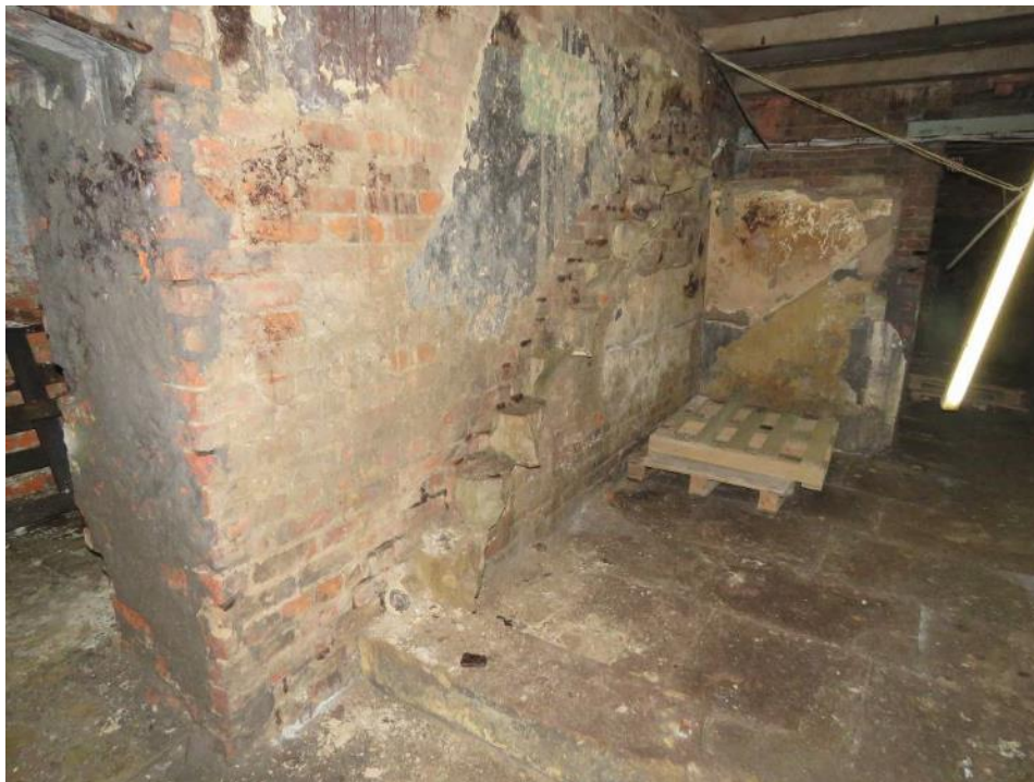
Figure 119: Room B17 (looking east) – The remains of the 1842-3 stone cantilevered office steps from basement floor to the northern ground floor entrance on Crown Street, which were removed in 1977. (Source: SLHA 2017)
