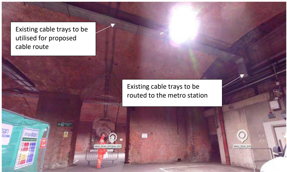
Figure 8: Existing Undercroft area
