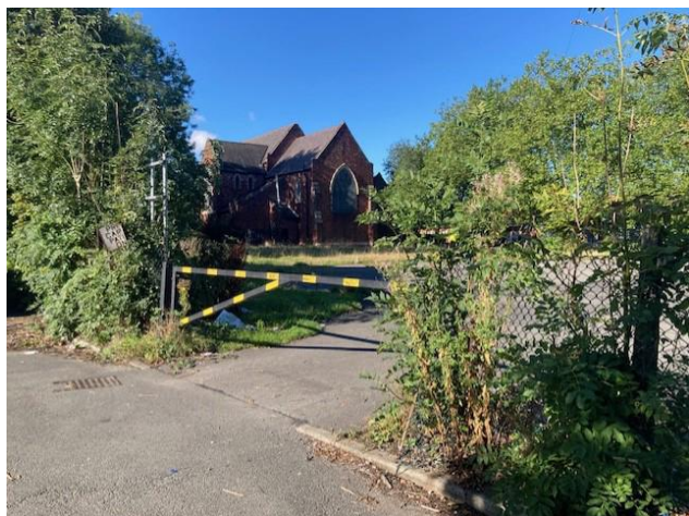
View from the terminus of Sulby Street with rear of St. Luke's Church to south-west
