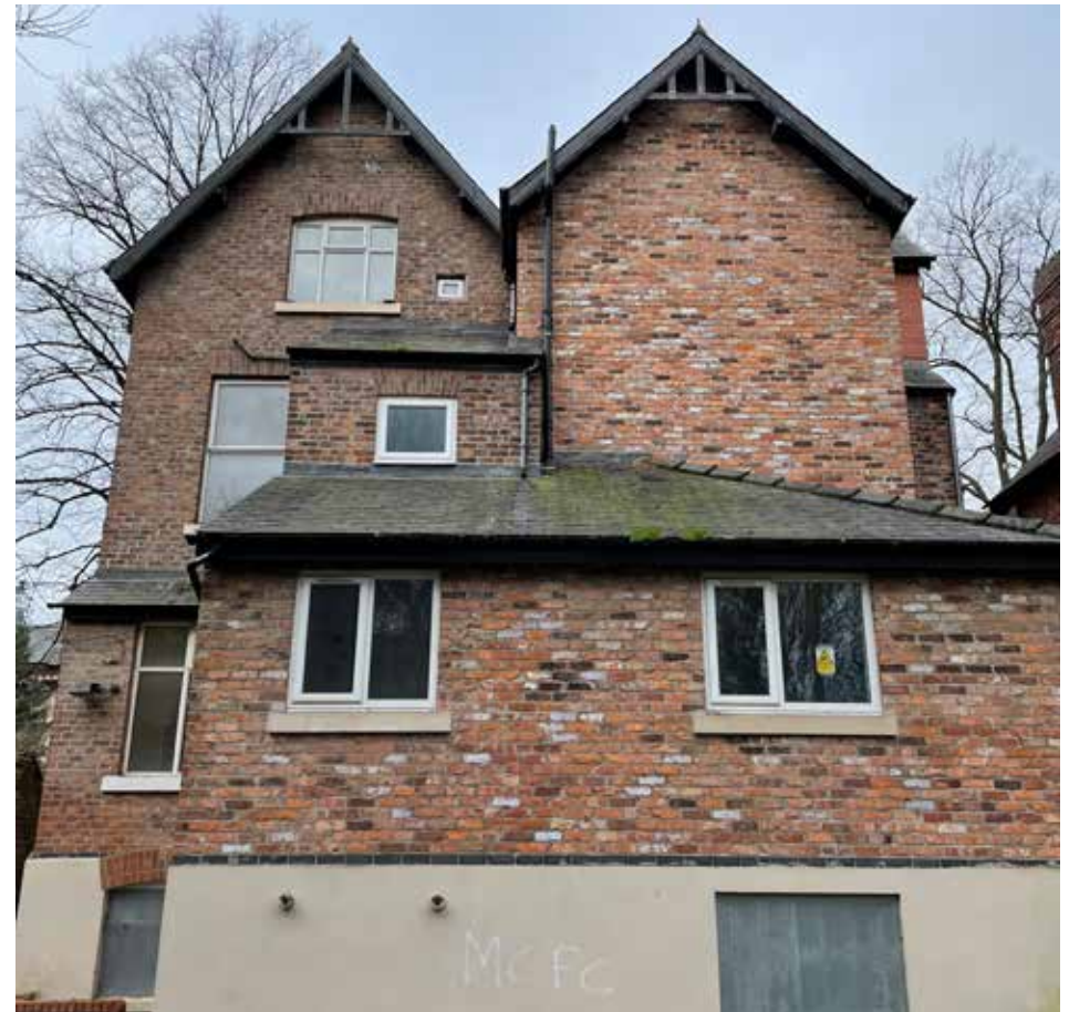
4.1 Existing view of rear elevation
