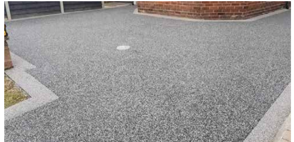
5.7 'Alpine' resin bonded hardstanding
