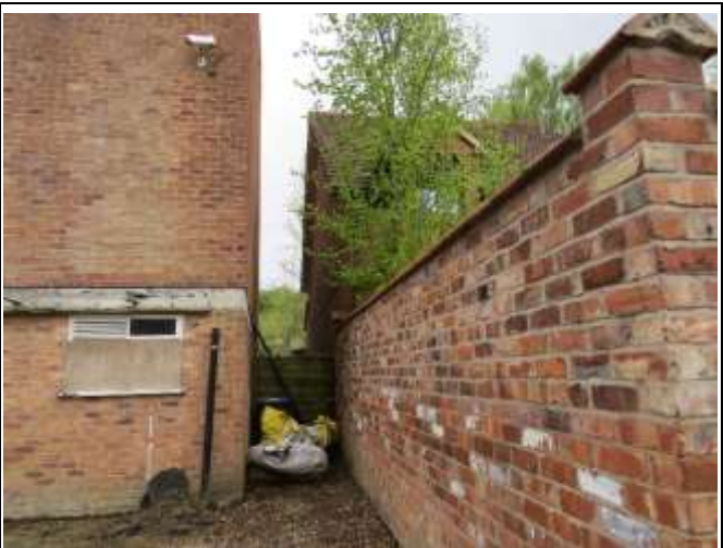
South Boundary to 5A Parkfield Road South
