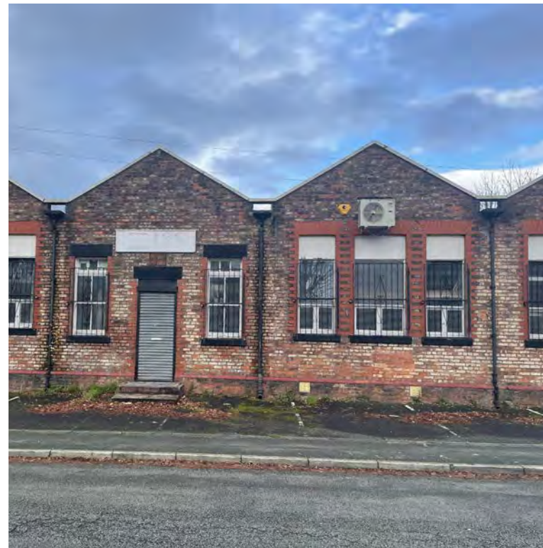
Francis Road, central elevation view of the existing industrial building.
