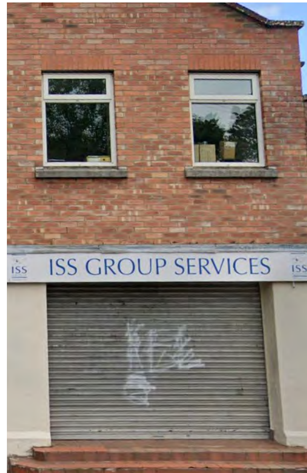
Red brick with feature soldier course and feature render (Existing building on-site)
