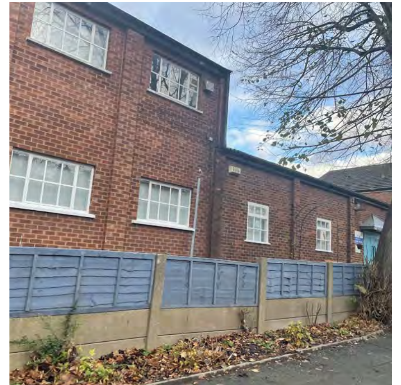
Francis Road, Kingslea House next door to the site.
