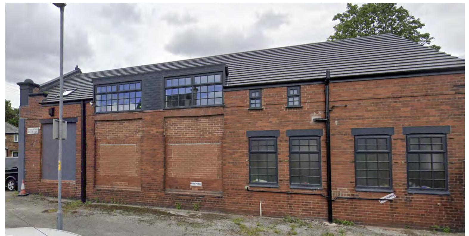
2- Commercial building opposite site
