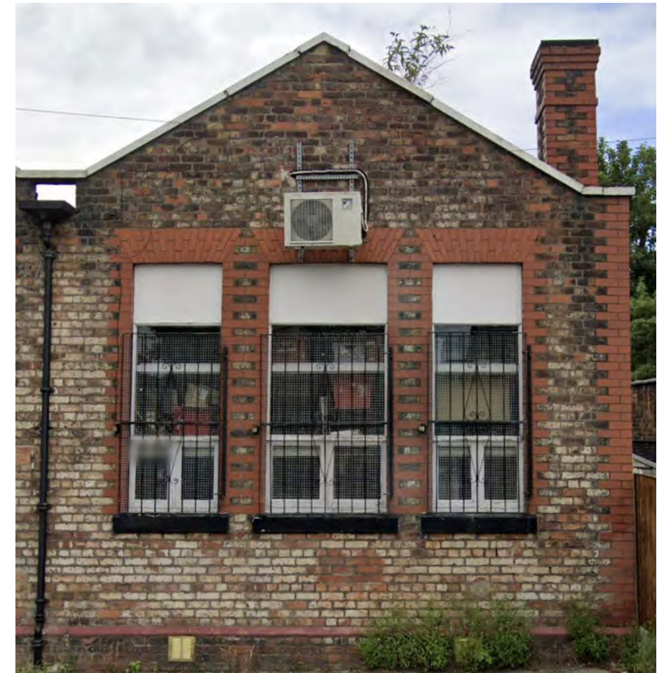
Feature brick details (Existing building on-site)
