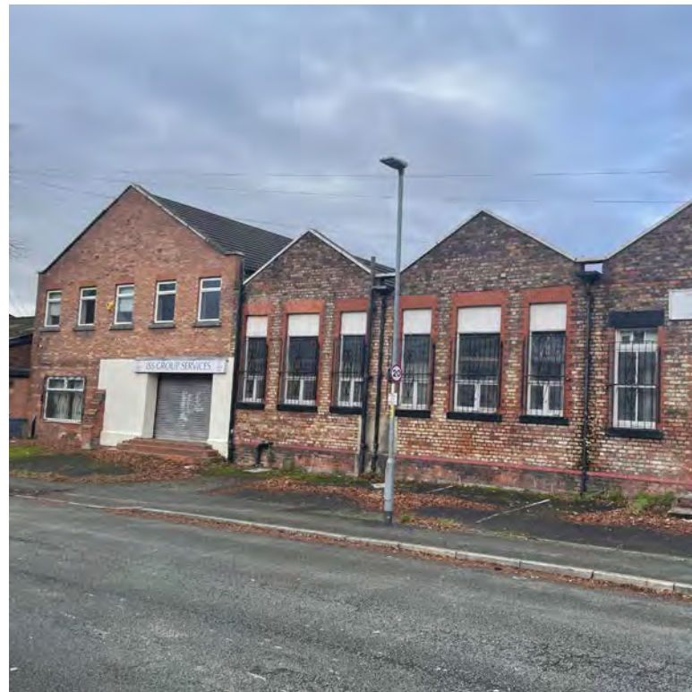
Francis Road, elevation view towards the South West end of the existing industrial building.
