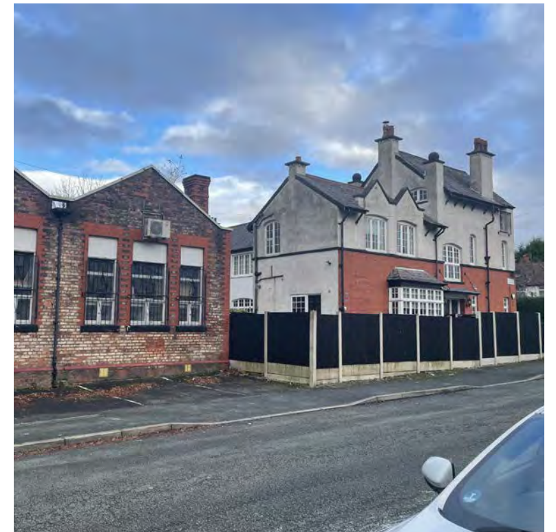
Francis Road, view towards the North East end of the existing industrial building and its abutment with 30 Cotton Lane.
