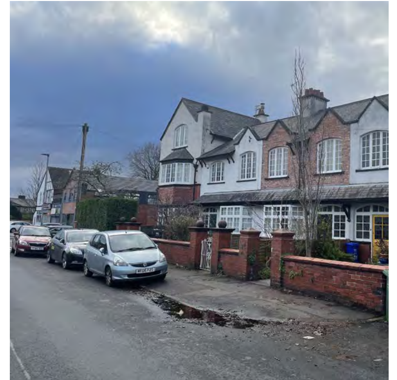
Cotton Lane, taller end terrace building turns corner into Francis Road.
