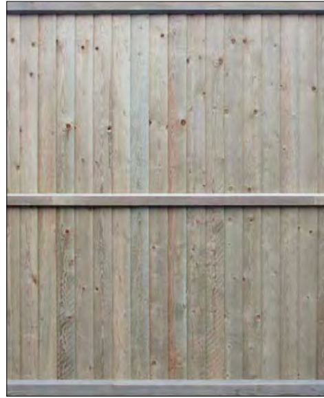
Close boarded fence to secure boundary
