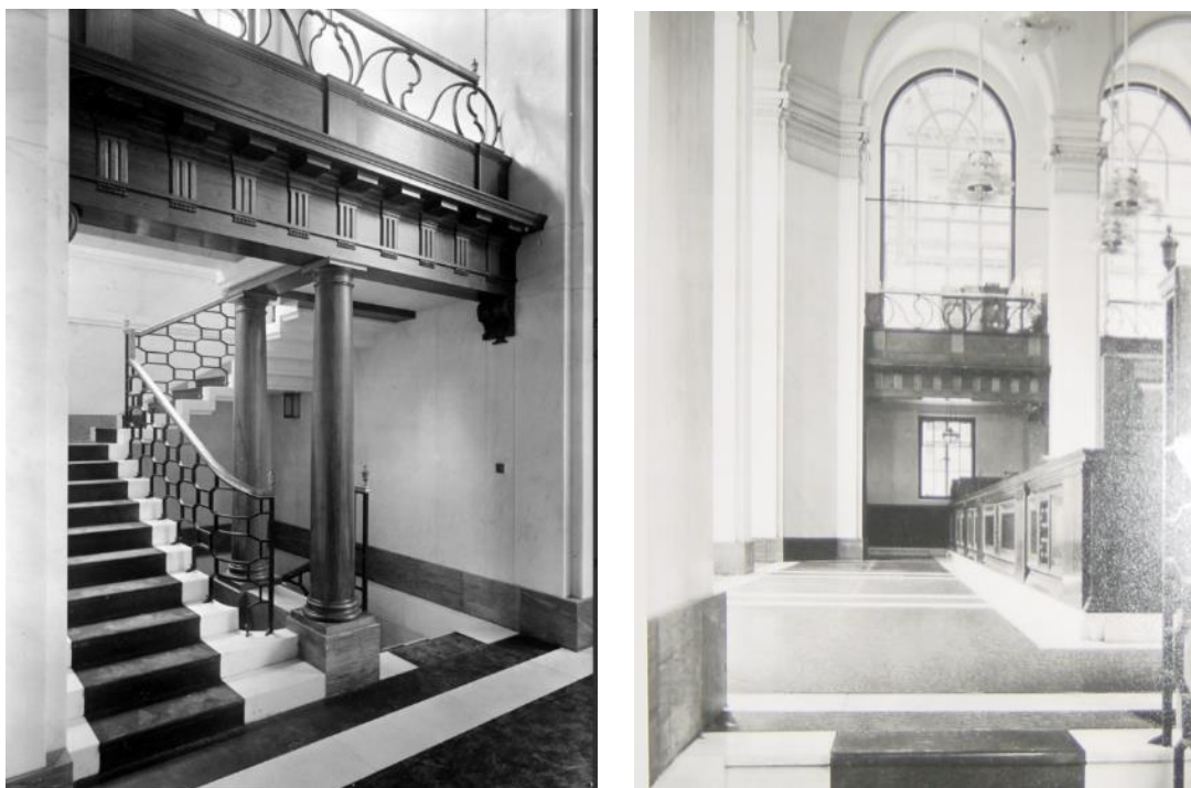
Figure 11 – 1935 photograph of stair and undated photograph of banking hall showing original location of the banking desks. The desks historically align with the column in between the flights of stairs.
