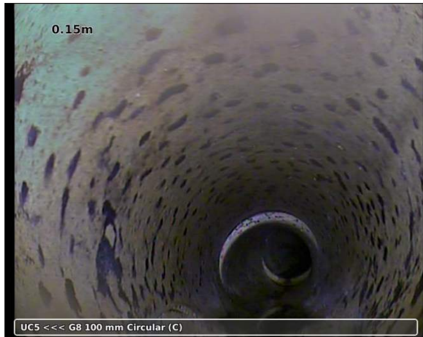
Photo: 20181204-150307-snap0001.jpg 0.15m, Junction from/at 05 o'clock to 07 o'clock diameter: 100 mm
