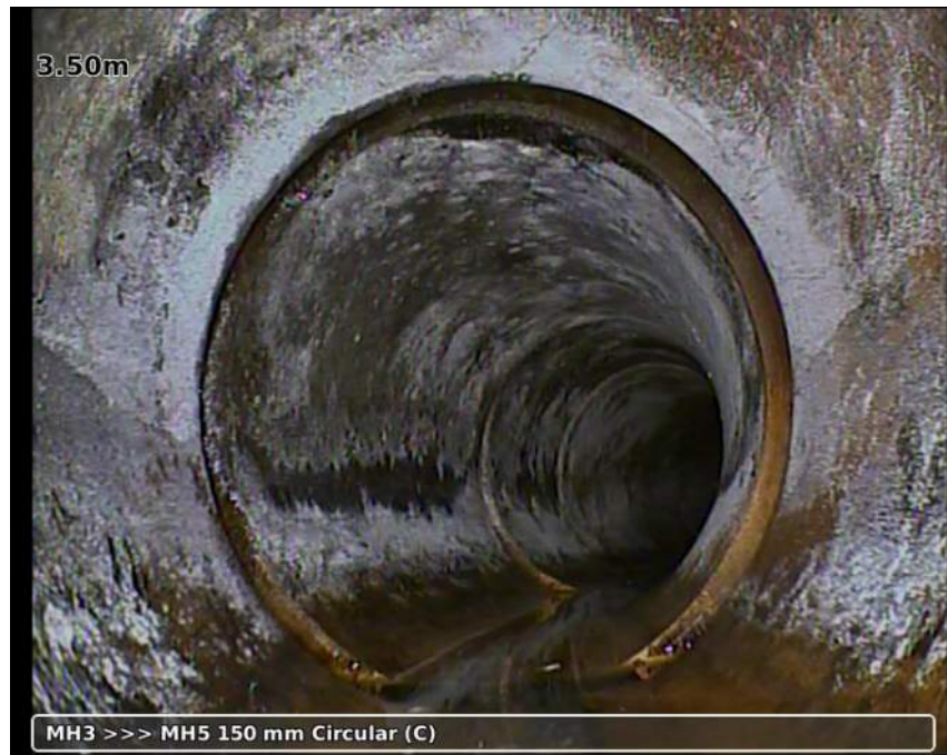
Photo: 20181122-114728-snap0001.jpg 3.5m, Line deviates right
