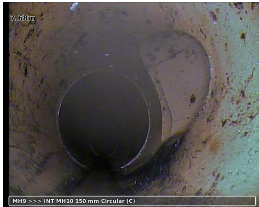
Photo: 20181123-111344-snap0001.jpg 7.68m, Junction from/at 03 o'clock diameter: 100 mm
