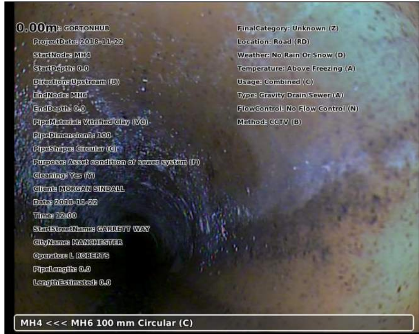
Photo: 20181122-120037-snap0000.jpg 0m, Start node type manhole reference number: MH4
