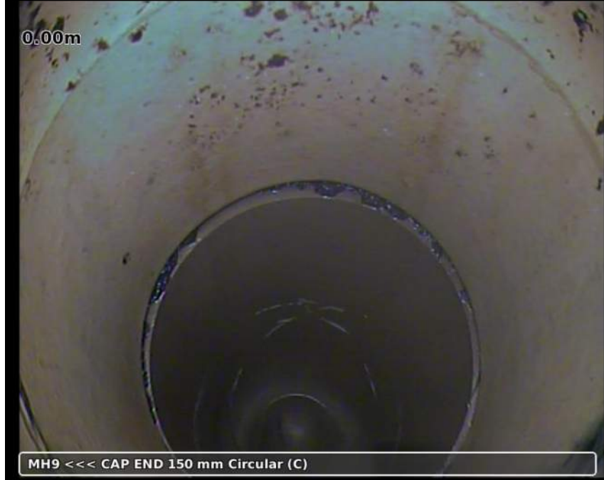
Photo: 20181123-115736-snap0000.jpg 0m, Start node type manhole reference number: MH9
