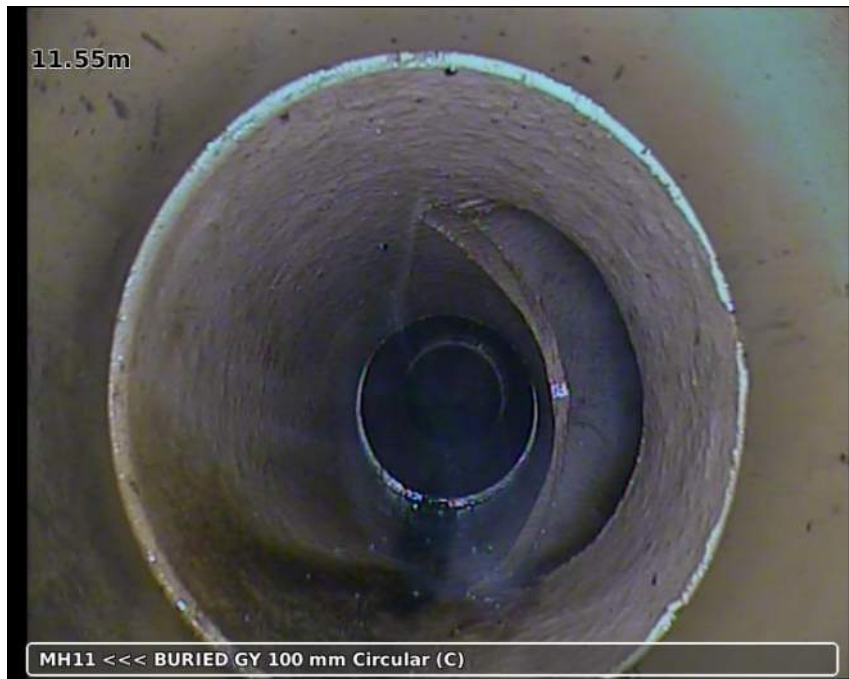
Photo: 20181123-141150-snap0003.jpg 11.55m, Junction from/at 03 o'clock diameter: 100 mm
