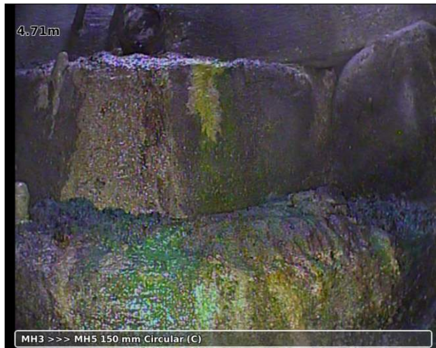
Photo: 20181122-114728-snap0002.jpg 4.71m, Finish node type manhole reference number: MH5
