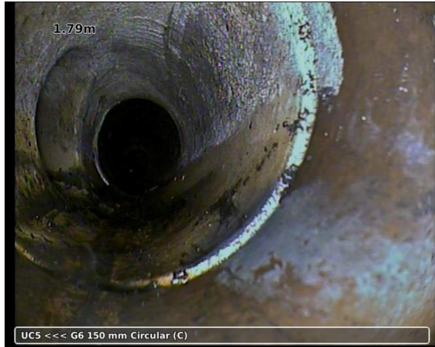
Photo: 20181204-144214-snap0002.jpg 1.79m, Junction from/at 07 o'clock to 10 o'clock diameter: 150 mm
