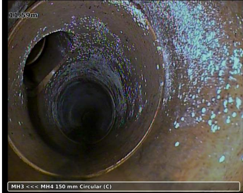
Photo: 20181122-105400-snap0002.jpg 11.59m, Junction from/at 10 o'clock diameter: 100 mm
