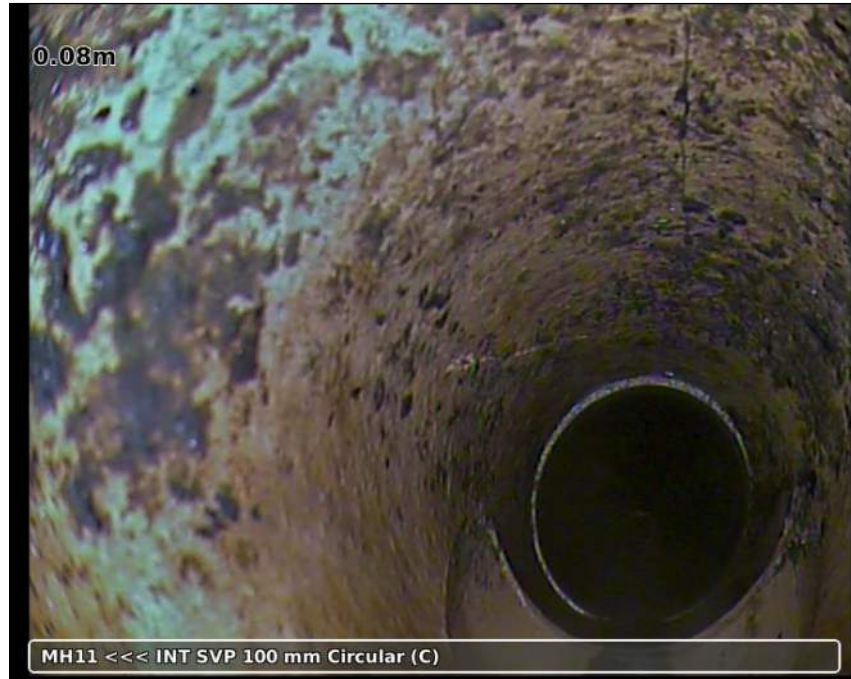
Photo: 20181123-142115-snap0002.jpg 0.08m, Junction from/at 06 o'clock diameter: 100 mm
