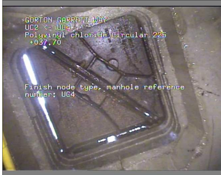
Photo: 10_10_64_A.JPG 37.7m, Finish node type, manhole reference number: UC4
