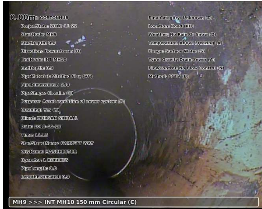
Photo: 20181123-111344-snap0000.jpg 0m, Start node type manhole reference number: MH9
