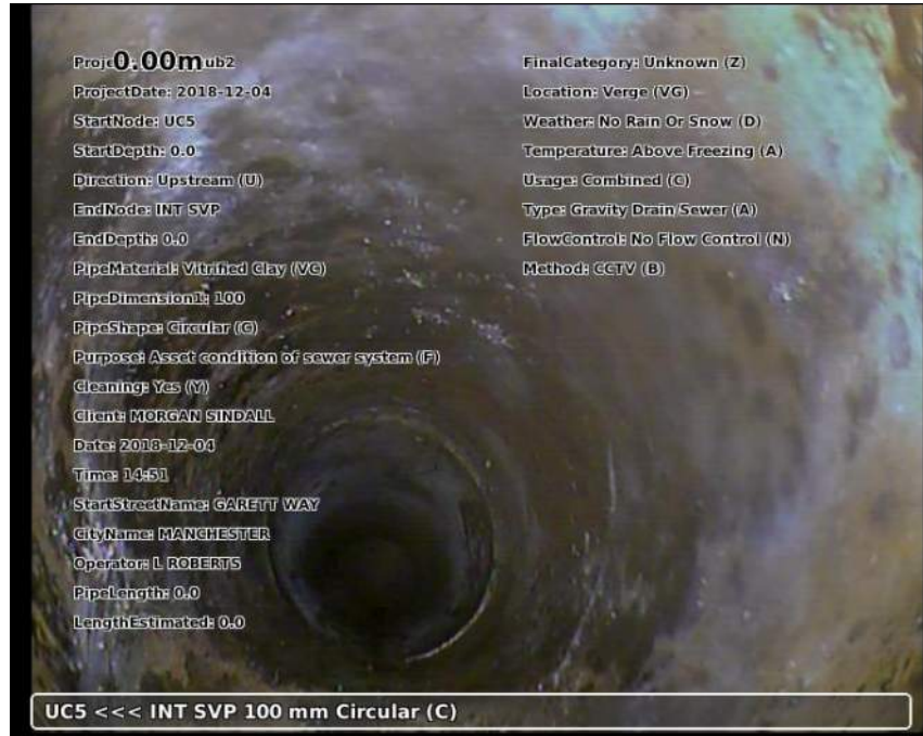
Photo: 20181204-145231-snap0000.jpg 0m, Start node type manhole reference number: UC5
