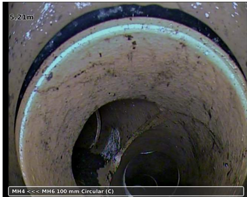
Photo: 20181122-120037-snap0001.jpg 5.21m, Junction from/at 09 o'clock diameter: 100 mm
