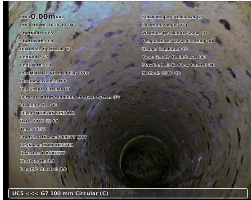
Photo: 20181204-145924-snap0000.jpg 0m, Start node type manhole reference number: UC5
