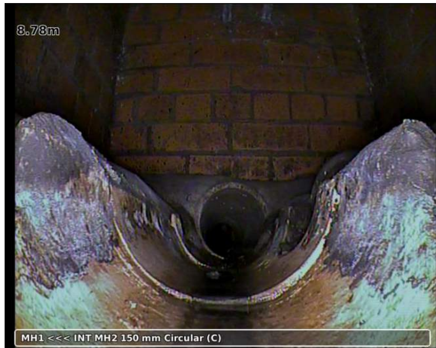
Photo: 20181122-101845-snap0001.jpg 8.78m, Finish node type manhole reference number: INT MH2
