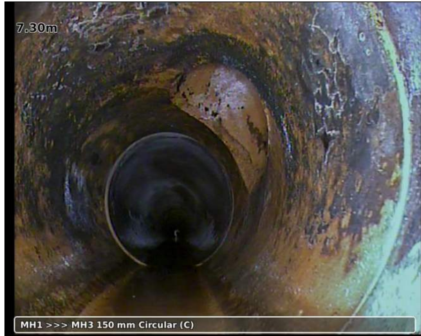
Photo: 20181122-103541-snap0002.jpg 7.3m, Junction from/at 02 o'clock diameter: 100 mm
