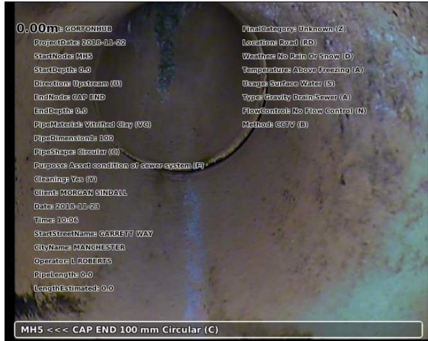
Photo: 20181123-100650-snap0000.jpg 0m, Start node type manhole reference number: MH5
