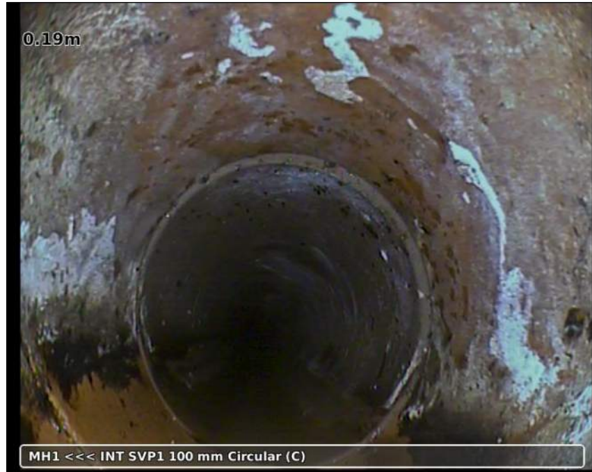
Photo: 20181122-102650-snap0002.jpg 0.19m, Junction from/at 06 o'clock diameter: 100 mm
