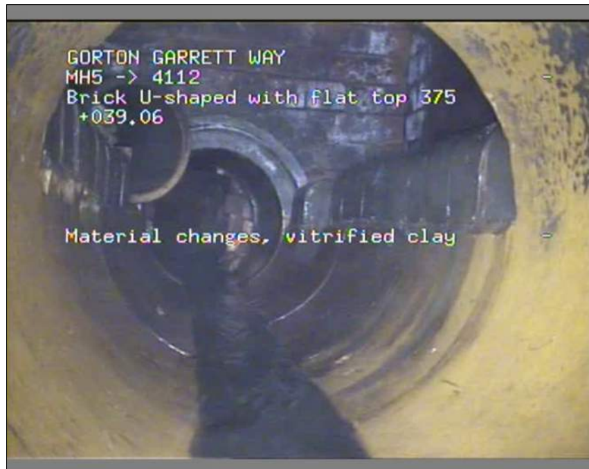
Photo: 4_4_28_A.JPG 39.08m, Material changes, vitrified clay
