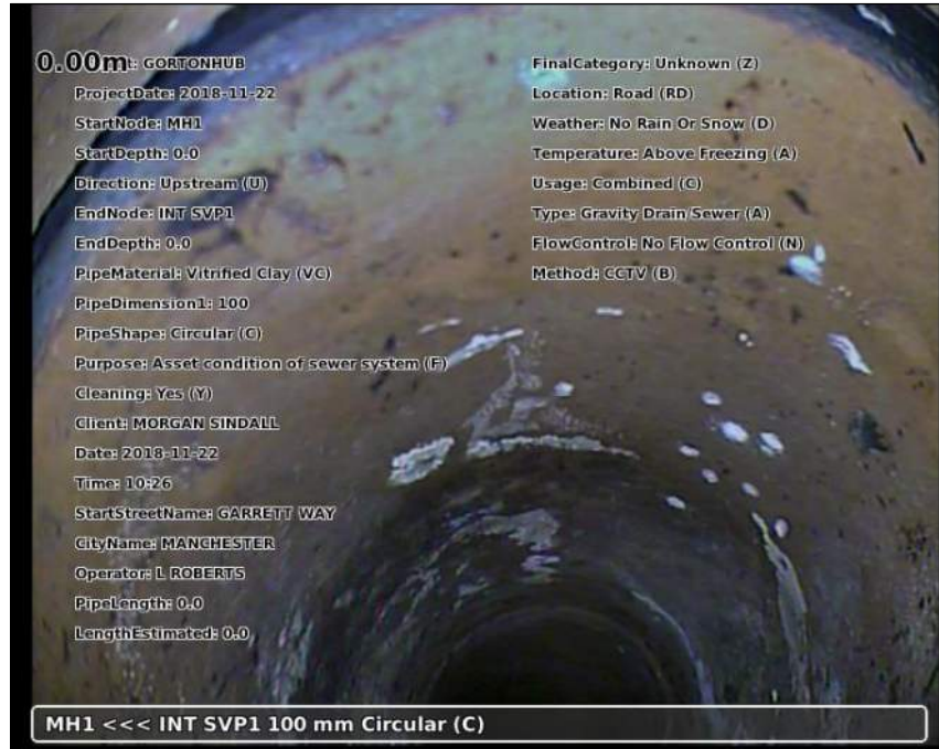
Photo: 20181122-102650-snap0000.jpg 0m, Start node type manhole reference number: MH1
