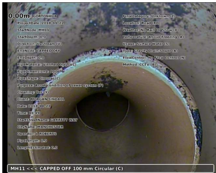
Photo: 20181123-135029-snap0000.jpg 0m, Start node type manhole reference number: MH11
