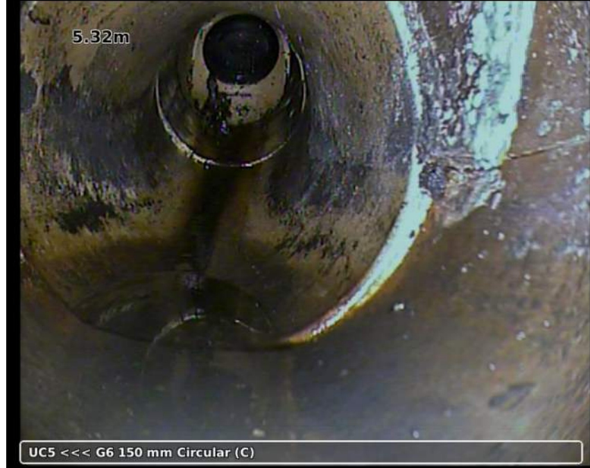
Photo: 20181204-144214-snap0004.jpg 5.32m, Line deviates up M
