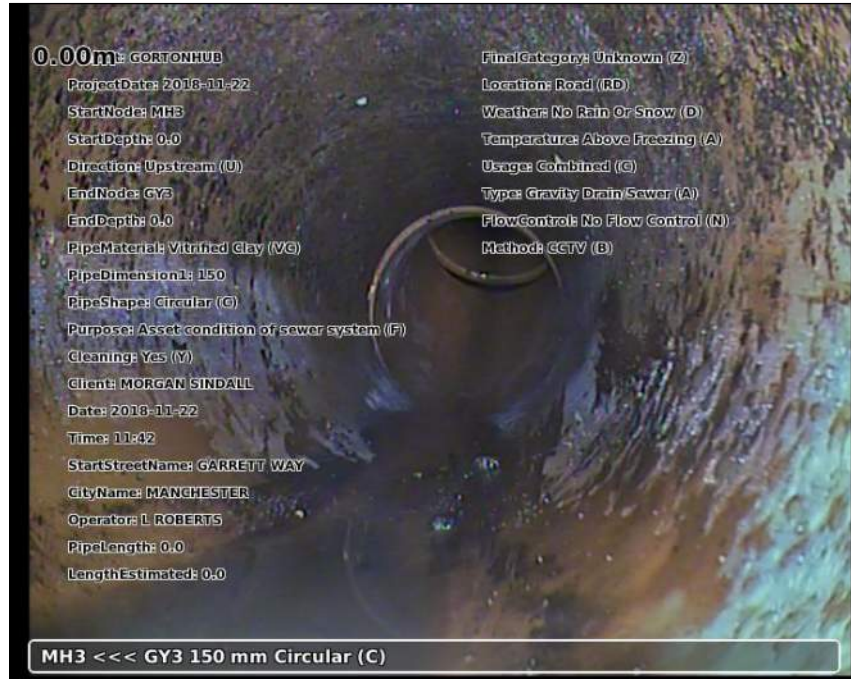
Photo: 20181122-114351-snap0000.jpg 0m, Start node type manhole reference number: MH3
