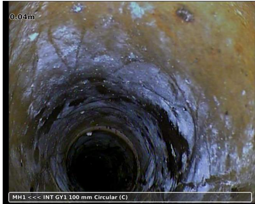
Photo: 20181122-102339-snap0002.jpg 0.04m, Junction from/at 06 o'clock diameter: 100 mm
