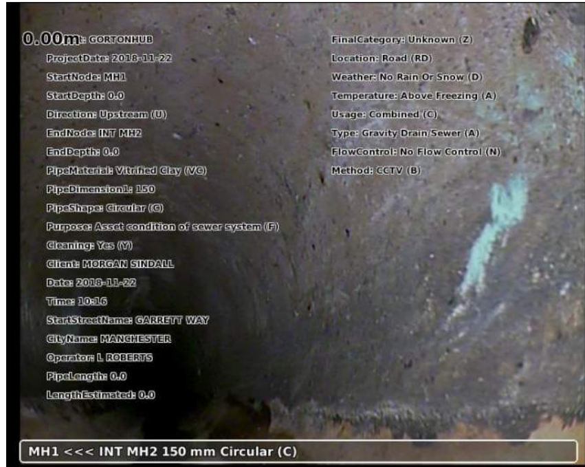
Photo: 20181122-101845-snap0000.jpg 0m, Start node type manhole reference number: MH1
