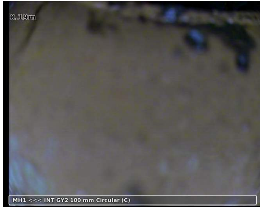
Photo: 20181122-103009-snap0002.jpg 0.19m, Junction from/at 06 o'clock diameter: 100 mm
