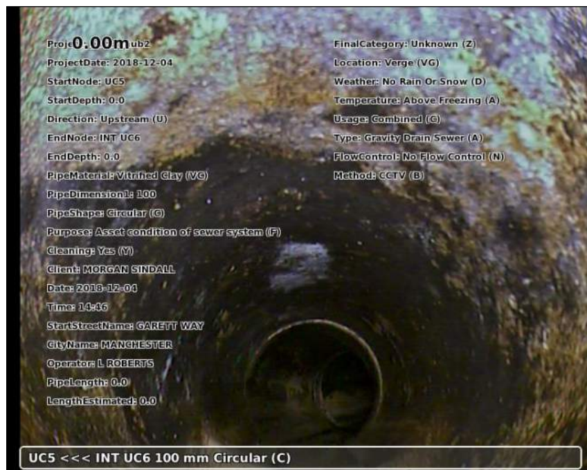
Photo: 20181204-144708-snap0000.jpg 0m, Start node type manhole reference number: UC5
