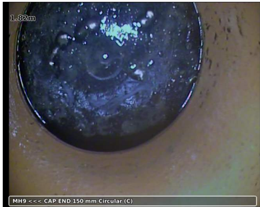
Photo: 20181123-115736-snap0005.jpg 1.82m, Survey abandoned
