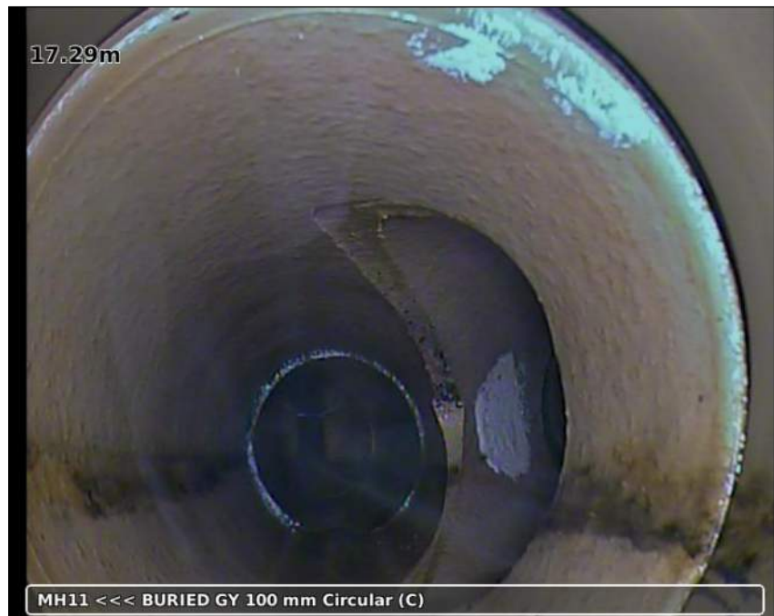
Photo: 20181123-141150-snap0004.jpg 17.29m, Junction from/at 03 o'clock diameter: 100 mm
