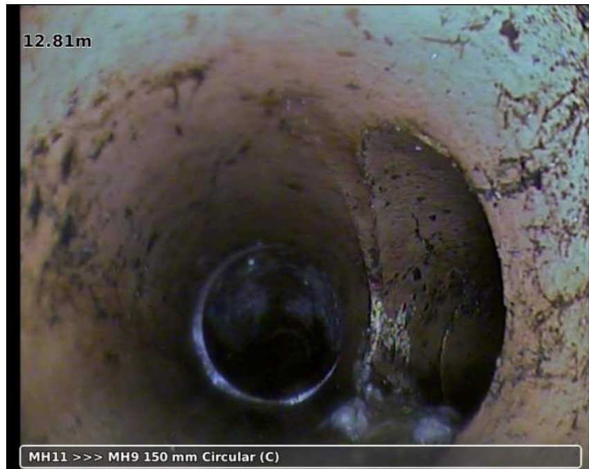
Photo: 20181123-113047-snap0001.jpg 12.81m, Junction from/at 03 o'clock diameter: 100 mm
