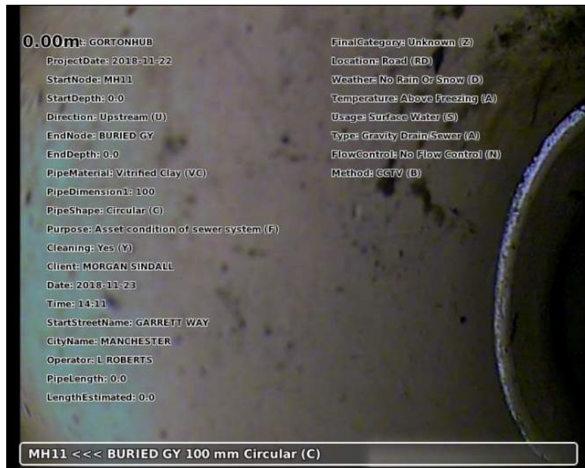
Photo: 20181123-141150-snap0000.jpg 0m, Start node type manhole reference number: MH11
