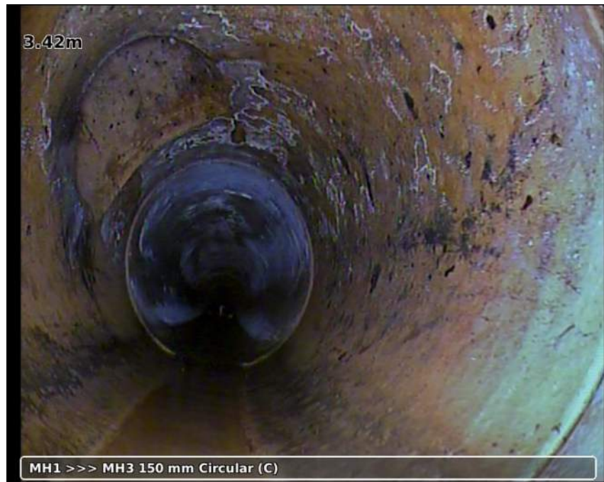
Photo: 20181122-103541-snap0001.jpg 3.42m, Junction from/at 10 o'clock diameter: 100 mm
