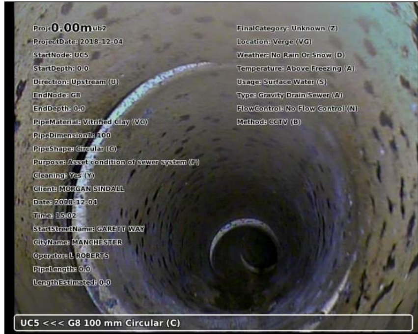
Photo: 20181204-150307-snap0000.jpg 0m, Start node type manhole reference number: UC5
