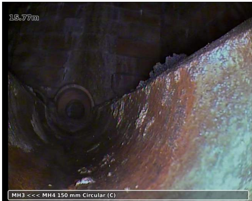
Photo: 20181122-105400-snap0003.jpg 15.77m, Finish node type manhole reference number: MH4
