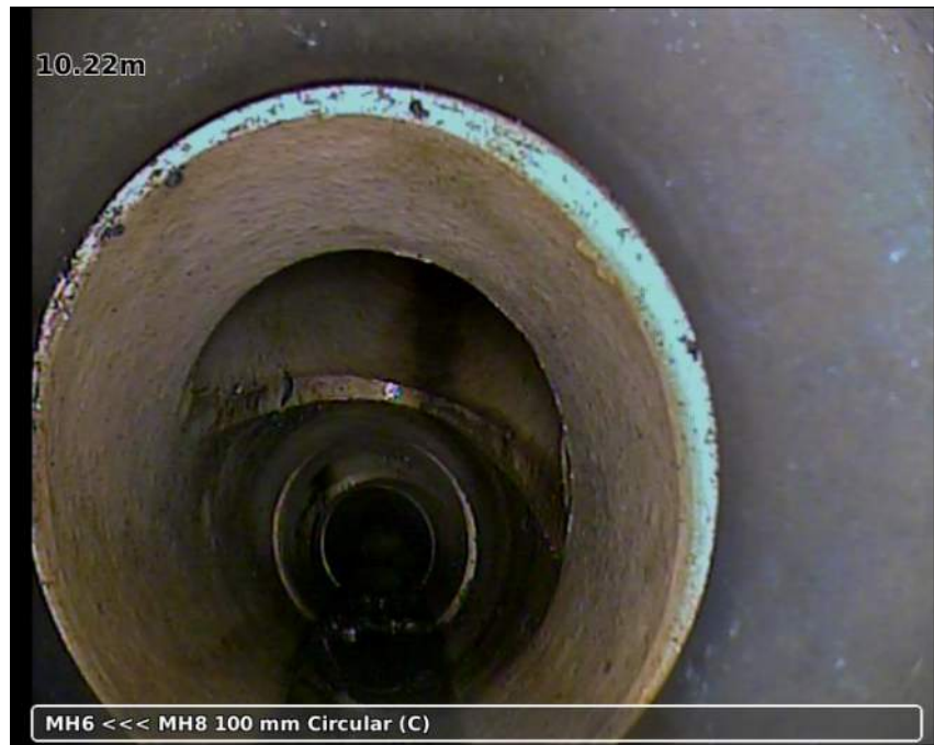
Photo: 20181123-082335-snap0001.jpg 10.22m, Junction from/at 01 o'clock diameter: 100 mm
