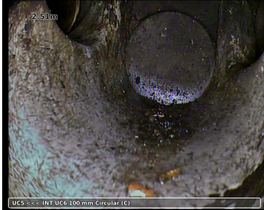
Photo: 20181204-144708-snap0002.jpg 2.51m, Finish node type manhole reference number: INT UC6
