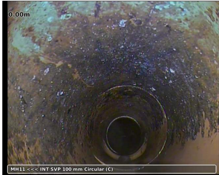
Photo: 20181123-142115-snap0000.jpg 0m, Start node type manhole reference number: MH11
