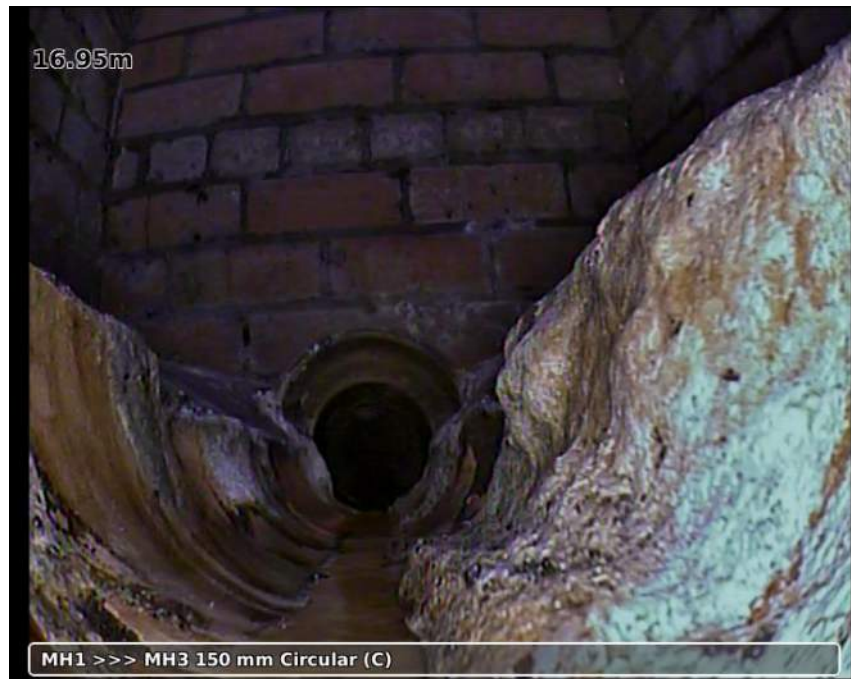
Photo: 20181122-103541-snap0003.jpg 16.95m, Finish node type manhole reference number: MH3
