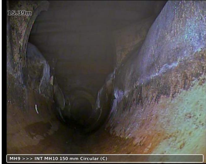
Photo: 20181123-111344-snap0002.jpg 15.39m, Finish node type manhole reference number: INT MH10
