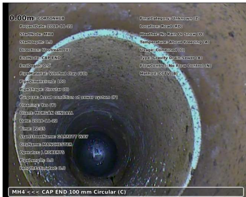
Photo: 20181122-120552-snap0000.jpg 0m, Start node type manhole reference number: MH4
