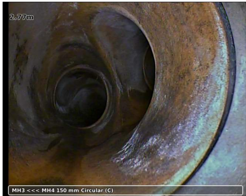
Photo: 20181122-105400-snap0001.jpg 2.77m, Junction from/at 03 o'clock diameter: 150 mm
