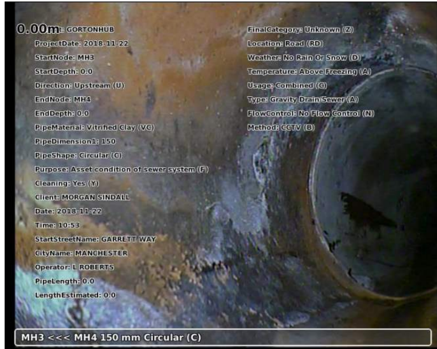
Photo: 20181122-105400-snap0000.jpg 0m, Start node type manhole reference number: MH3
