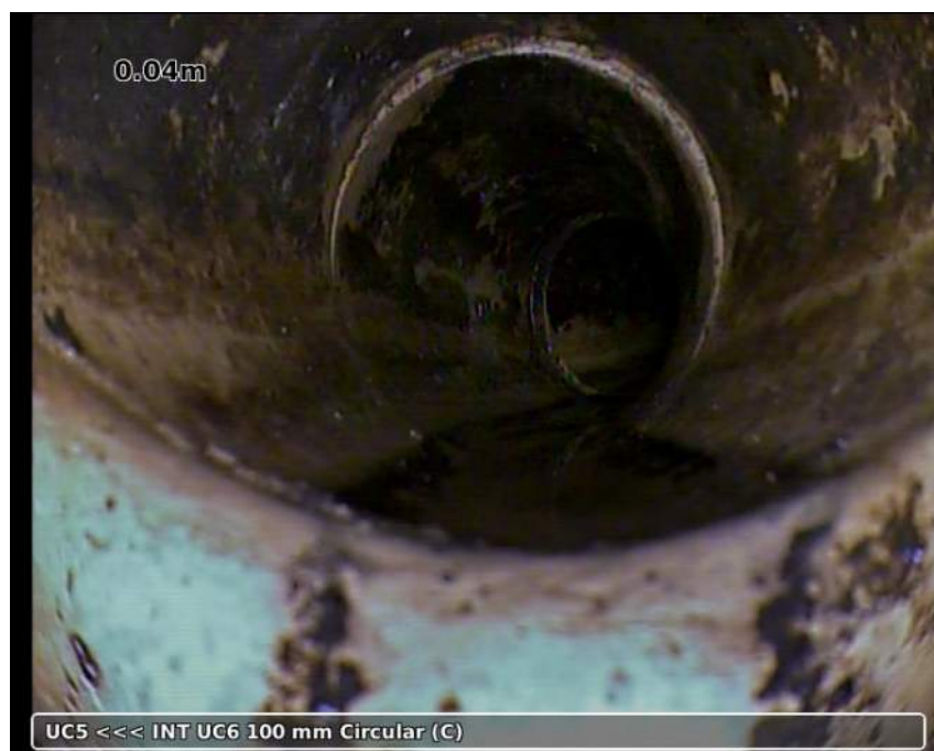
Photo: 20181204-144708-snap0001.jpg 0.04m, Junction from/at 05 o'clock to 07 o'clock diameter: 100 mm
