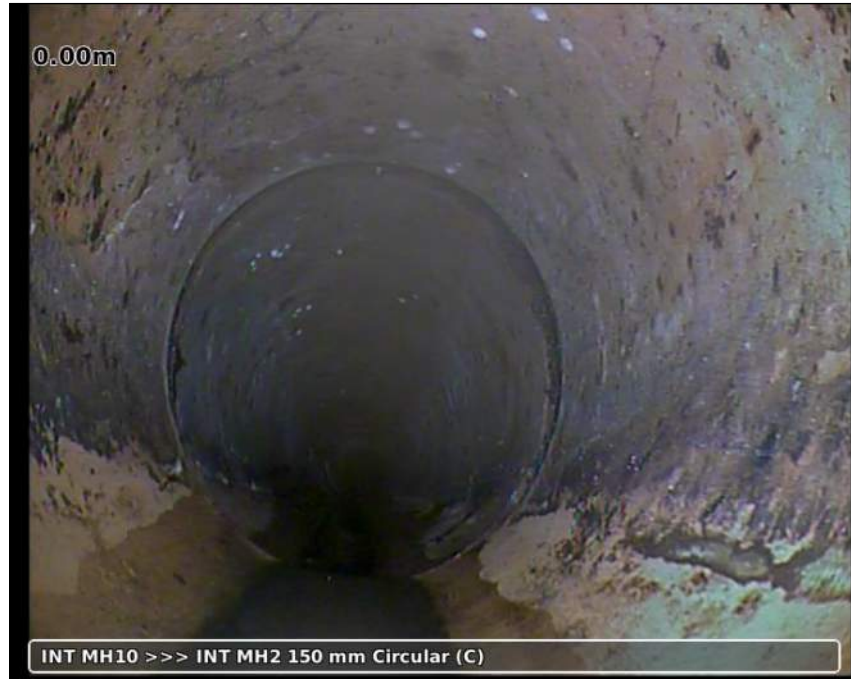
Photo: 20181123-111622-snap0000.jpg 0m, Start node type manhole reference number: INT MH10
