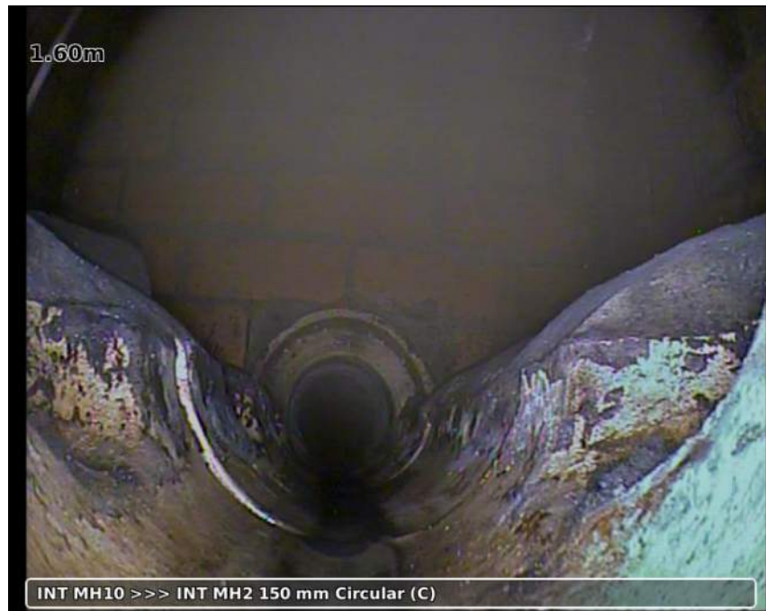
Photo: 20181123-111622-snap0001.jpg 1.6m, Finish node type manhole reference number: INT MH2
