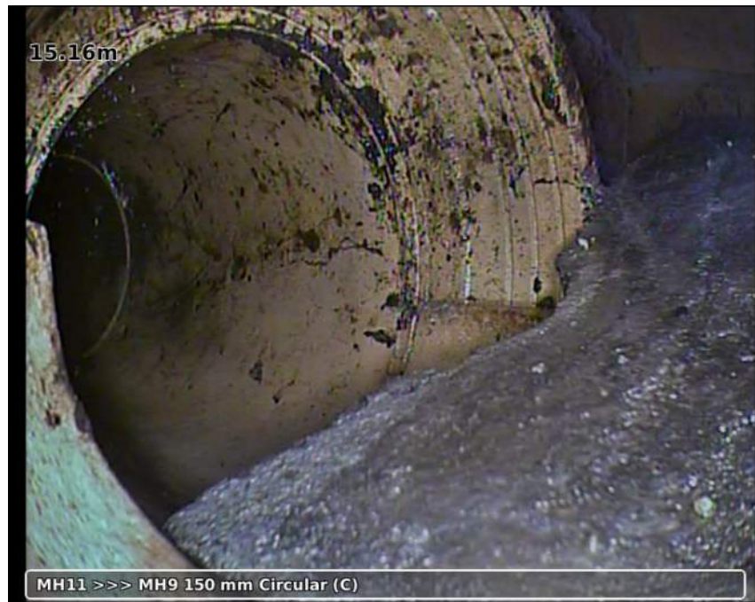
Photo: 20181123-113047-snap0003.jpg 15.16m, Finish node type manhole reference number: MH9
