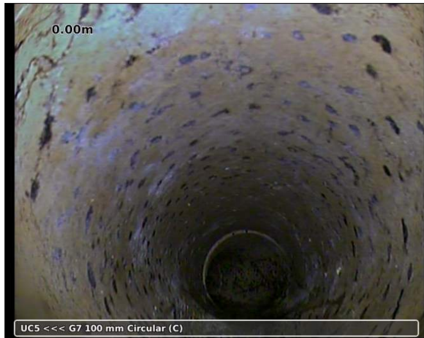
Photo: 20181204-145924-snap0001.jpg 0m, Junction from/at 05 o'clock to 07 o'clock diameter: 100 mm
