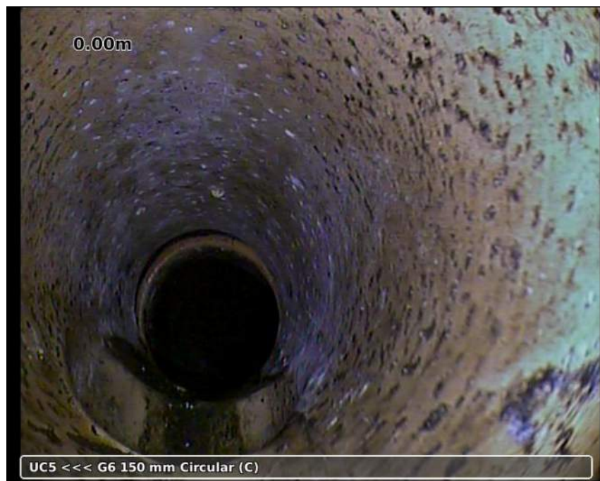
Photo: 20181204-144214-snap0001.jpg 0m, Junction from/at 05 o'clock to 07 o'clock diameter: 150 mm
