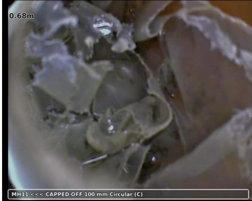
Photo: 20181123-135029-snap0004.jpg 0.68m, Survey abandoned
