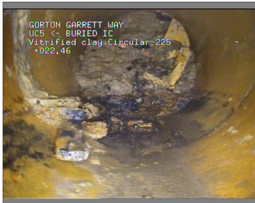
Photo: 13_13_82_A.JPG 22.46m, Finish node type, inspection chamber reference number: BURIED IC
