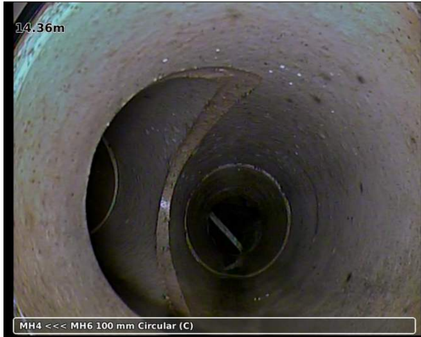
Photo: 20181122-120037-snap0002.jpg 14.36m, Junction from/at 09 o'clock diameter: 100 mm
