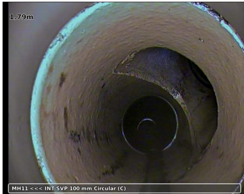
Photo: 20181123-142115-snap0003.jpg 1.79m, Junction from/at 03 o'clock diameter: 100 mm
