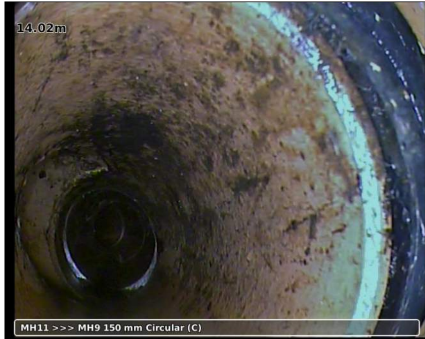
Photo: 20181123-113047-snap0002.jpg 14.02m, Junction from/at 09 o'clock diameter: 100 mm
