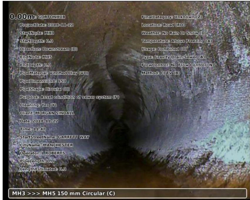
Photo: 20181122-114728-snap0000.jpg 0m, Start node type manhole reference number: MH3
