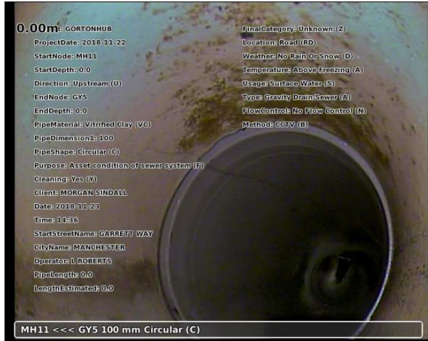
Photo: 20181123-144743-snap0000.jpg 0m, Start node type manhole reference number: MH11
