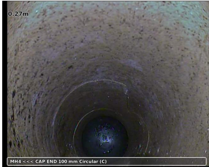
Photo: 20181122-120552-snap0002.jpg 0.27m, Junction from/at 06 o'clock diameter: 100 mm
