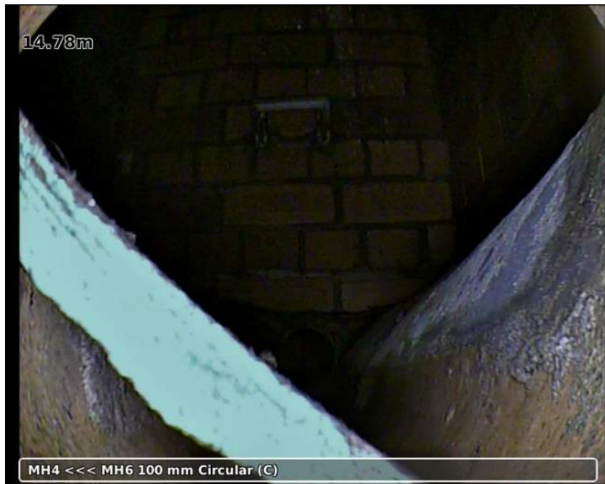
Photo: 20181122-120037-snap0003.jpg 14.78m, Finish node type manhole reference number: MH6
