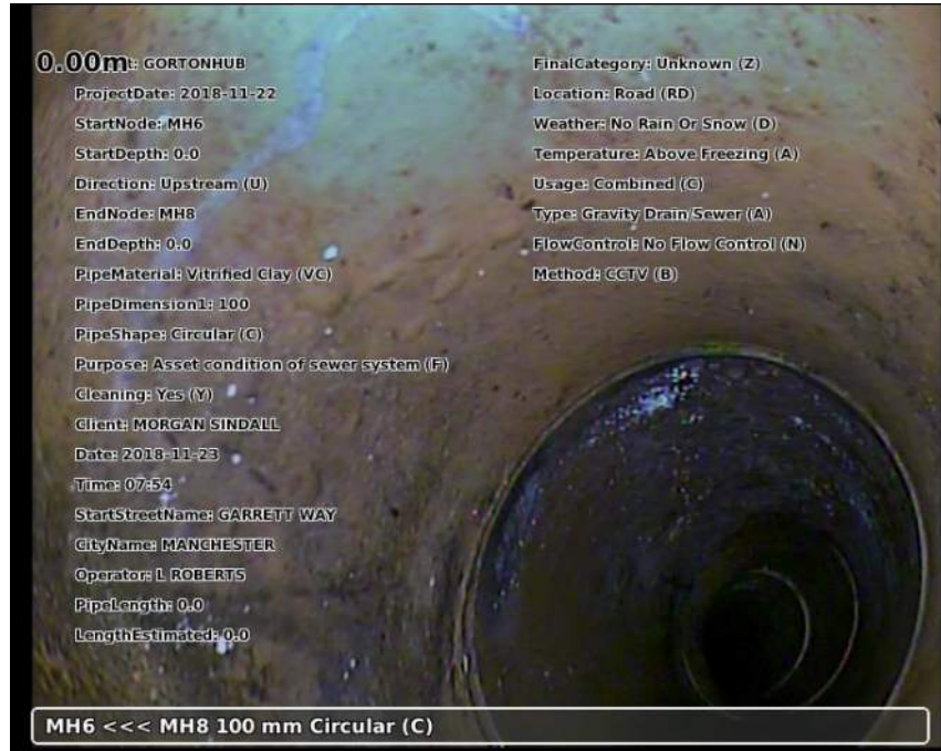
Photo: 20181123-082335-snap0000.jpg 0m, Start node type manhole reference number: MH6
