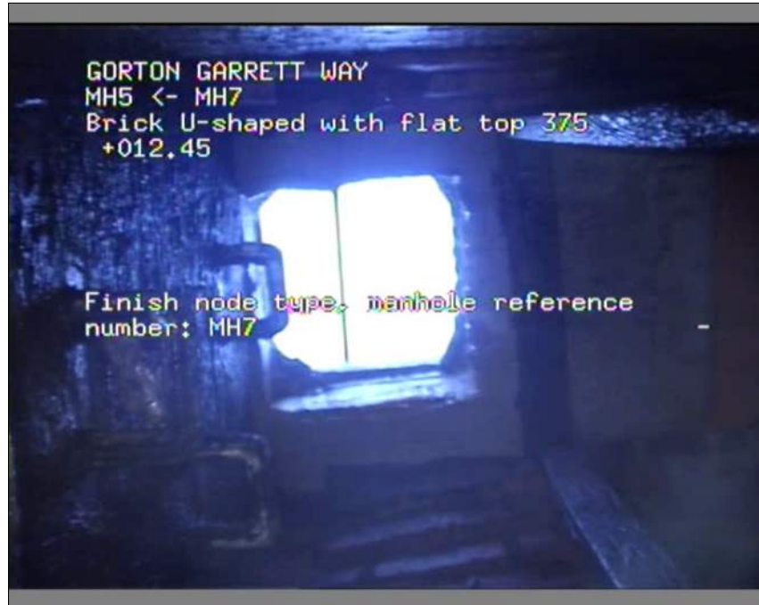
Photo: 1_1_13_A.JPG 12.45m, Finish node type, manhole reference number: MH7
