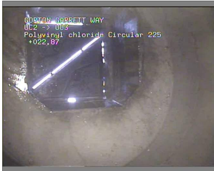
Photo: 9_9_57_A.JPG 22.87m, Finish node type, manhole reference number: UC3
