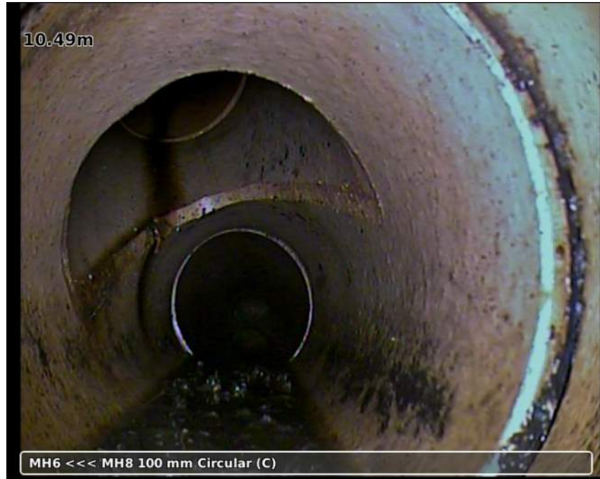
Photo: 20181123-082335-snap0002.jpg 10.49m, Junction from/at 11 o'clock diameter: 100 mm
