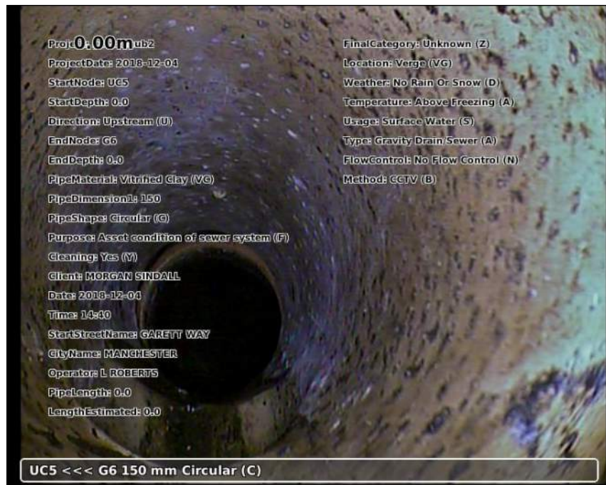
Photo: 20181204-144214-snap0000.jpg 0m, Start node type manhole reference number: UC5
