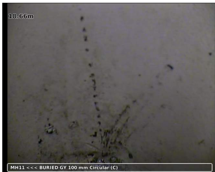
Photo: 20181123-141150-snap0005.jpg 18.66m, Finish node type gully reference number: BURIED GY
