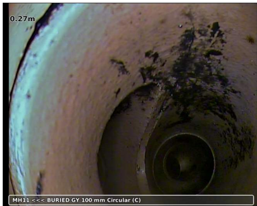
Photo: 20181123-141150-snap0001.jpg 0.27m, Junction from/at 09 o'clock diameter: 100 mm
