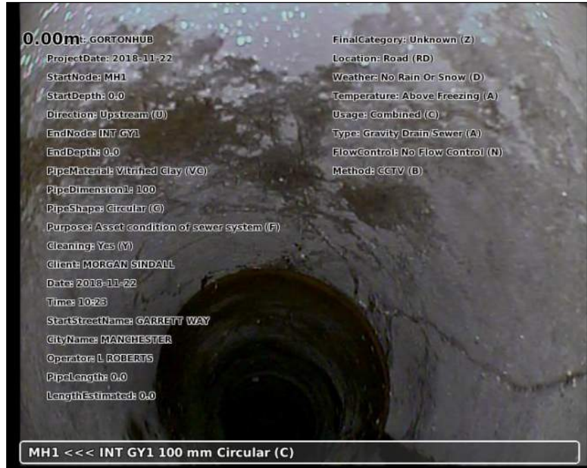
Photo: 20181122-102339-snap0000.jpg 0m, Start node type manhole reference number: MH1
