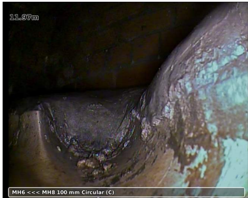
Photo: 20181123-082335-snap0003.jpg 11.93m, Finish node type manhole reference number: MH8
