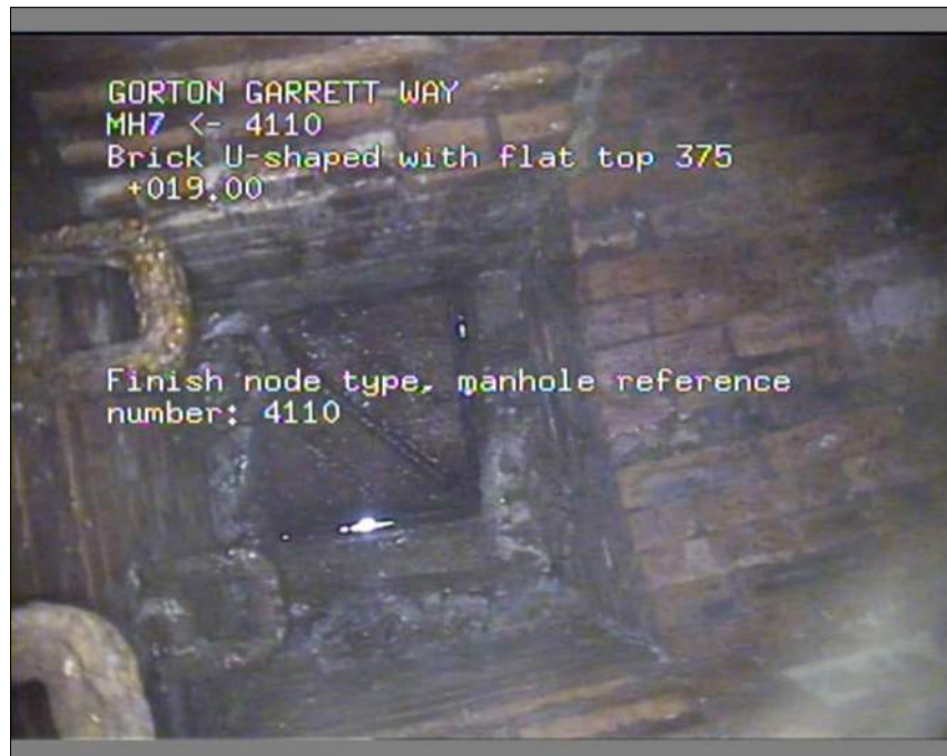
Photo: 3_3_20_A.JPG 19m, Finish node type, manhole reference number: 4110
