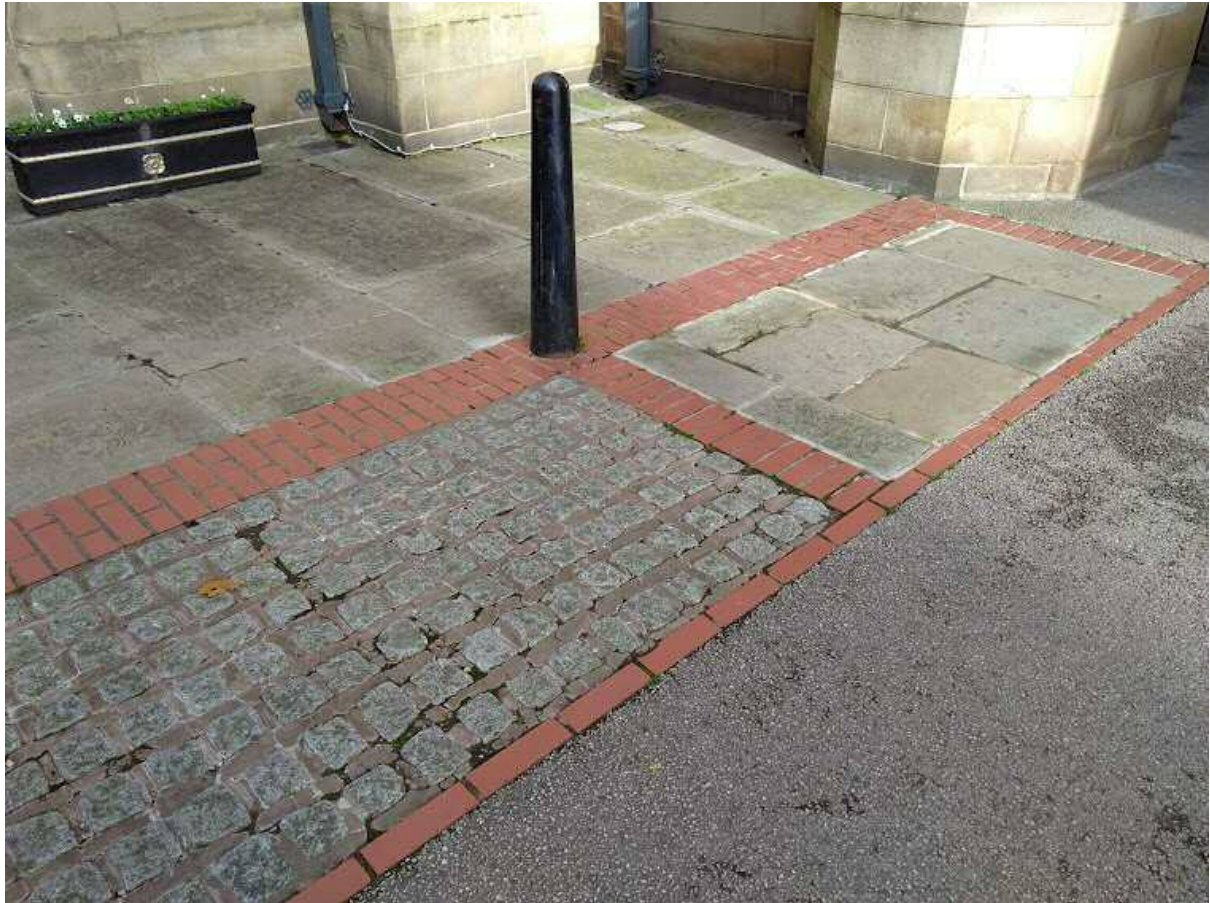
Fig 3: Example of Granite Setts and red bricks in the Old Quad – design to be replicated in front of Christie Building.
