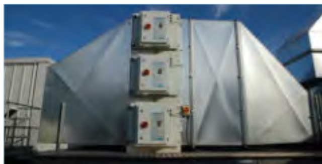
3 ESP Units Stacked in modular formation
