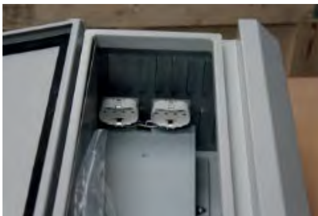
Figure 34 - UV-O 500 UV Lamp Plugs
