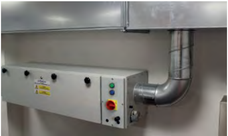
Figure 6 - UV-O 1000 Unit Installed
